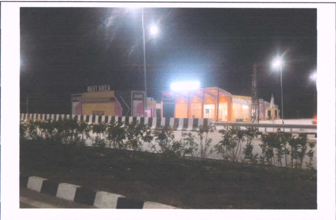
Km. 15+400 (Rest Area) Photographs of Rest Area RHS
