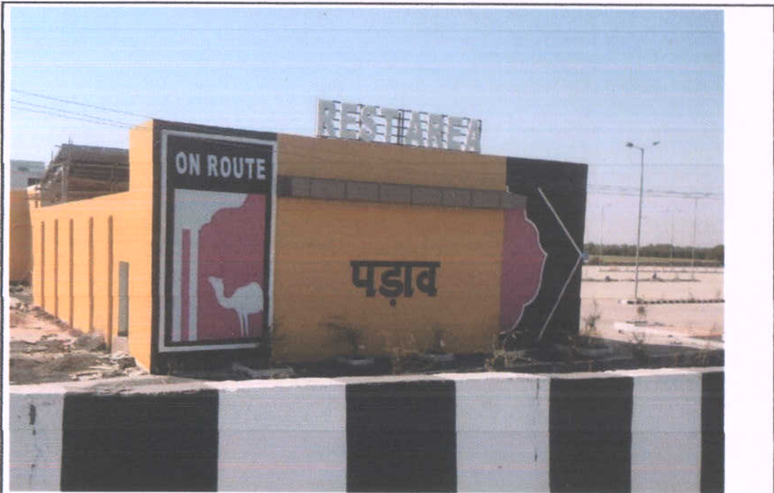
Km. 15+400 (Rest Area) Photographs of Shop Block RHS
