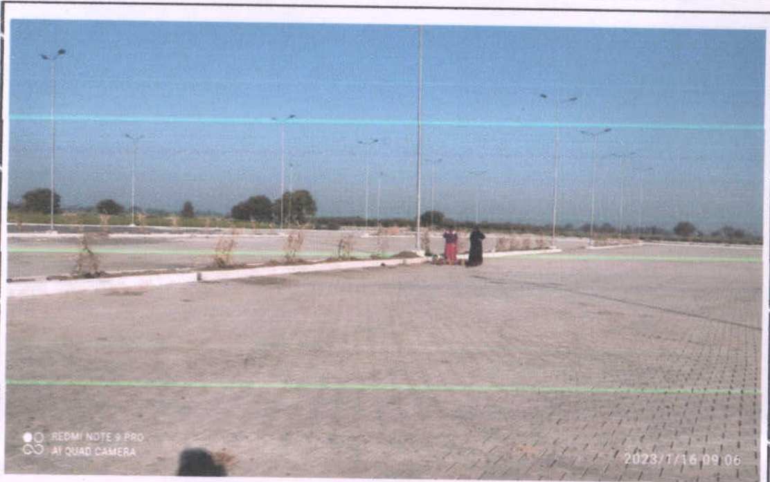
Km. 15+400 (Rest Area) Photographs of Parking area of Rest Area RHS
