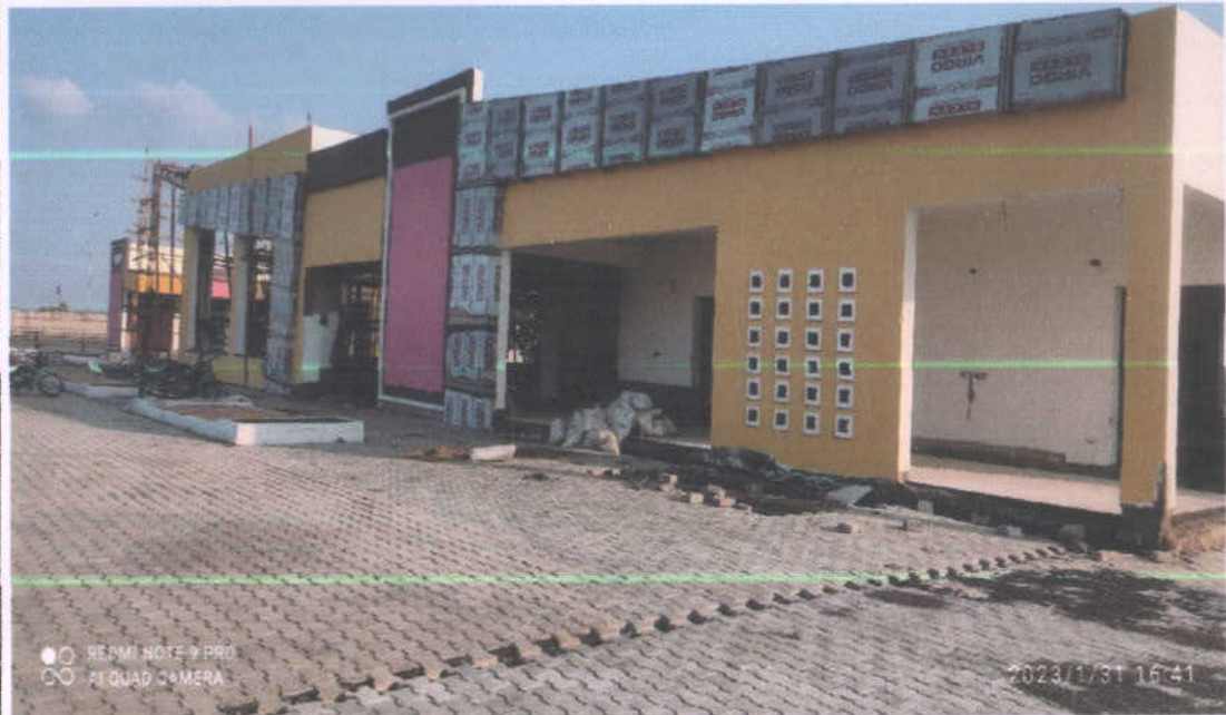
Km. 15+400 (Rest Area) Photographs of Visitor Block & Restaurant Block RHS
