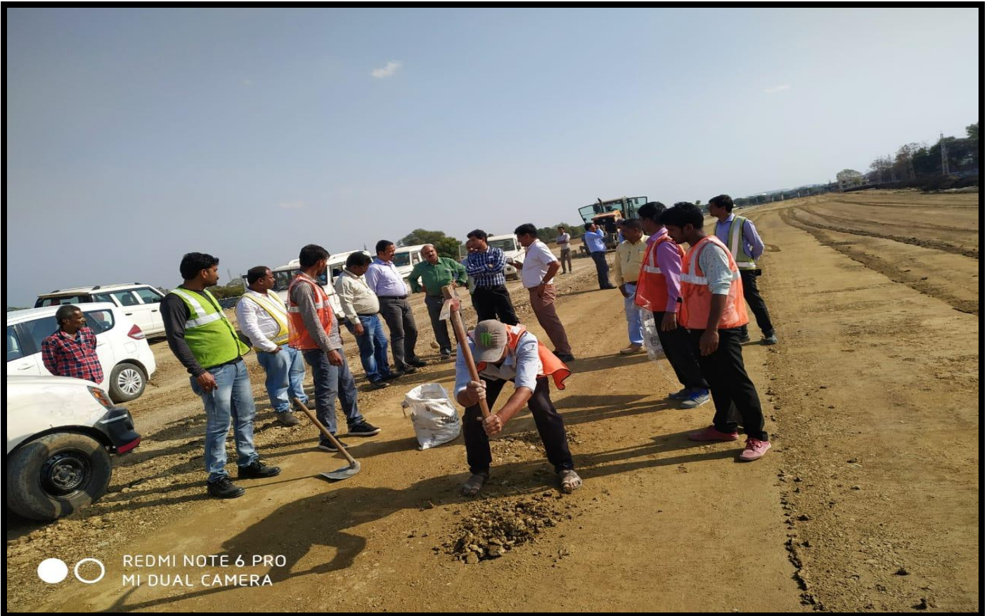
Lenders Engineer & Team Leader Testing of Subgrade Top @ Ch. 15+250 (RHS)
