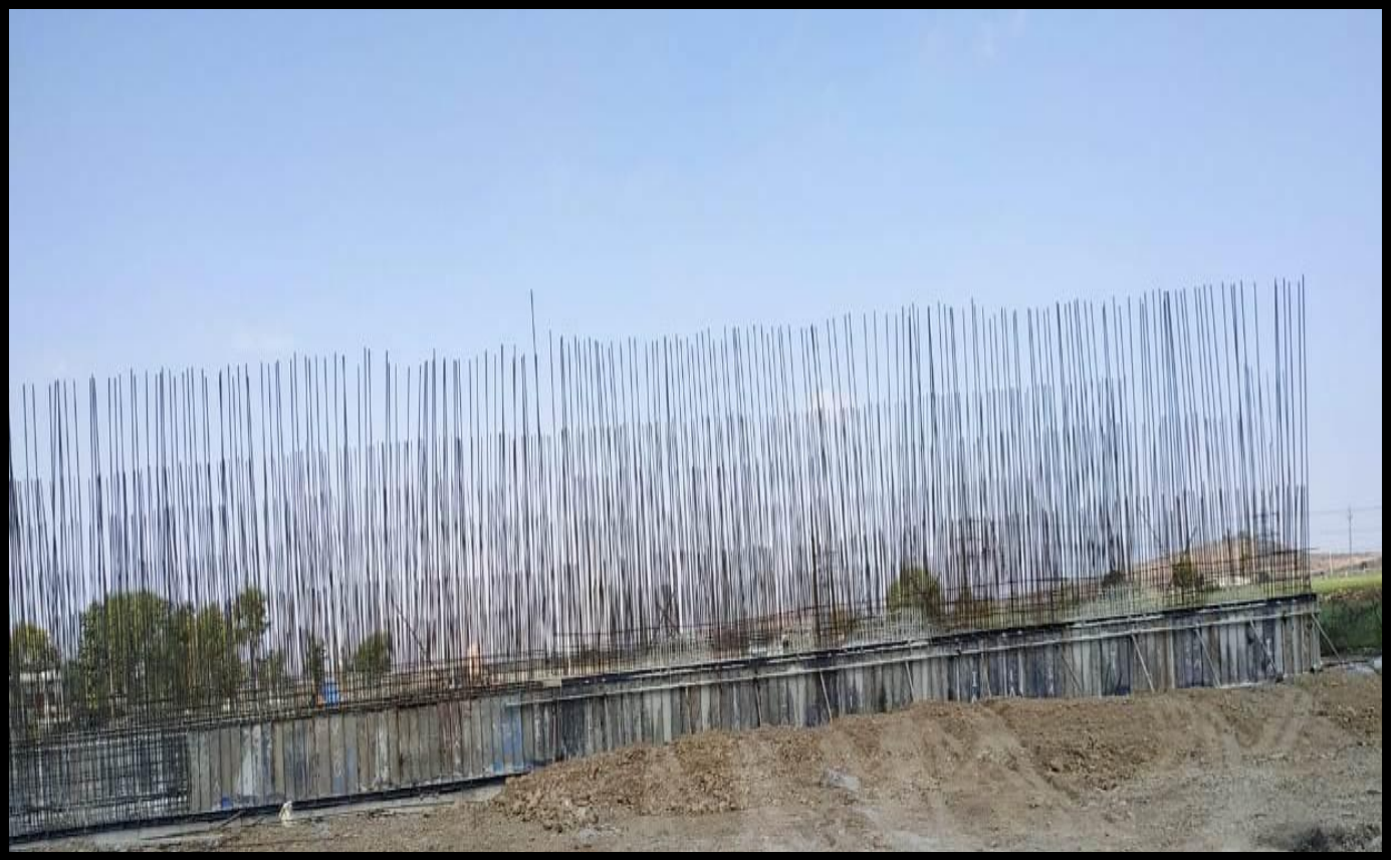
Minor Bridge @ Ch. 44+800
