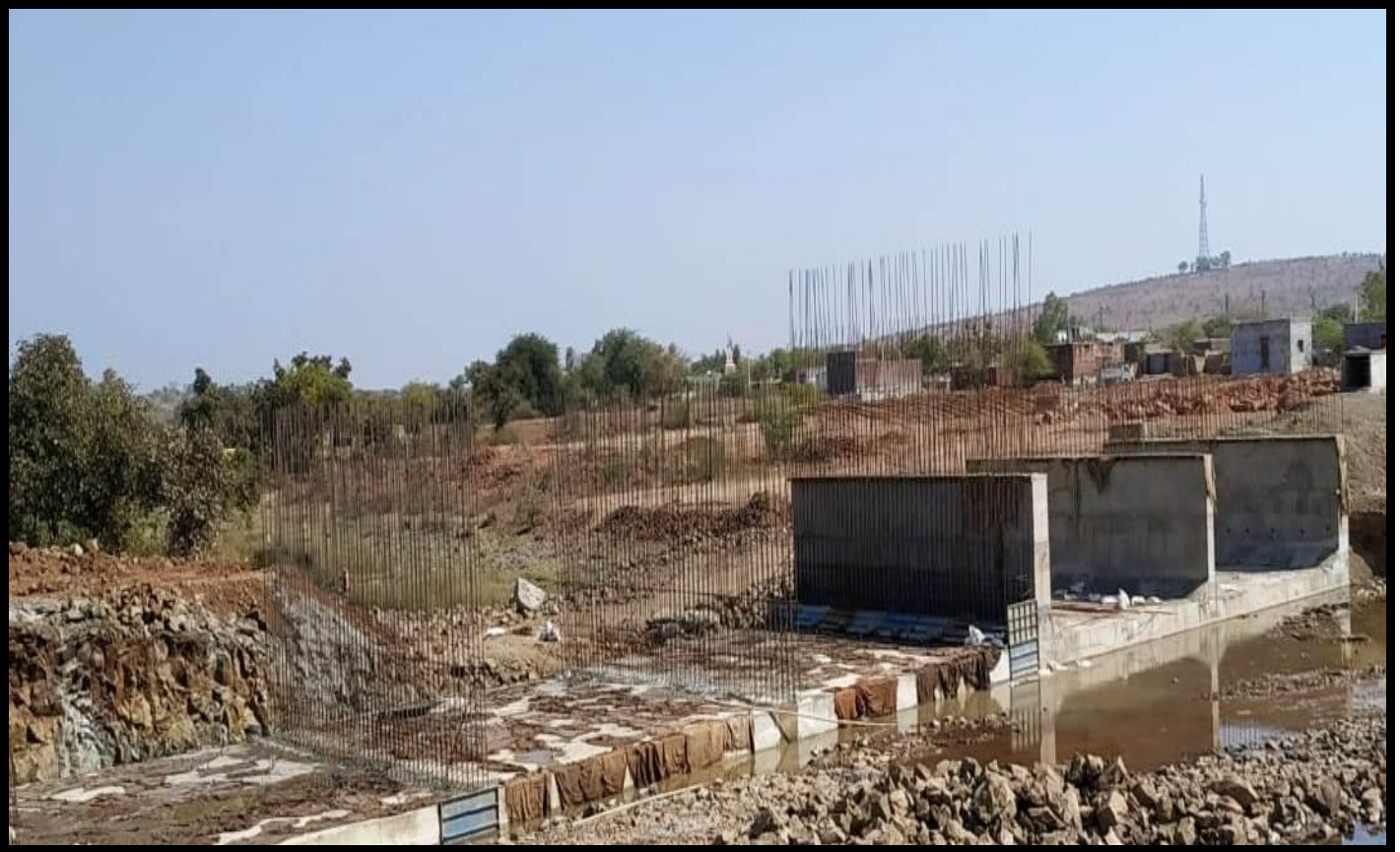
Minor Bridge @ Ch. 49+785
