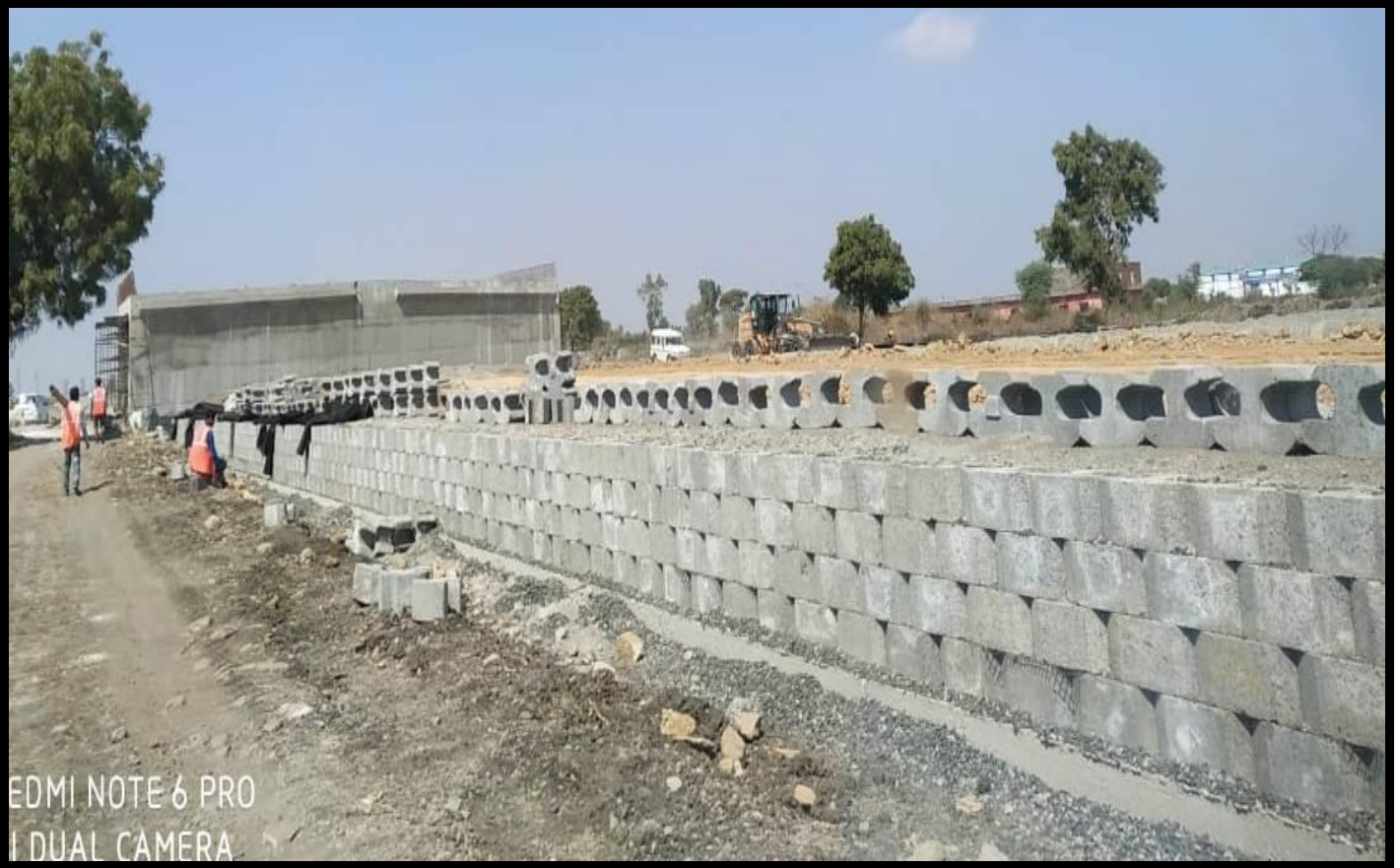
RE Wall Block Erection @ Ch 41+465
