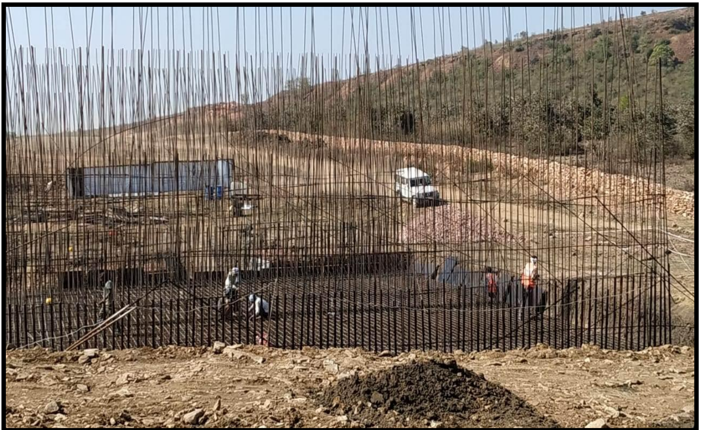
Checking of Raft Steel & Shuttering @ Ch. 54+075
