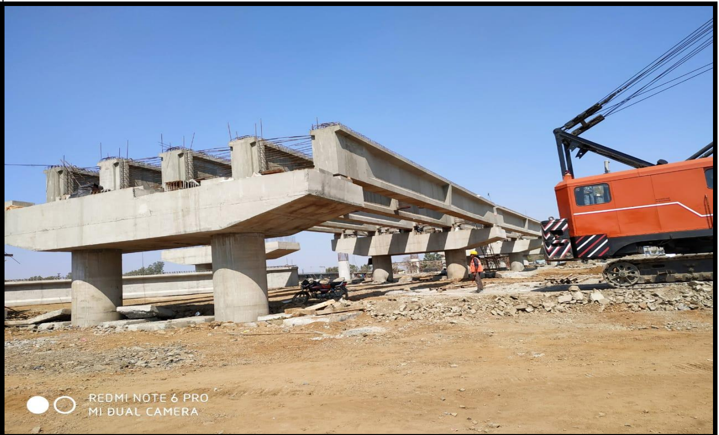
Girder Launching at Elevated Highway @ Ch 47+830
