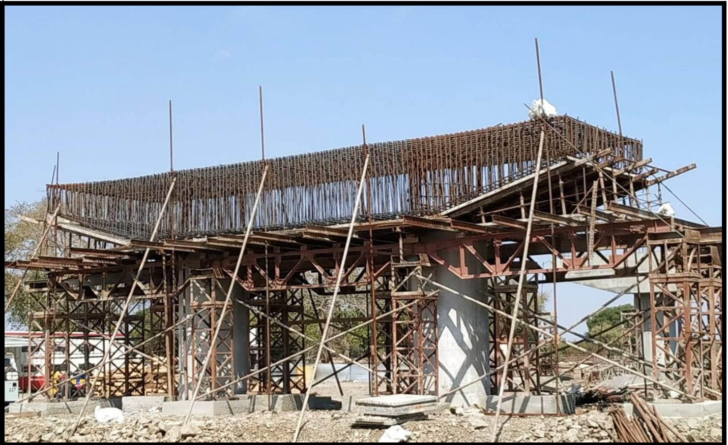
Checking of Girders Casting by Landers Engineers @ Ch 47+830
