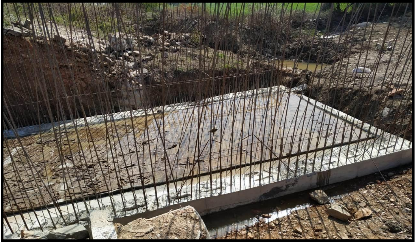
Raft of Box Culvert @ Ch. 55+820
