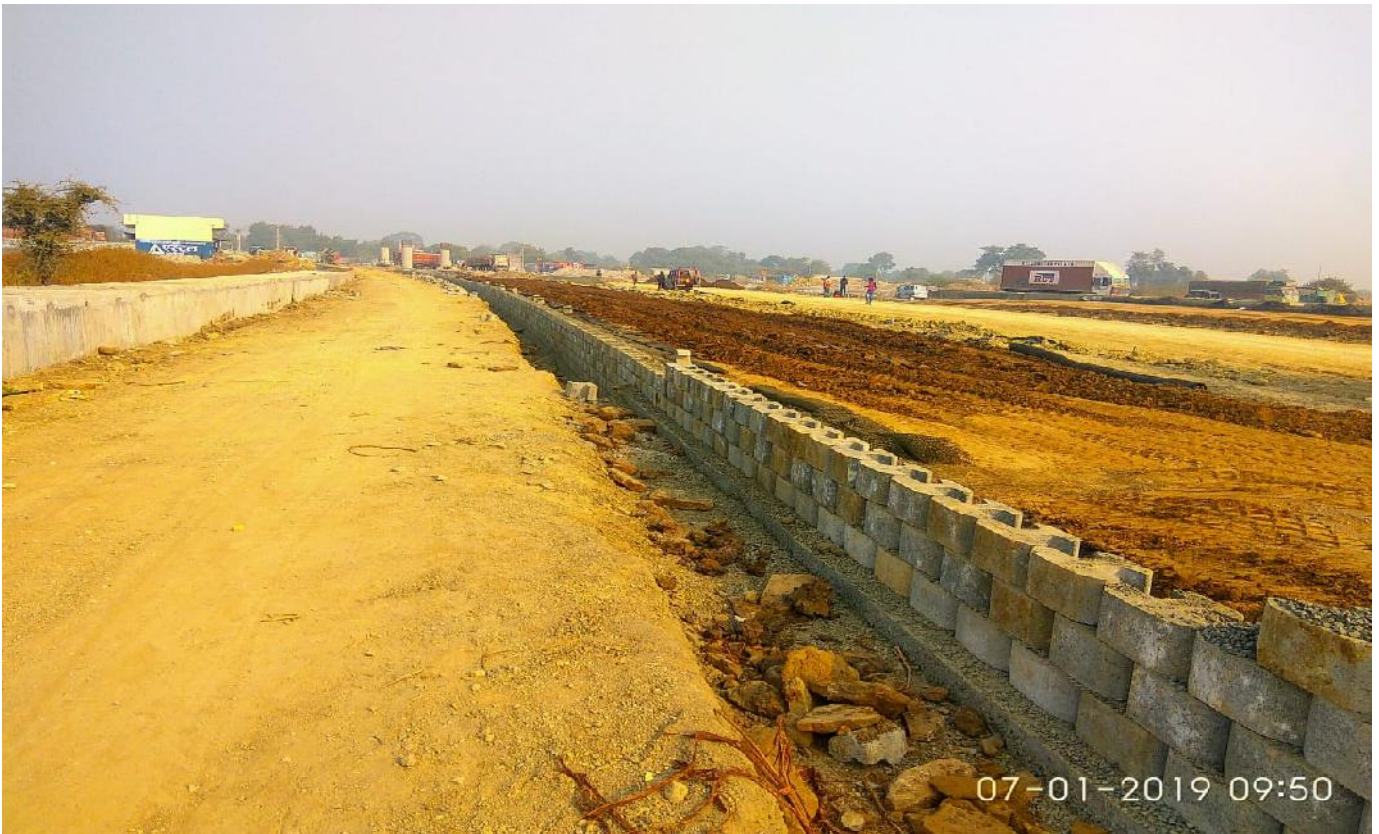
RE Block Erection at at Ch.27+029(VUP)
