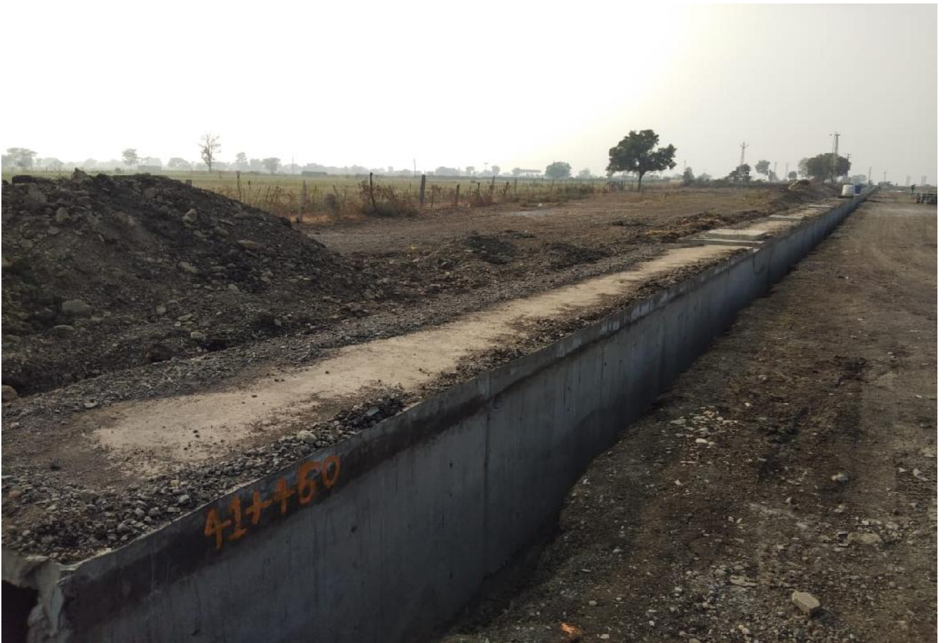
Drain Slab at Ch.41+400 to 41+460
