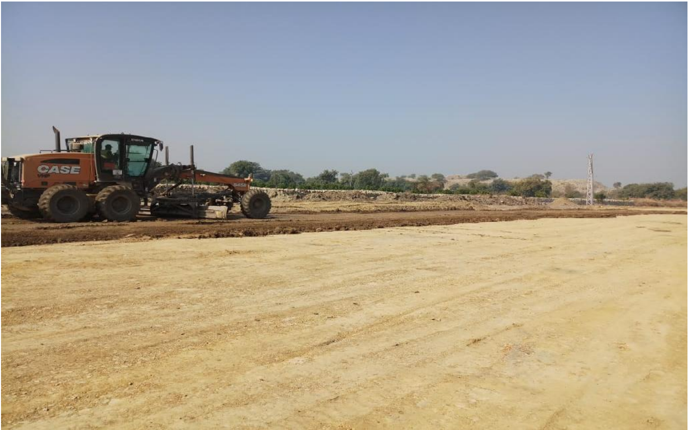
Embankment Layer at Ch.56+480 to 56+900
