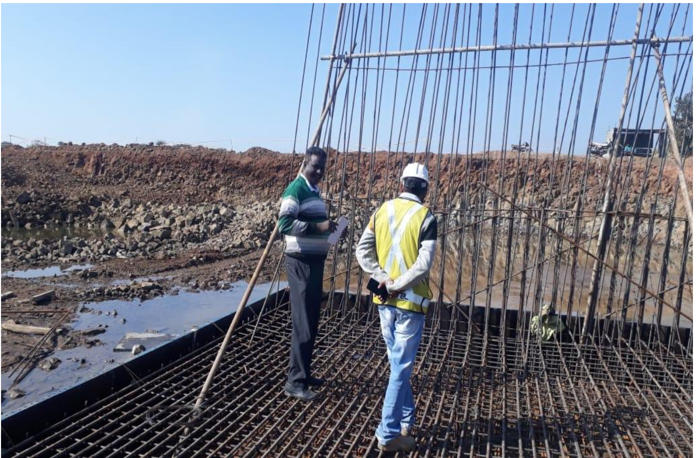
MNB Raft Service Road at Ch.49+785
