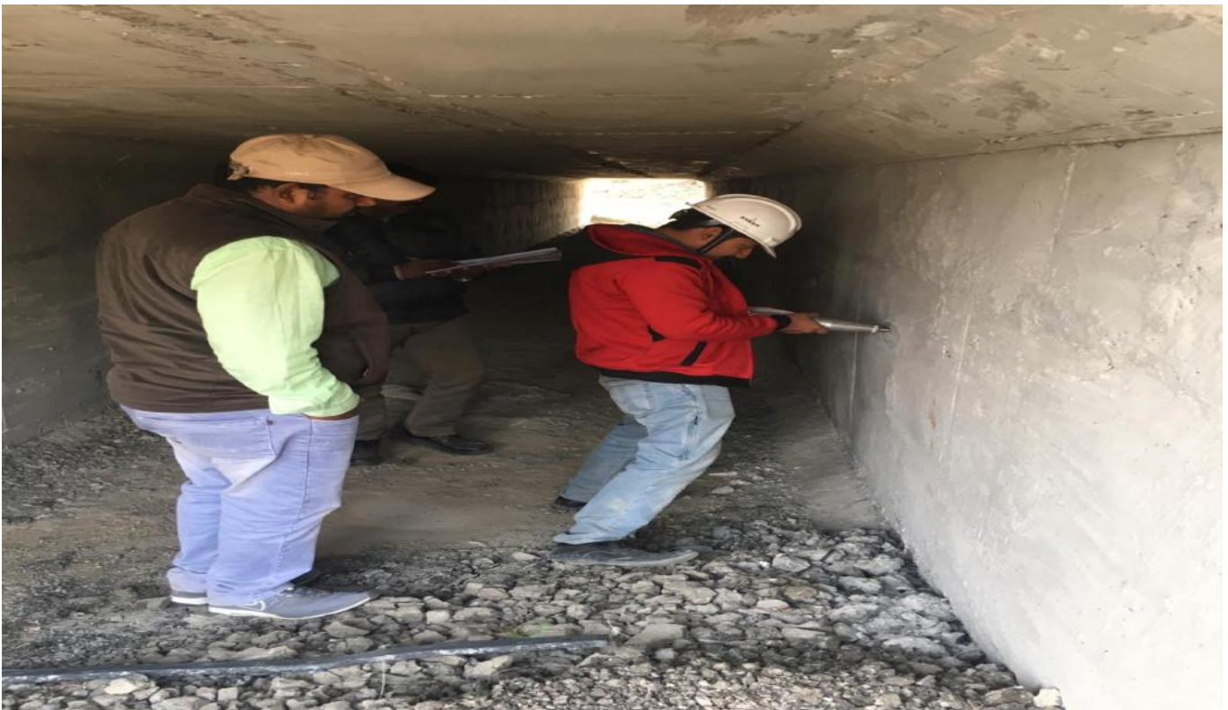
Rebound Hammer Test at Box Culvert
