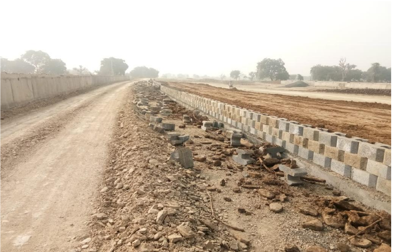
RE Block Erection at at Ch.25+100 (VUP)
