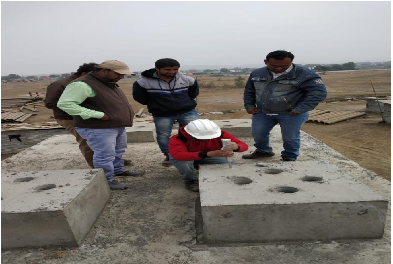
Rebound Hammer test at Ch.47+830 Elevated Highway
