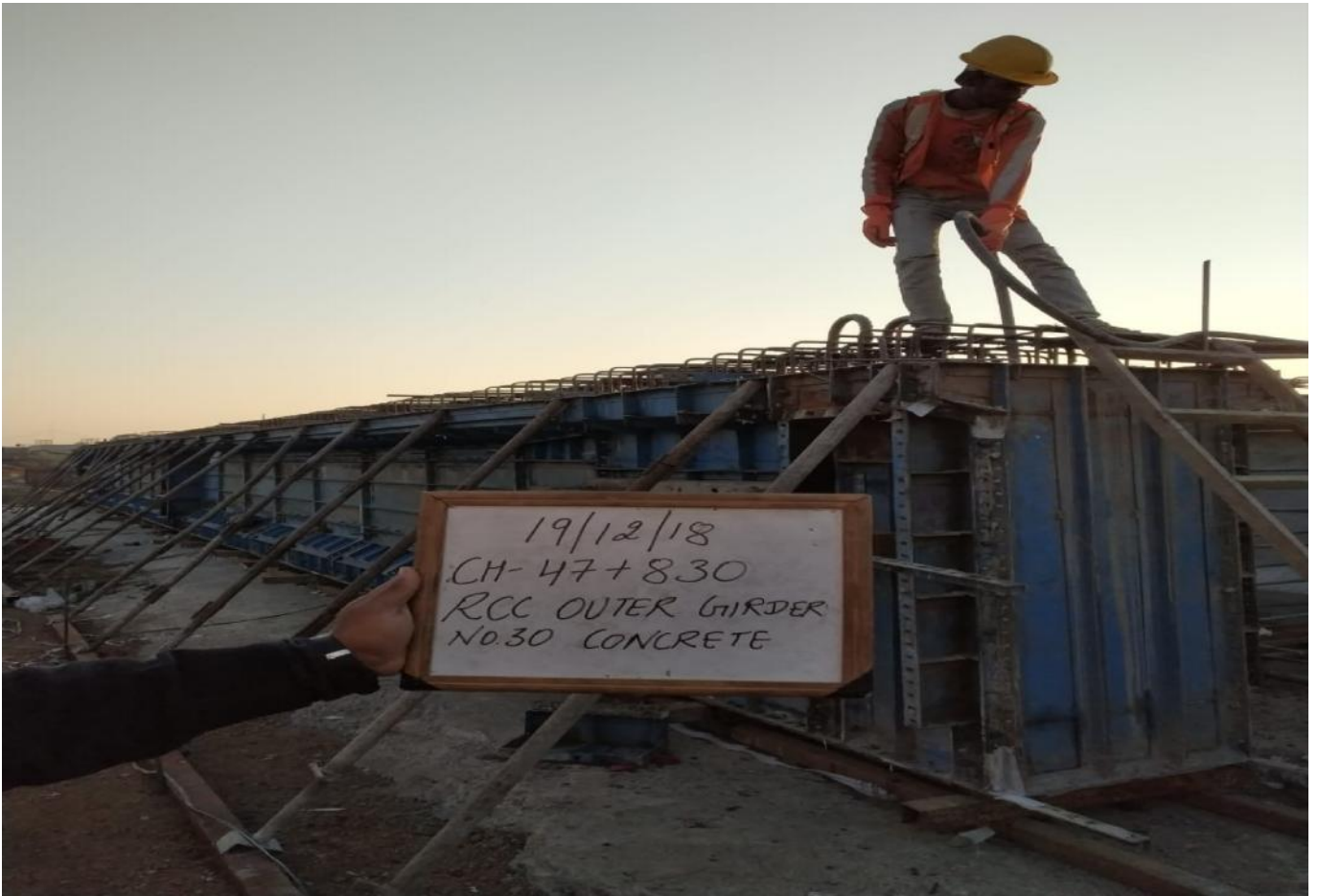
Girder Casting at Ch.47+830(Elevated Highway)
