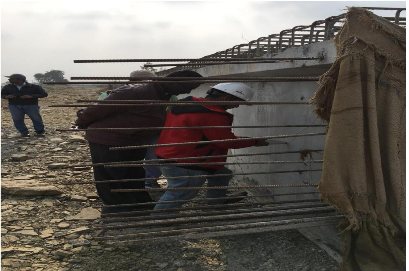
Rebound Hammer Testing of Girder at Ch.36+105 MJB
