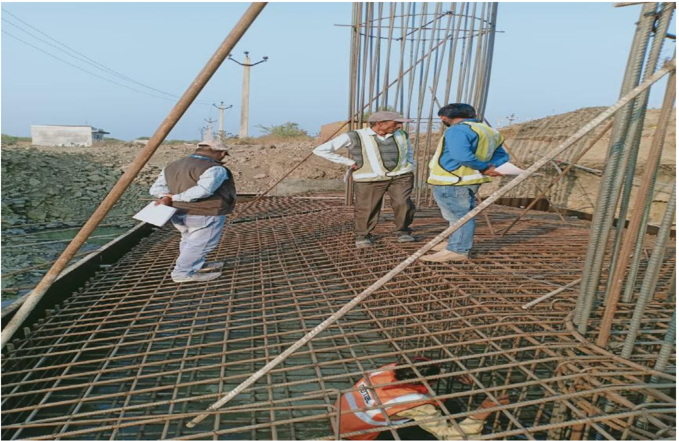
Reinforcement Checking at Ch.49+330 VUP
