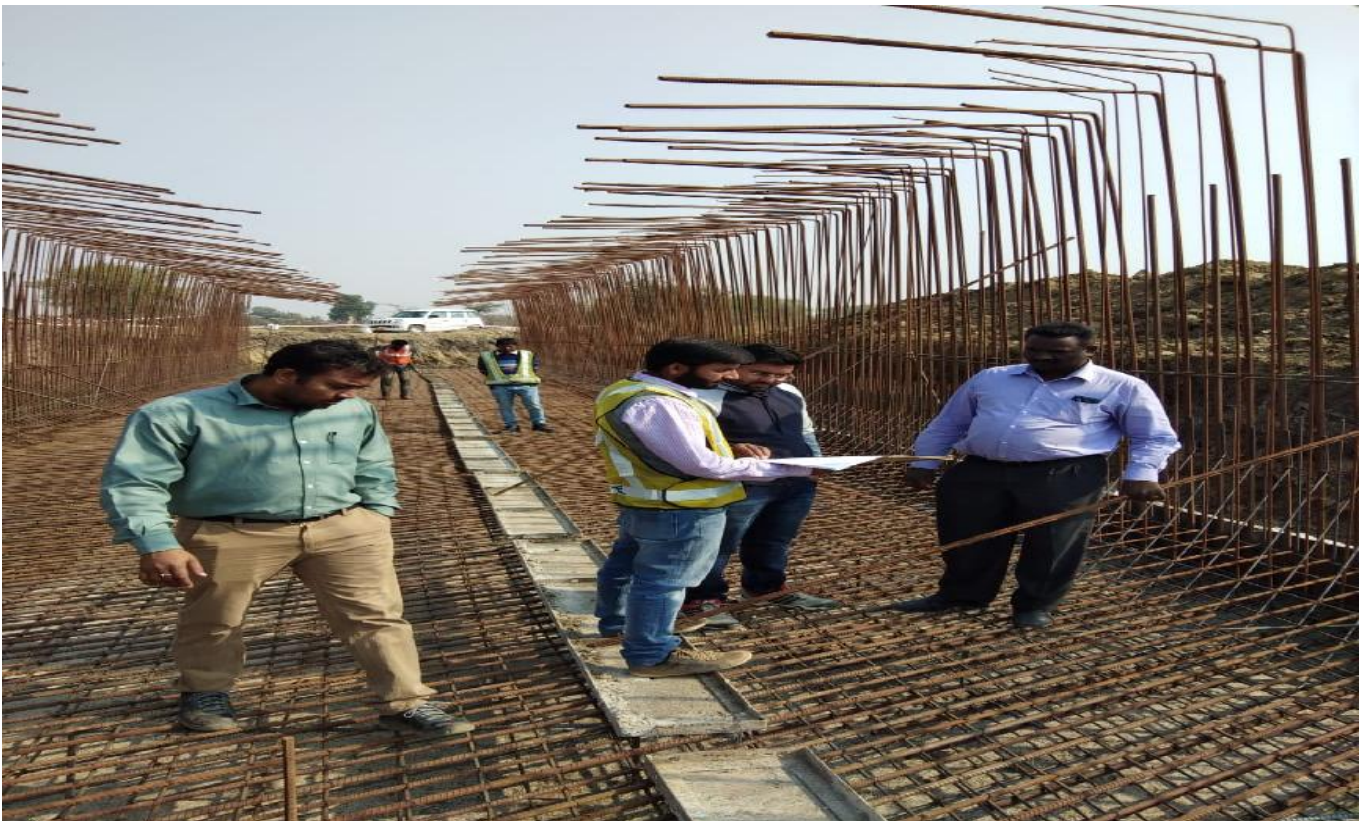
Pier's and Pedestal of Elevated Highway at Mela Ground Ch.47+830
