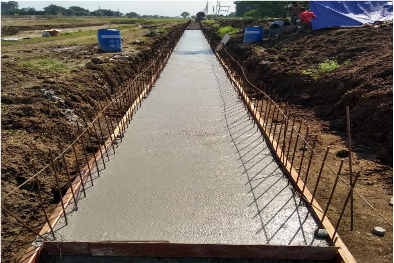
Checking of Drain PCC Thickness at Ch.37+053.
