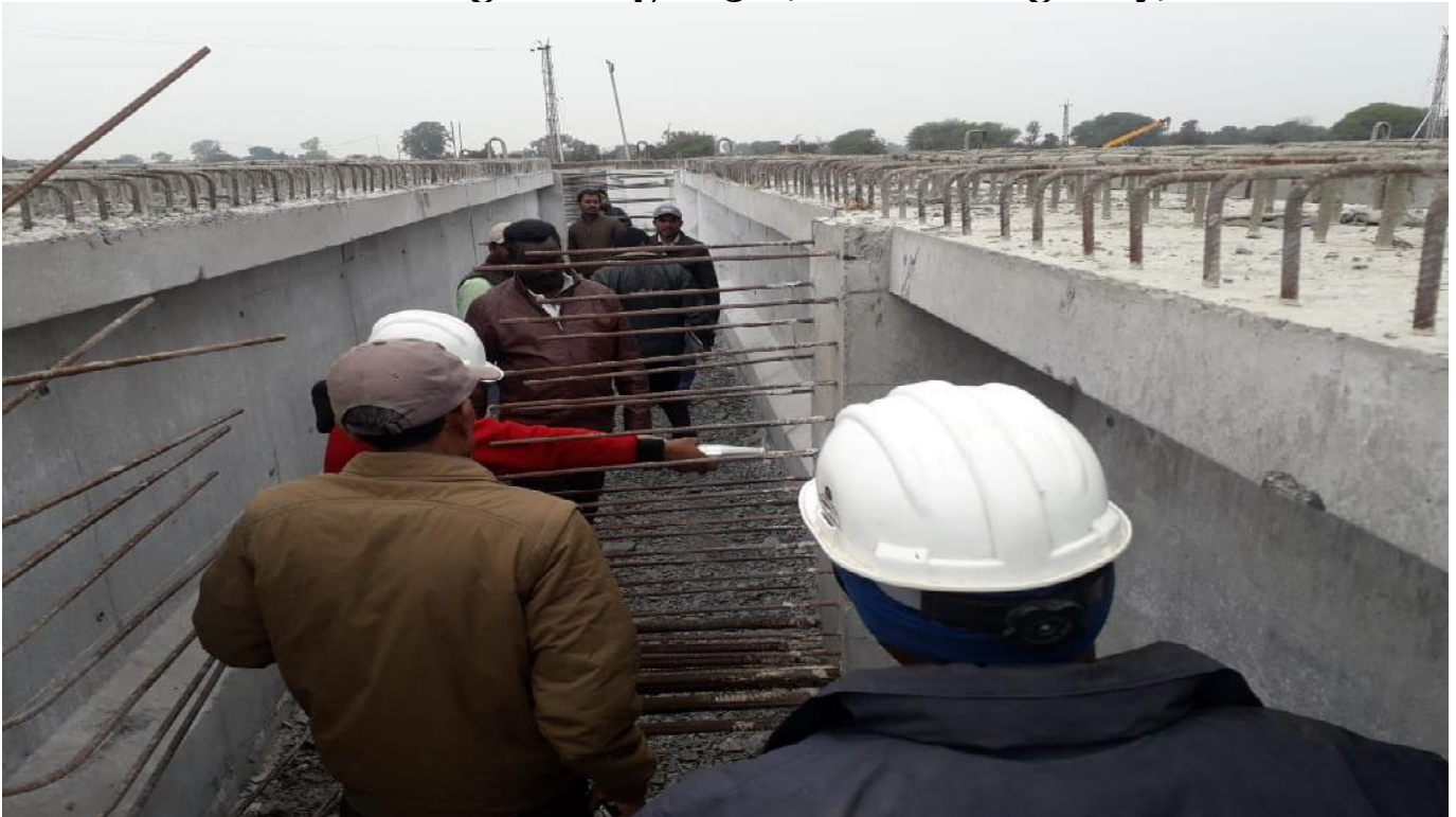
Girder Casting at Ch.47+830(Elevated Highway)
