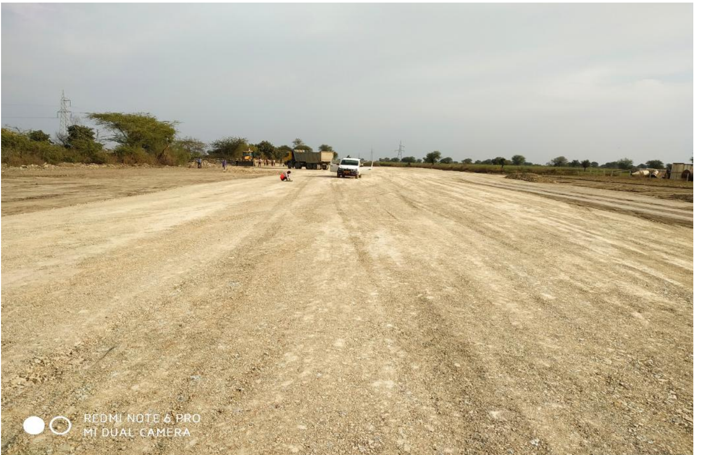
Embankment Layer at Ch.30+200
