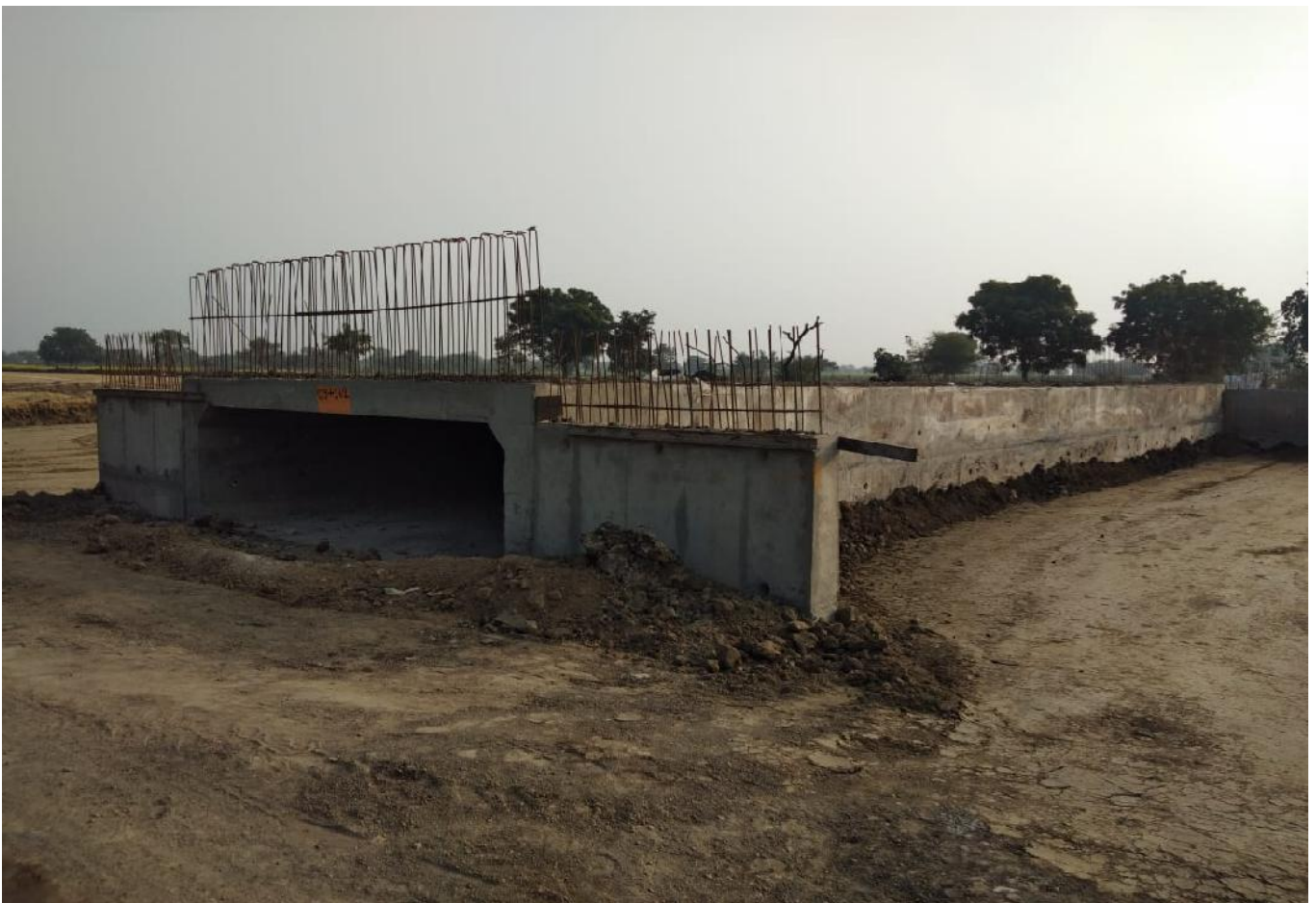
Box Culvert Slab at Ch.39+162
