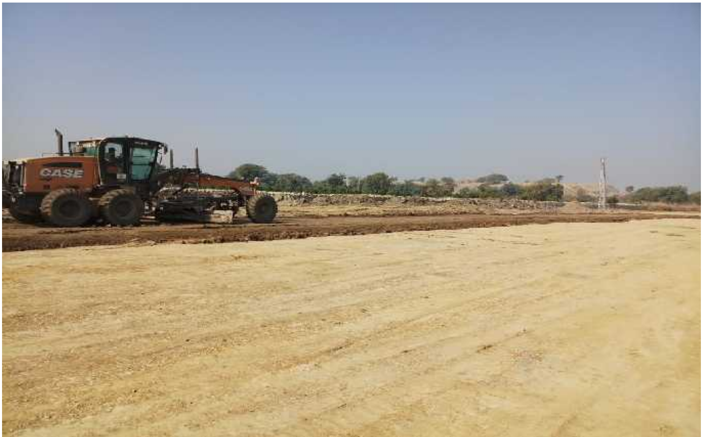
Embankment Layer at Ch.39+165 to 39+200
