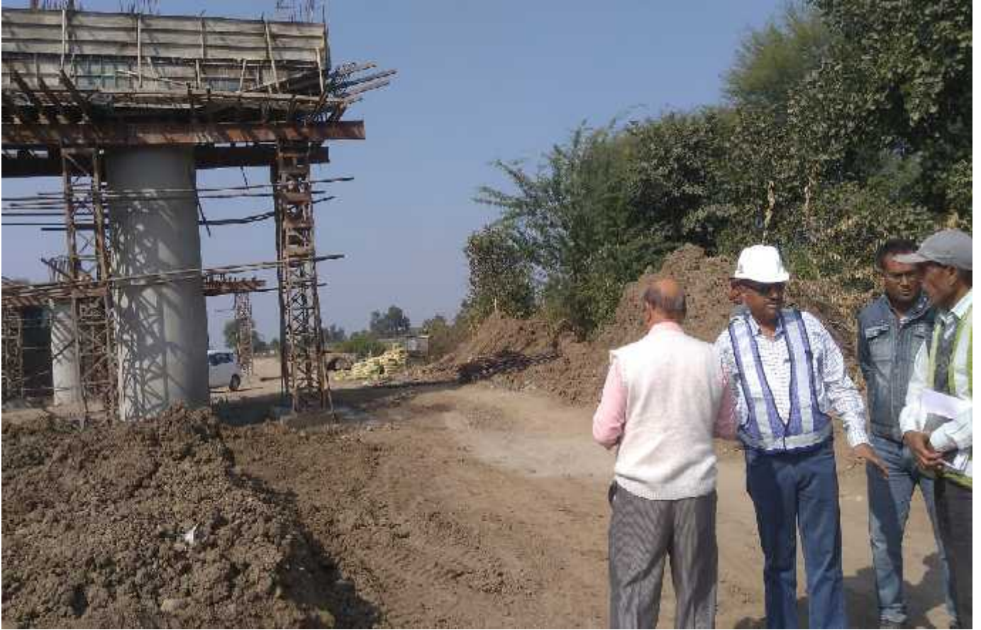
Pier P-9 Lift Checking at Ch.57+127(MJB)
