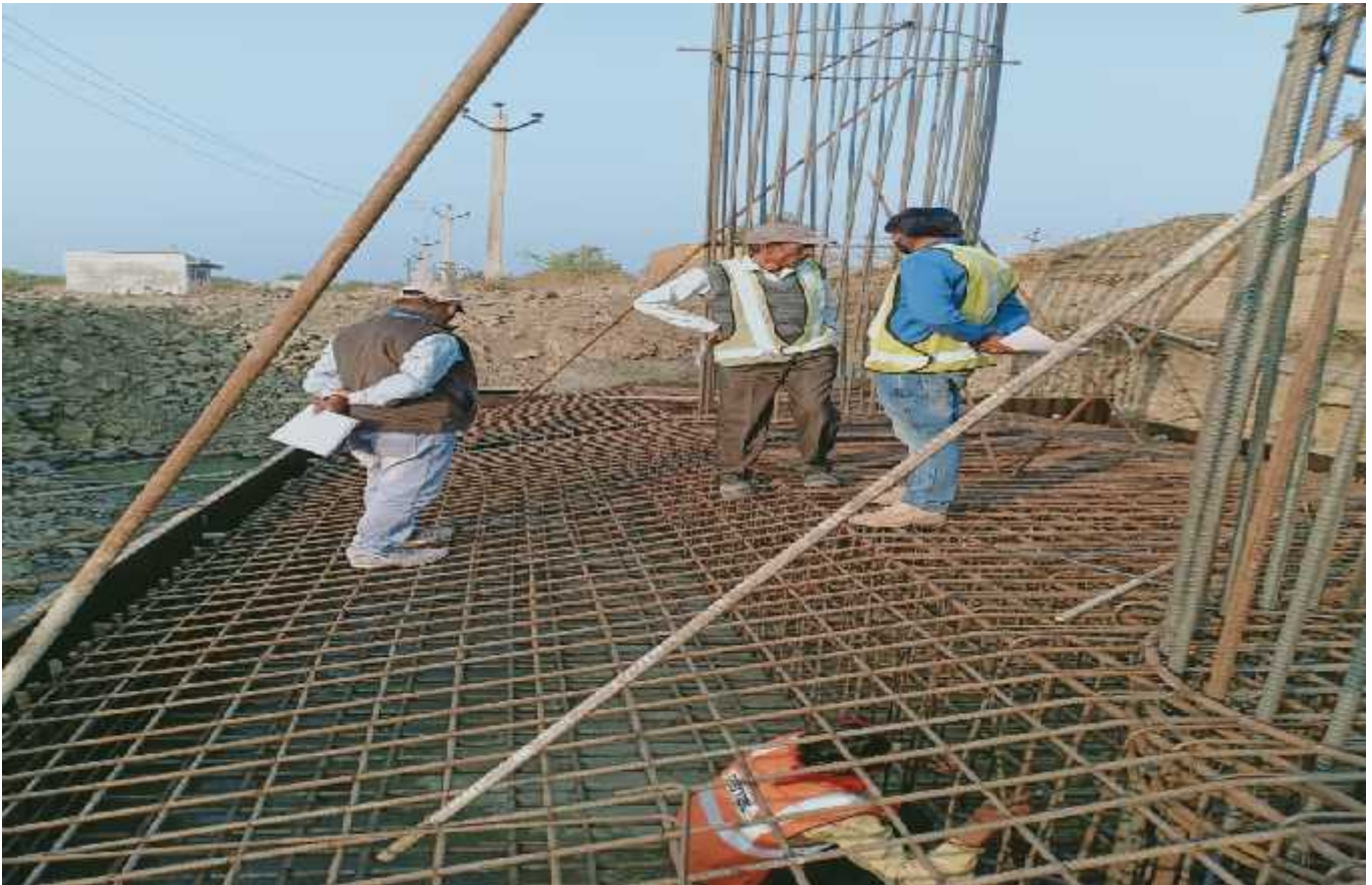
Reinforcement Checking at Ch.49+330 VUP
