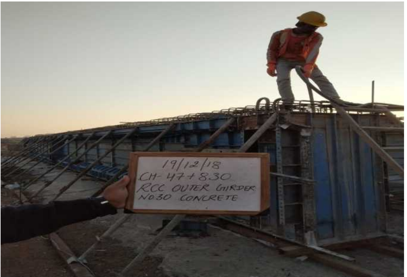
Girder Casting at Ch.47+830(Elevated Highway)
