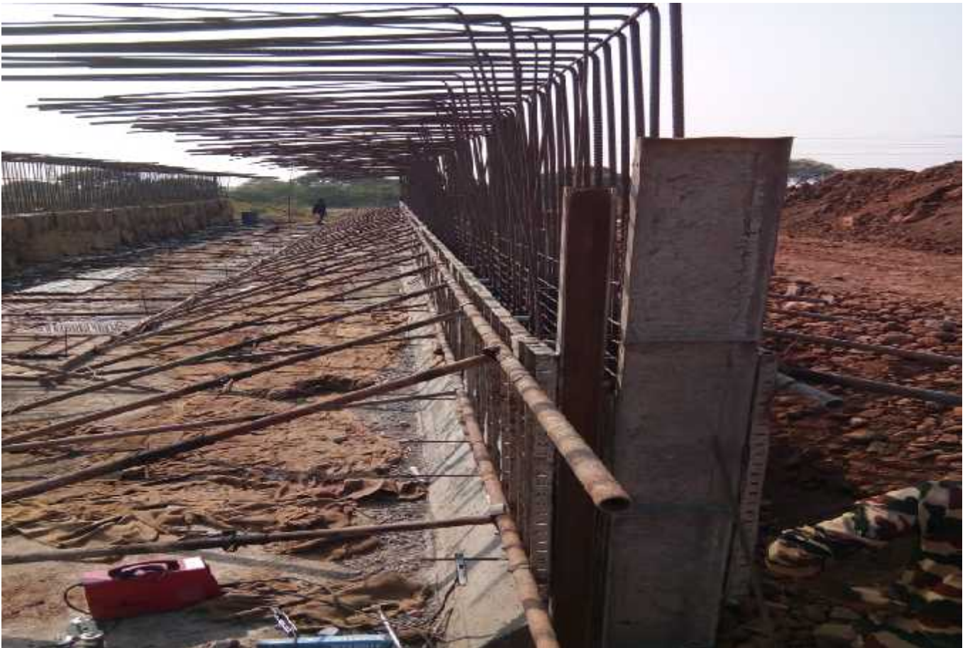
Box Culvert at Ch.53+125
