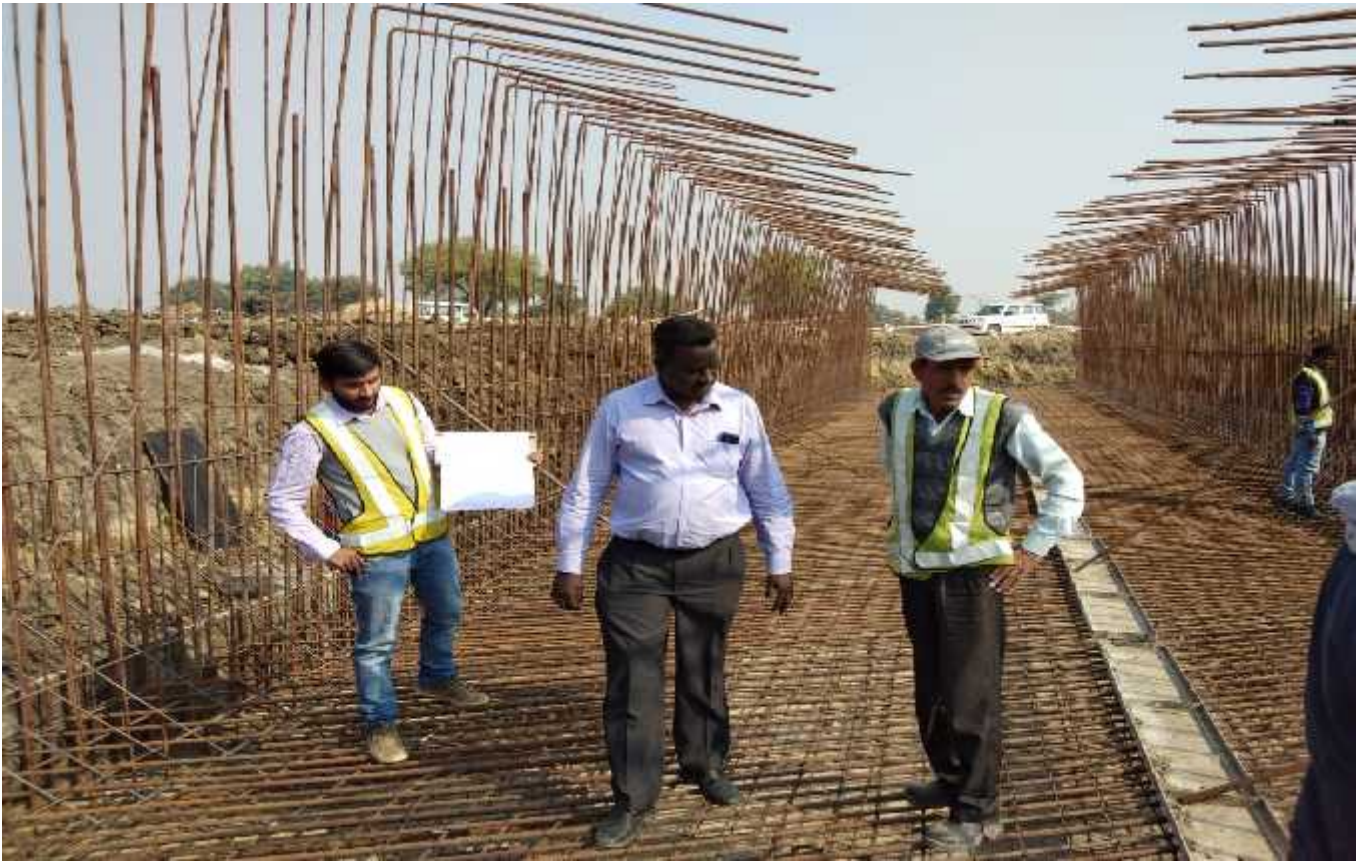
Reinforcement Checking of Box Culvert by RE,LASA at Ch.38+141
