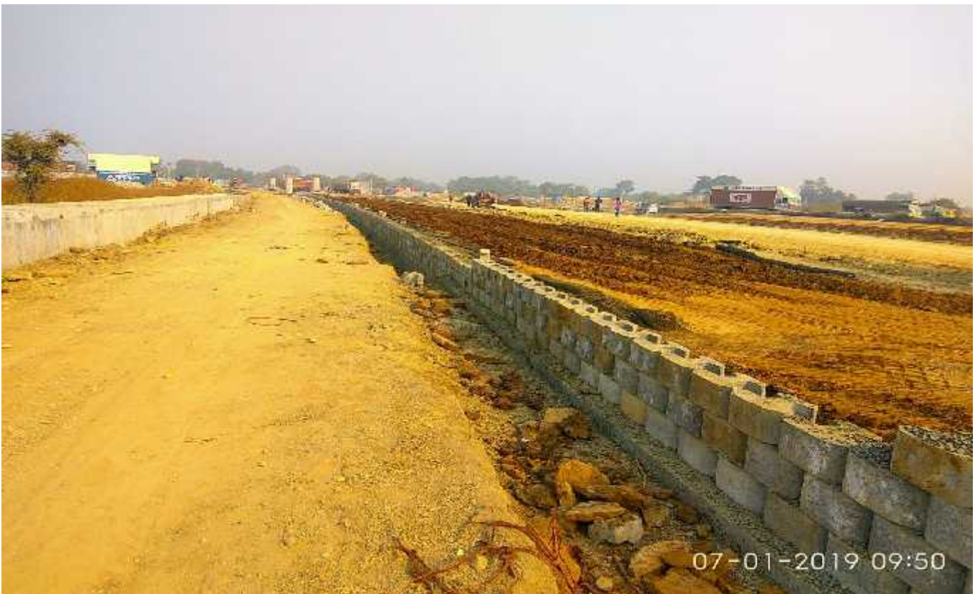
RE Block Erection at at Ch.27+029(VUP)
