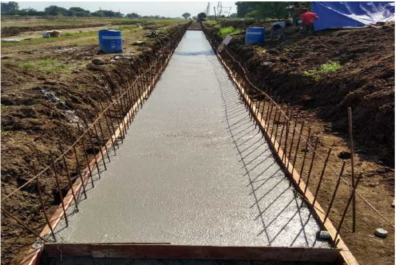
Checking of Drain PCC Thickness at Ch.37+053
