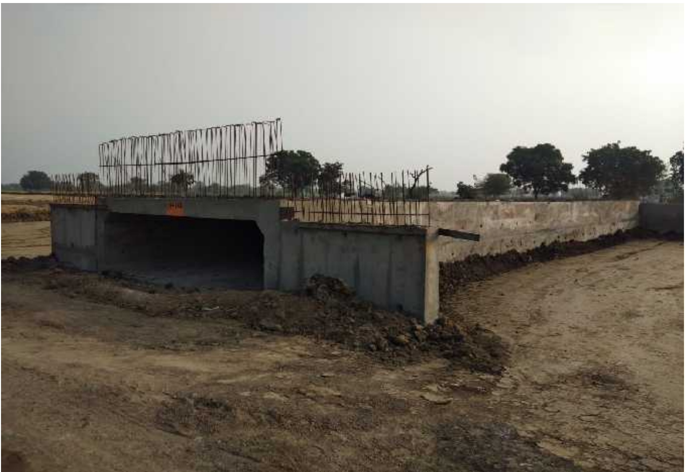
Box Culvert Slab at Ch.39+162
