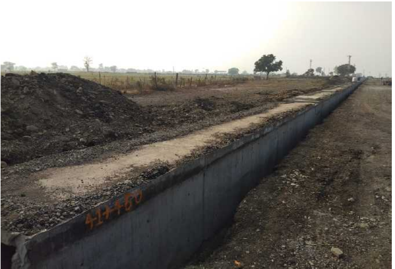
Drain Slab at Ch.41+400 to 41+460
