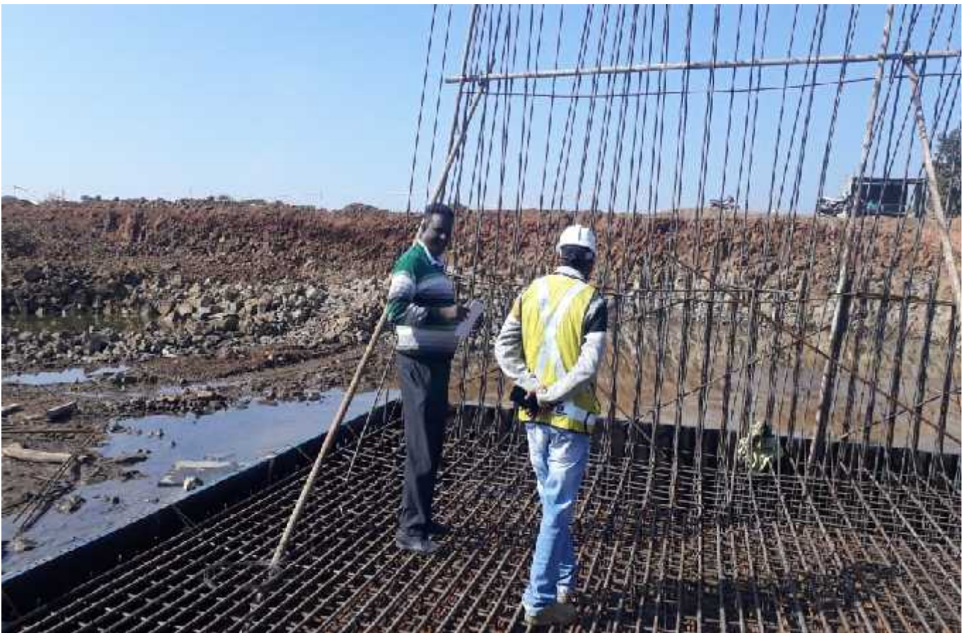
MNB Raft Service Road at Ch.49+785
