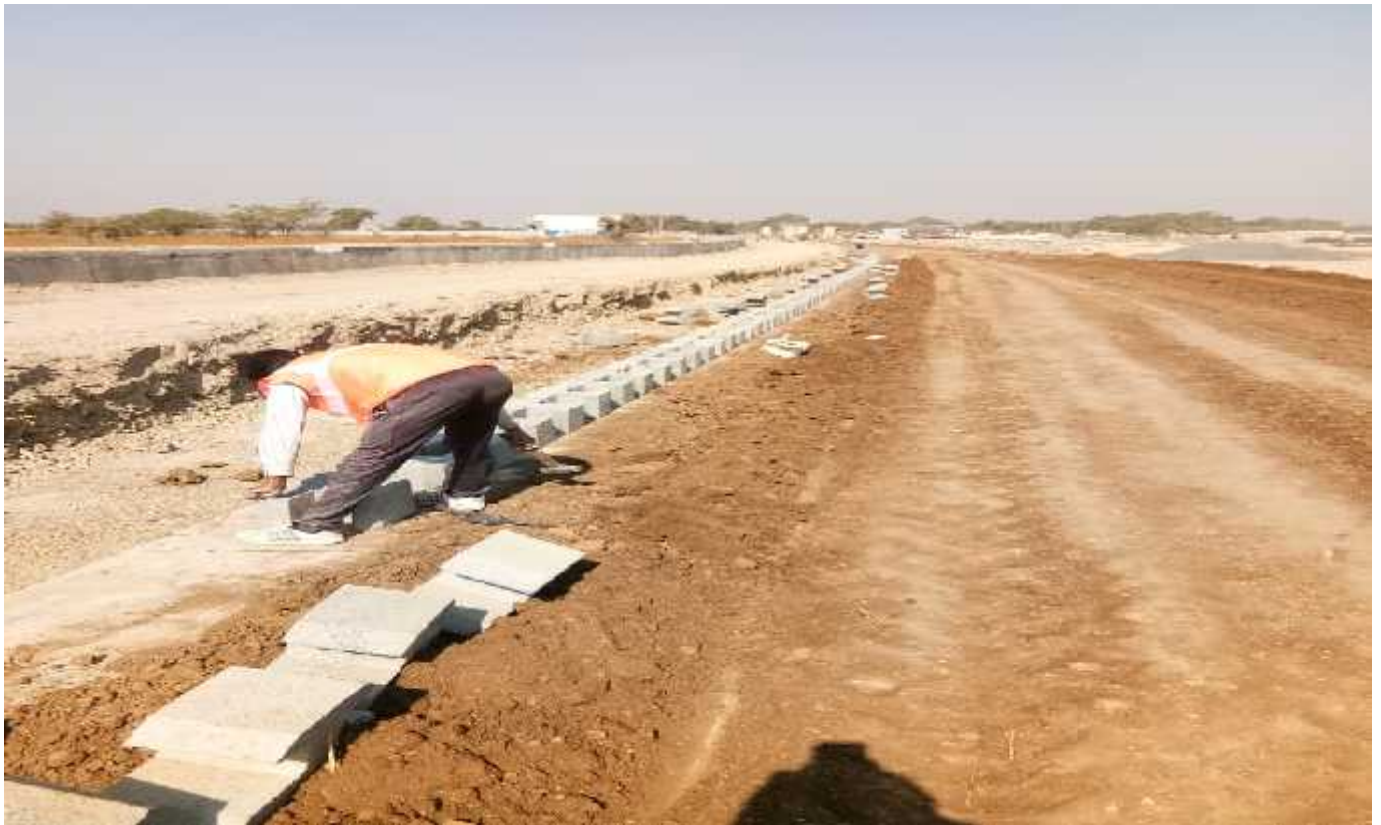
RE Block Erection at at Ch.25+100 (VUP)
