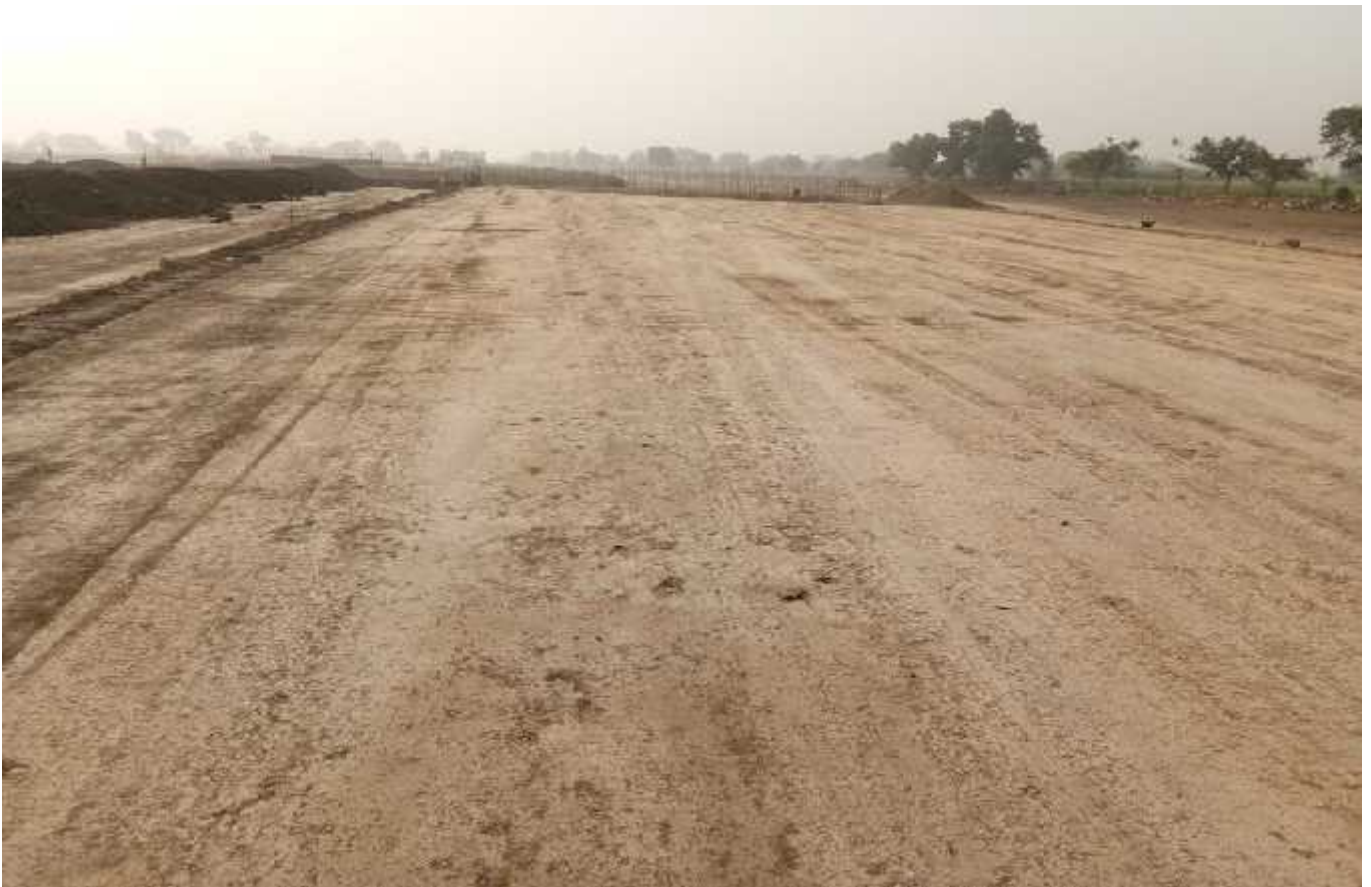
Embankment Layer at Ch.27+380 to Ch.27+580
