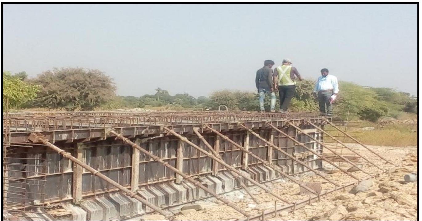
Outer girder steel reinforcement & shuttering checking @CH 27+029
