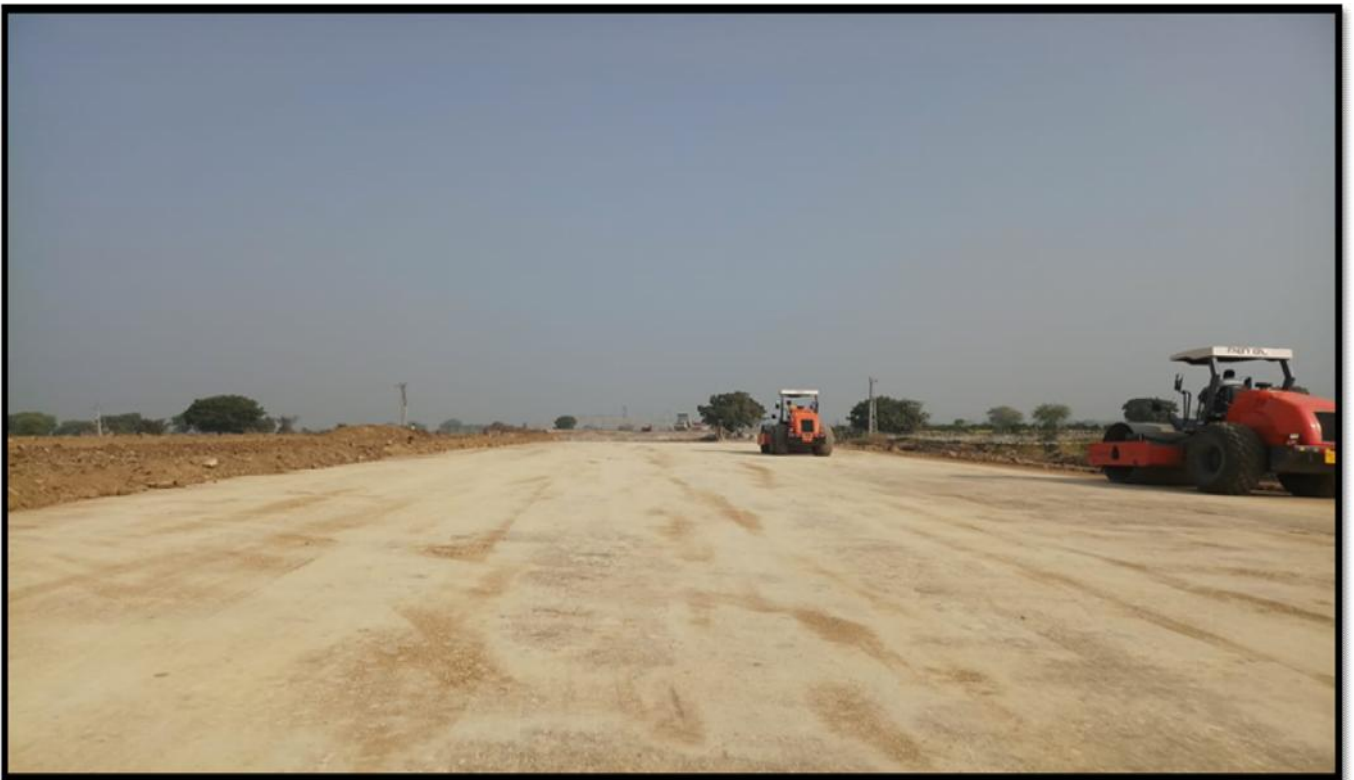
Embankment Layer at Ch.14+000
