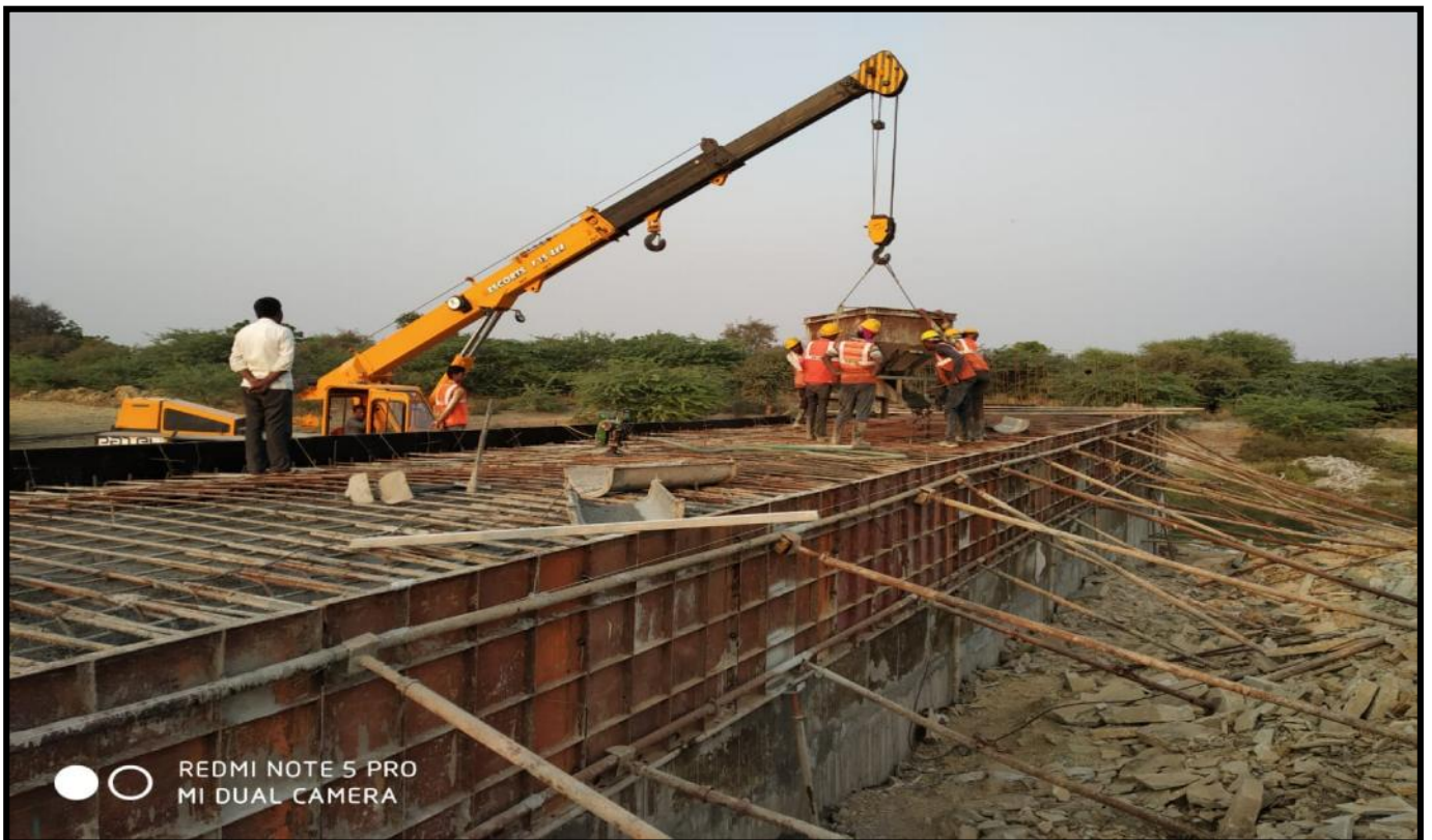
Box-culvert at 22+450 work of slab casting
