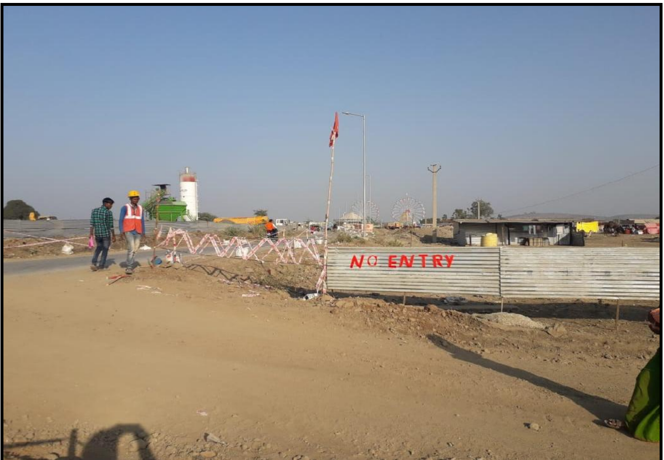
47+830 Mela ground safety maintenance work
