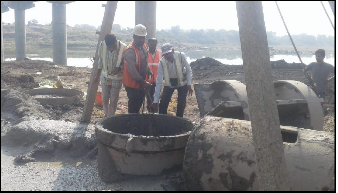
P4/5 bore depth checking at Ch. 57+127
