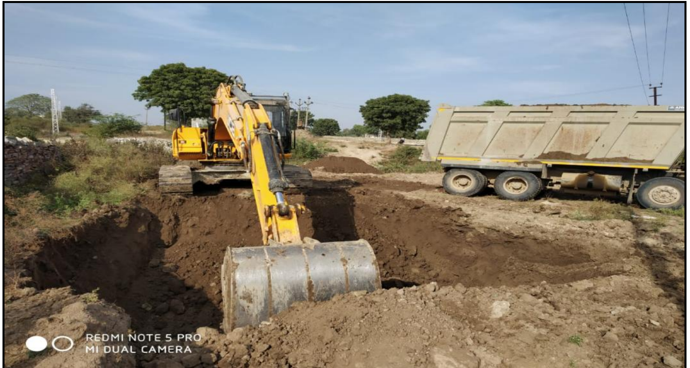
MNB 16+060 RHS Service Road Excavation
