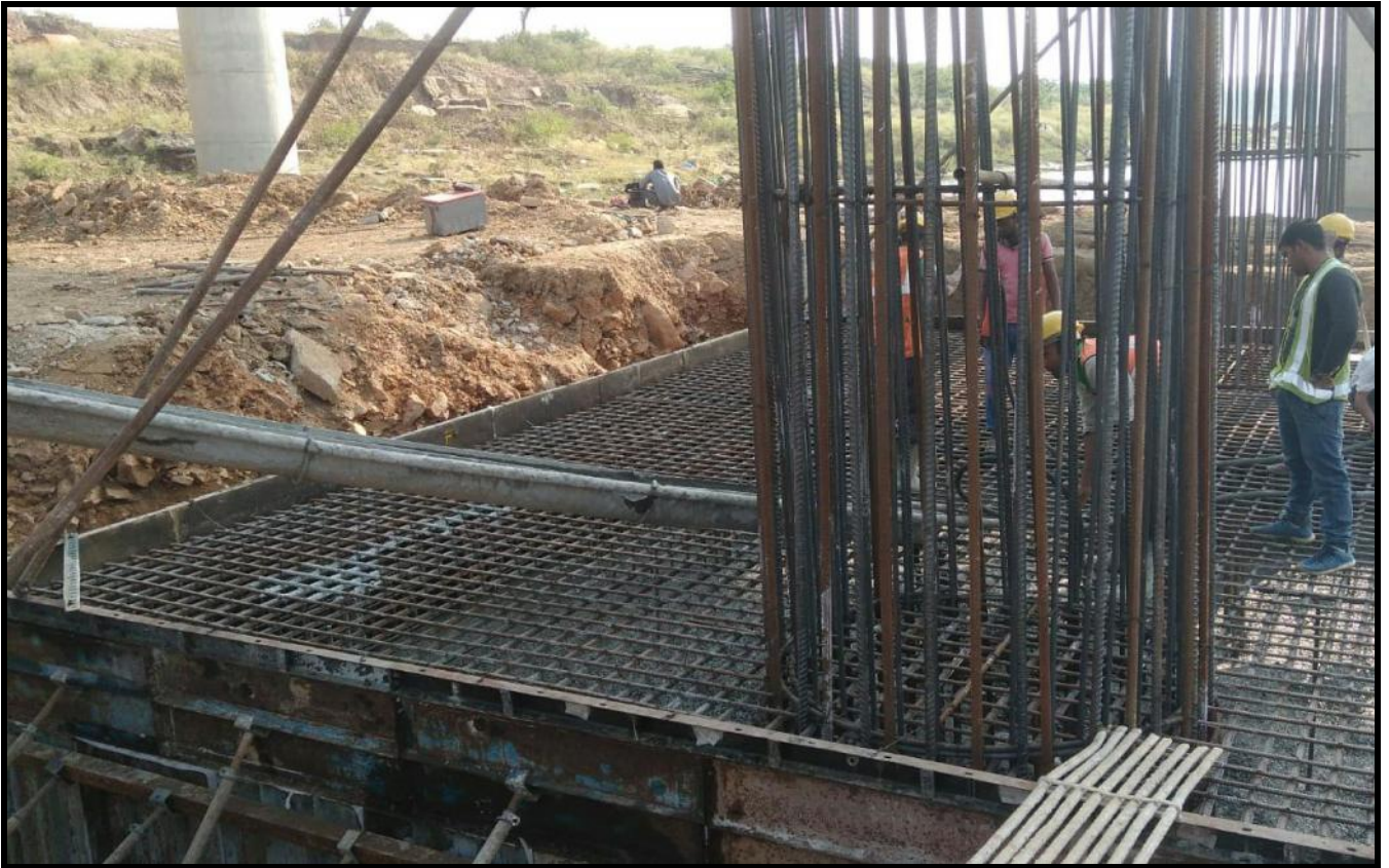
P9 pile cap concreting at Ch 57+127
