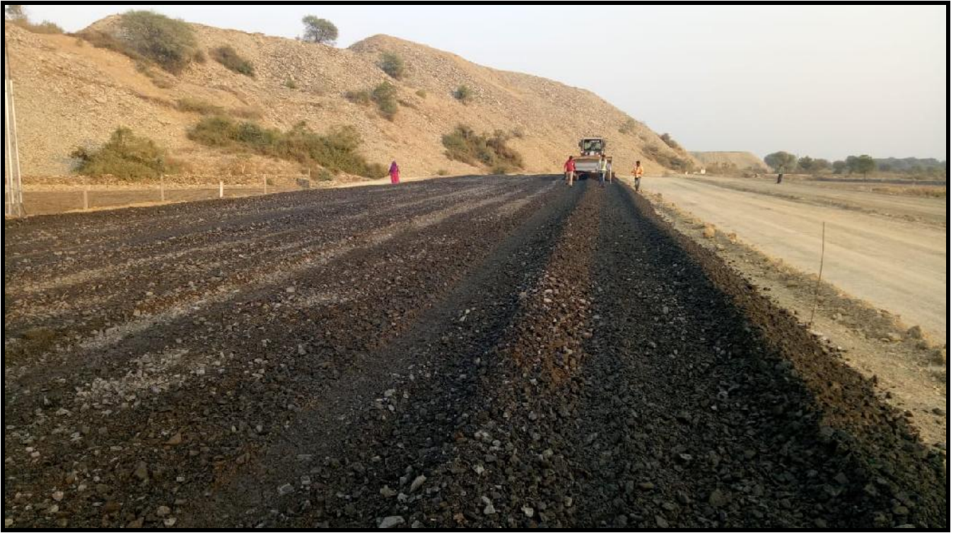
GSB Laying at km 18+600
