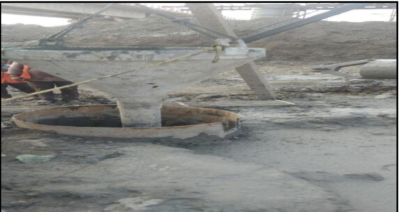
Pile P4/5 concreting at Ch 57+127
