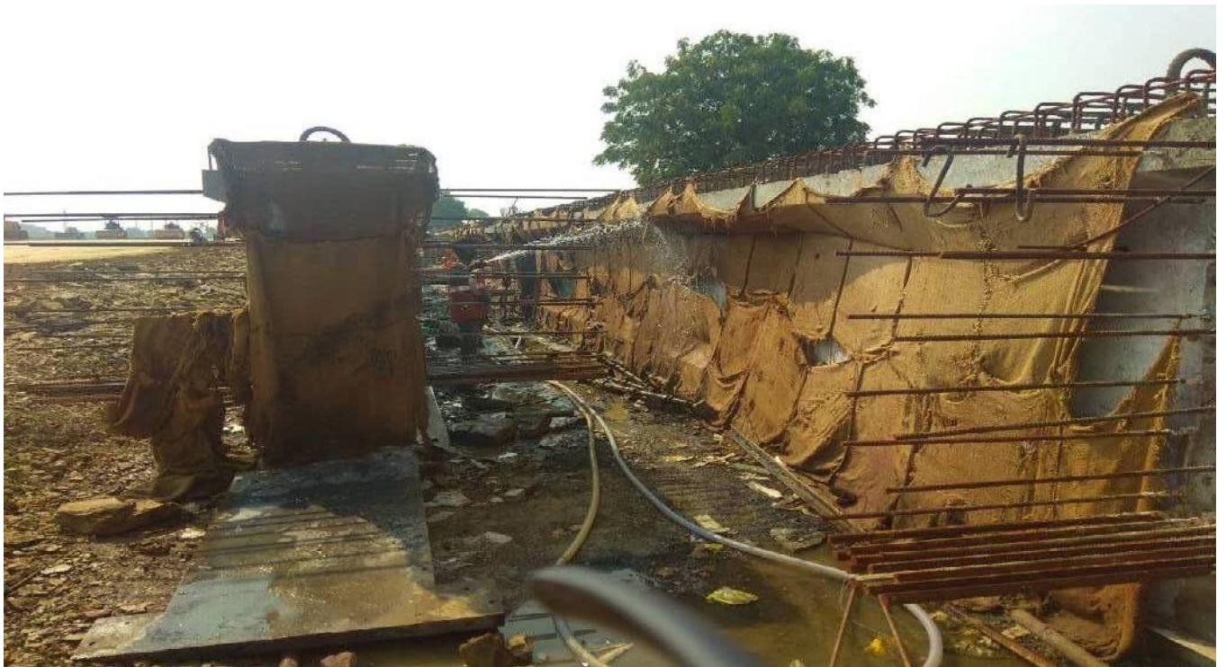
Girder Casting at Ch.27+029
