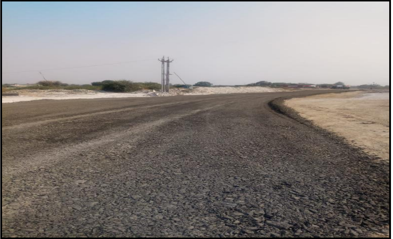
Diversion at CH. 25+000
