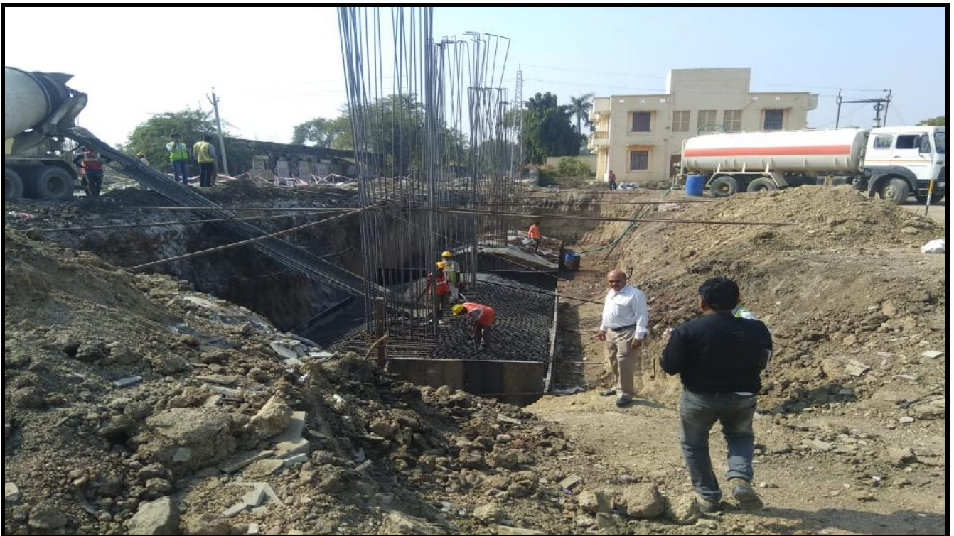
CH 15+725 (LHS) VUP Abutment A1 Raft Concreting
