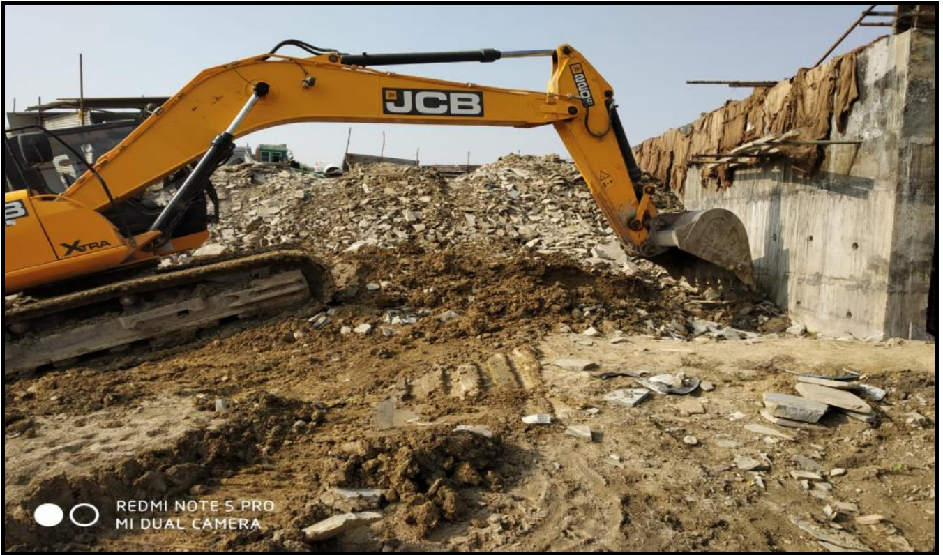
Ch: 22+450 box culvert retaining wall excavation
