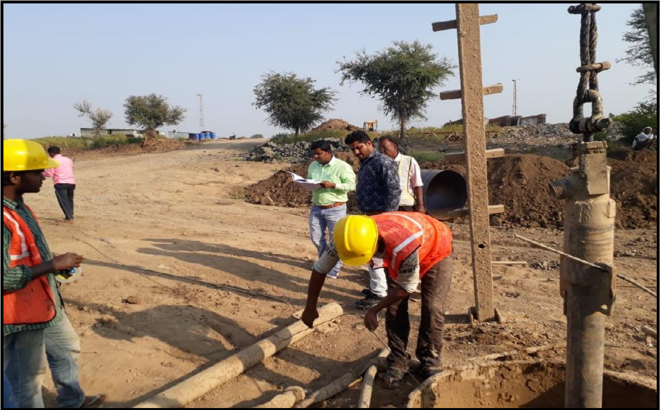
Checking of pile depth at km 36+232 RHS pile no1 major bridge
