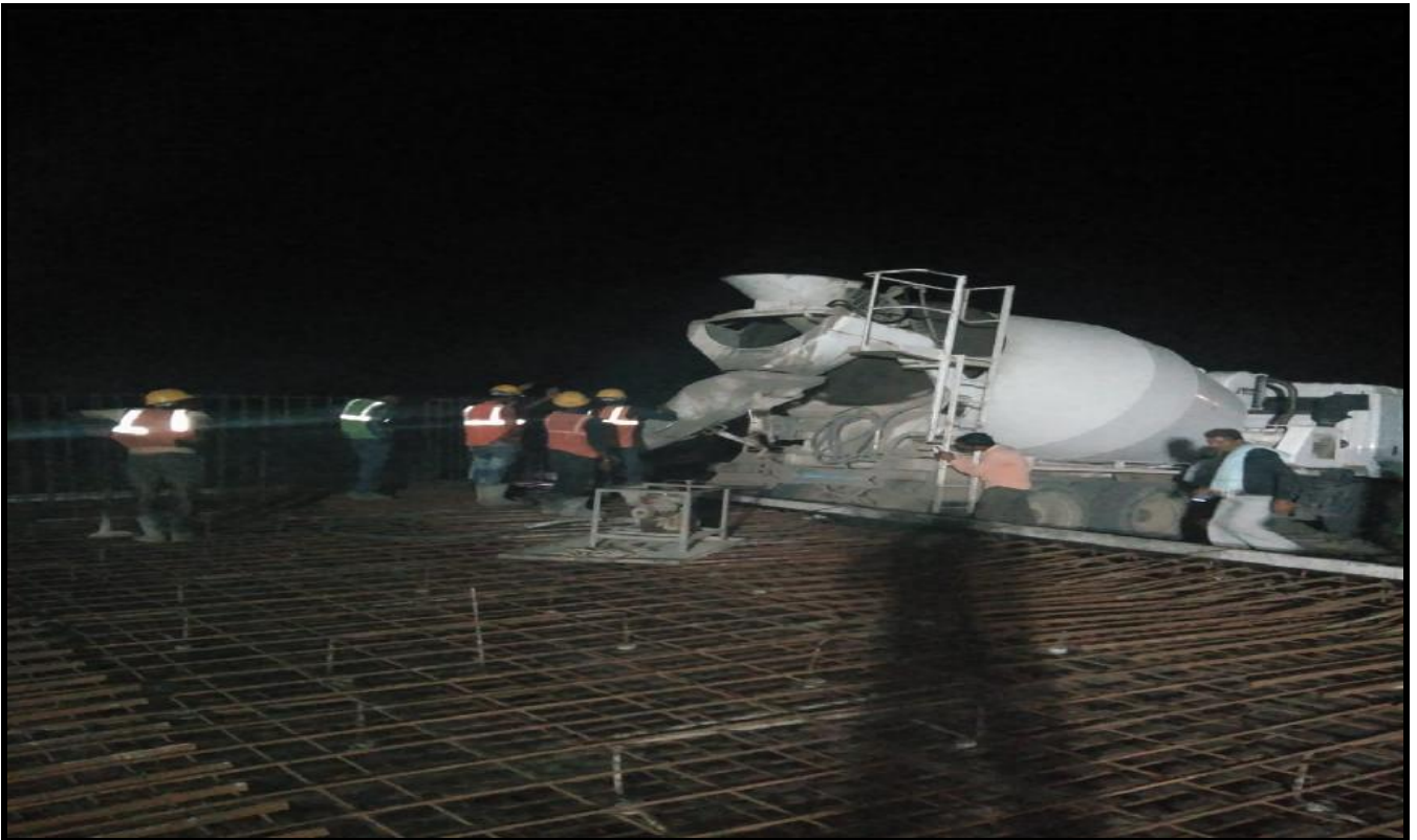
Ch.39+162 box culvert slab casting
