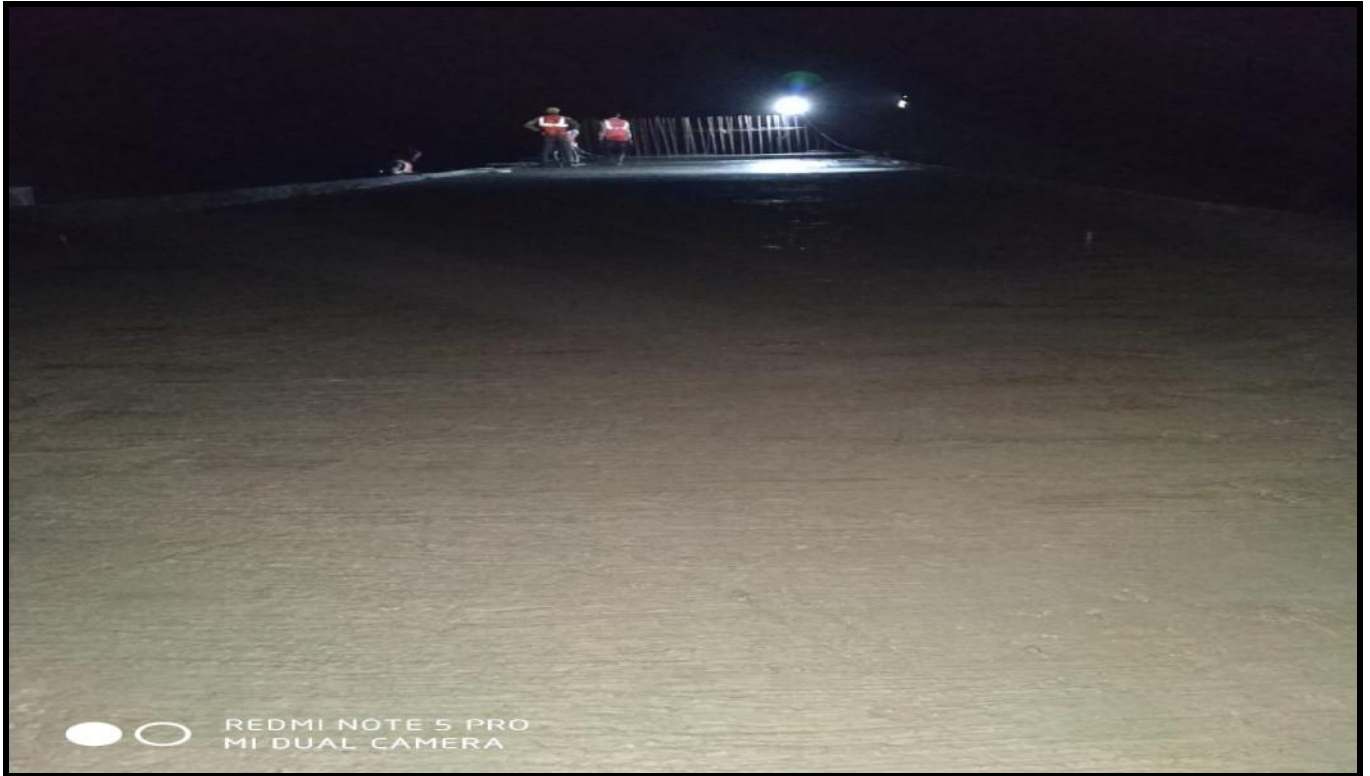
Box culvert 22+450 slab concrete
