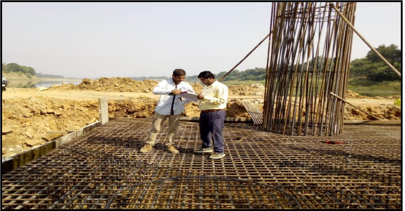
P9 pile cap Checking at Ch 57+127
