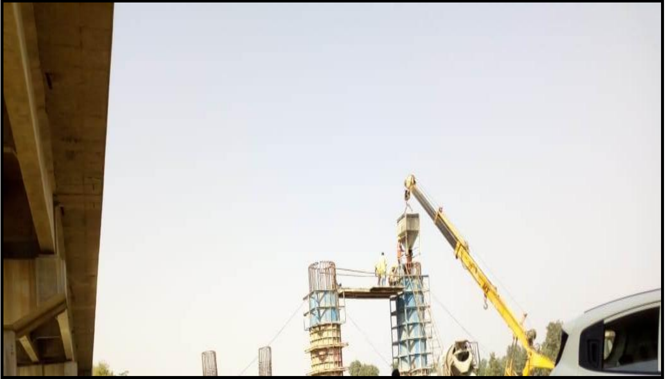
P2 concreting ongoing at Ch 57+127 of pier
