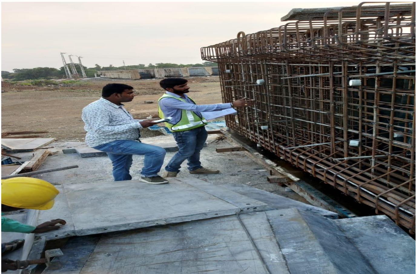
Girder Reinforcement Checking at Ch.47+830
