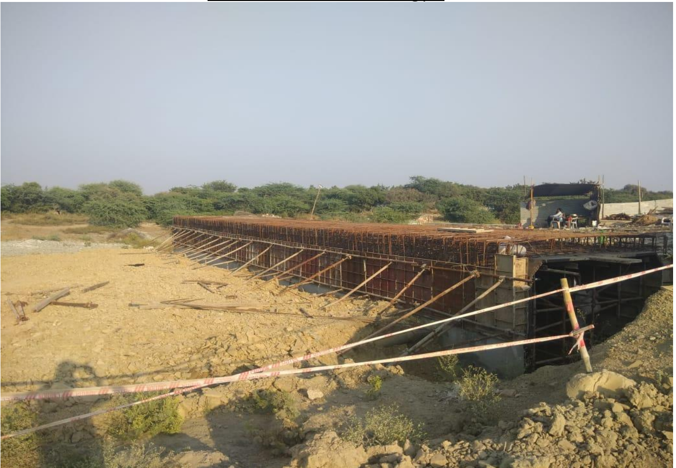
Box Slab Reinforcement Checking at Ch.29+900
