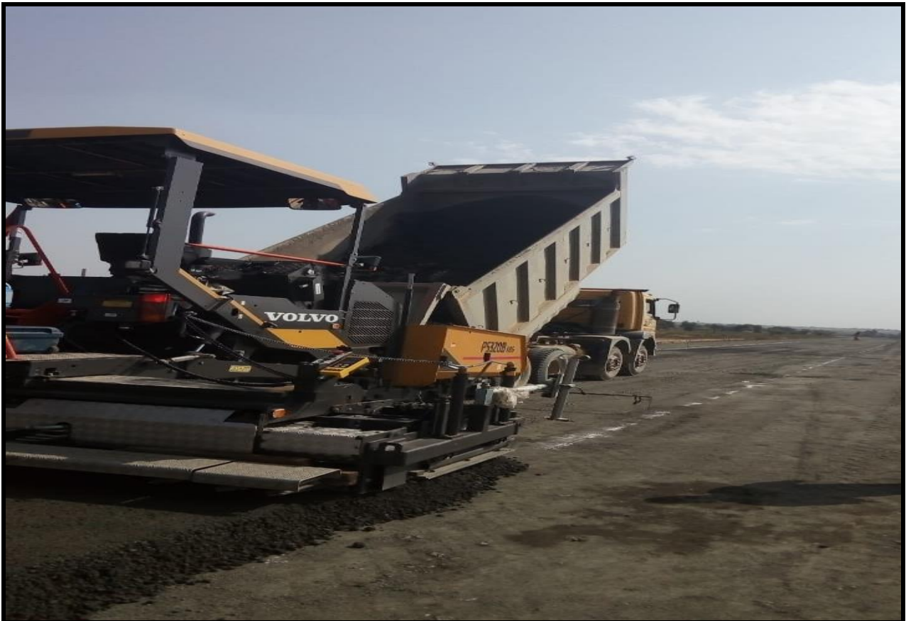
DLC laying at Chainage 28+000
