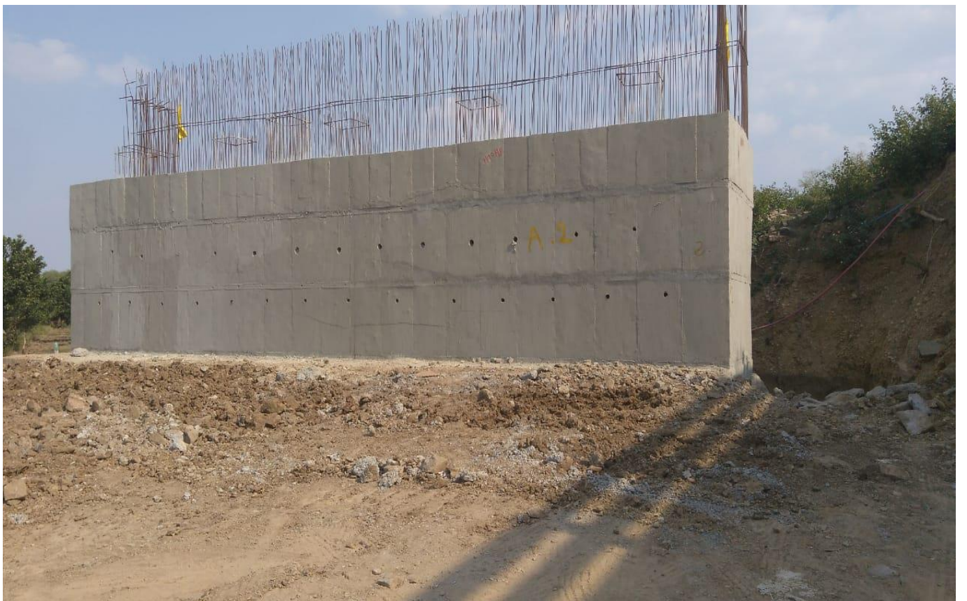
Abutment A-2 Side Ch.57+127 MJB
