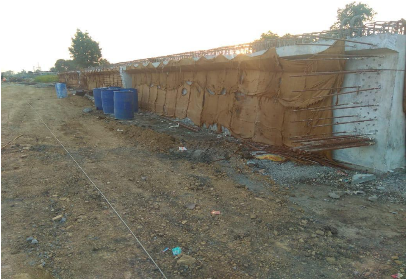
Girder Casting at Ch.26+400
