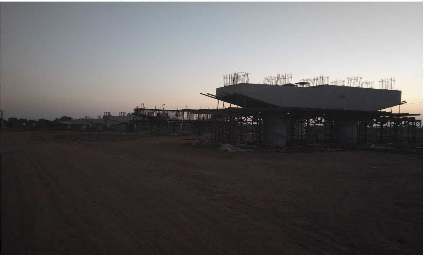
Piers of Elevated Highway(Mela Ground) Ch.47+830.
