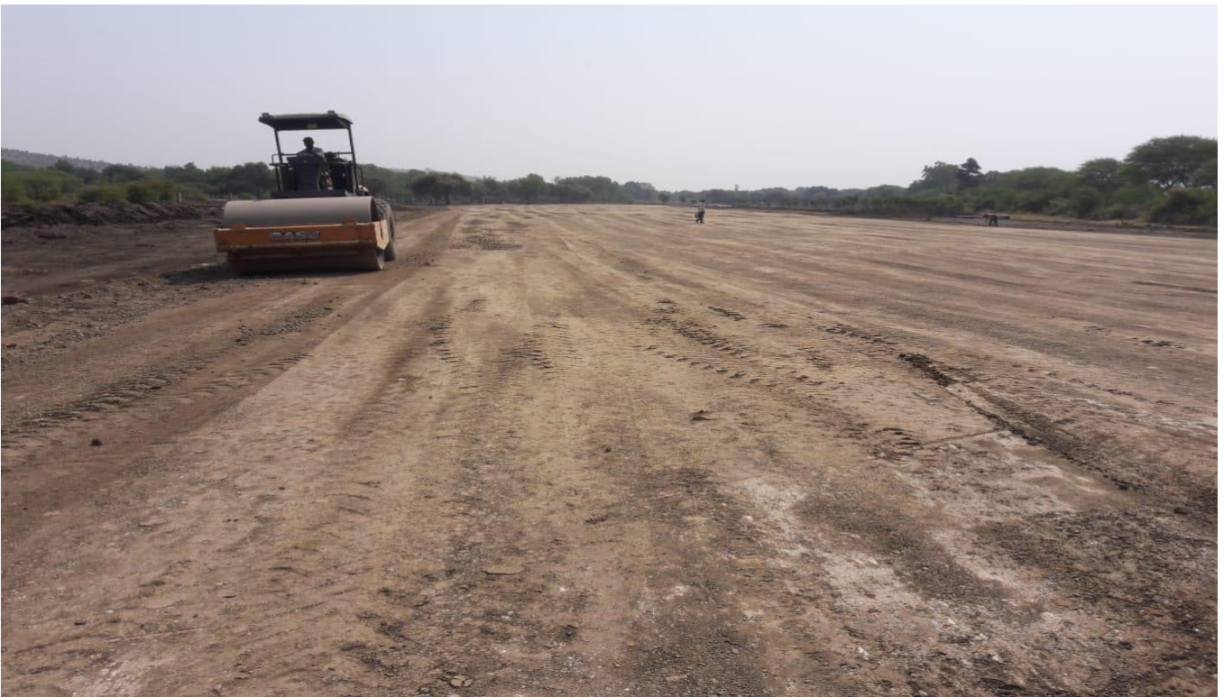
Embankment Layer at Ch.43+700.
