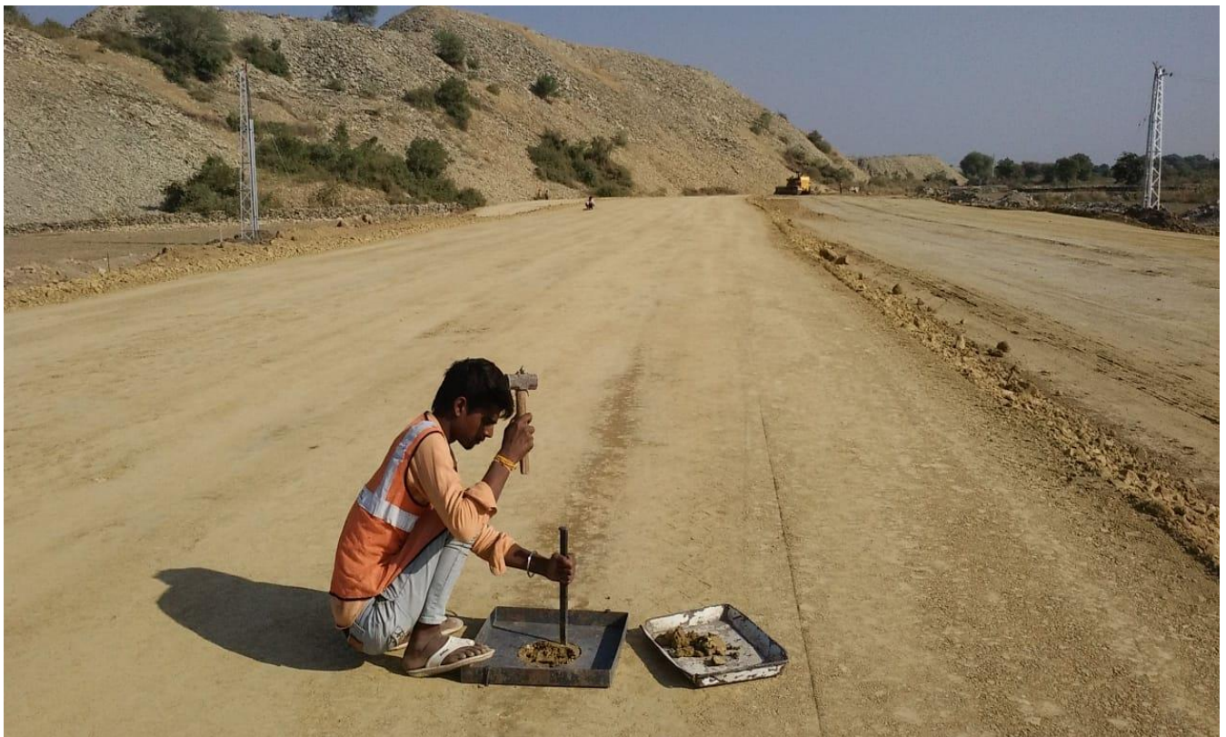
FDD Checking of Subgrade Layer.
