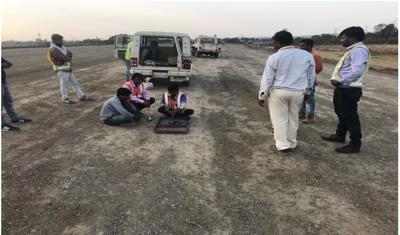
FDD Checking of Embankment Layer.
