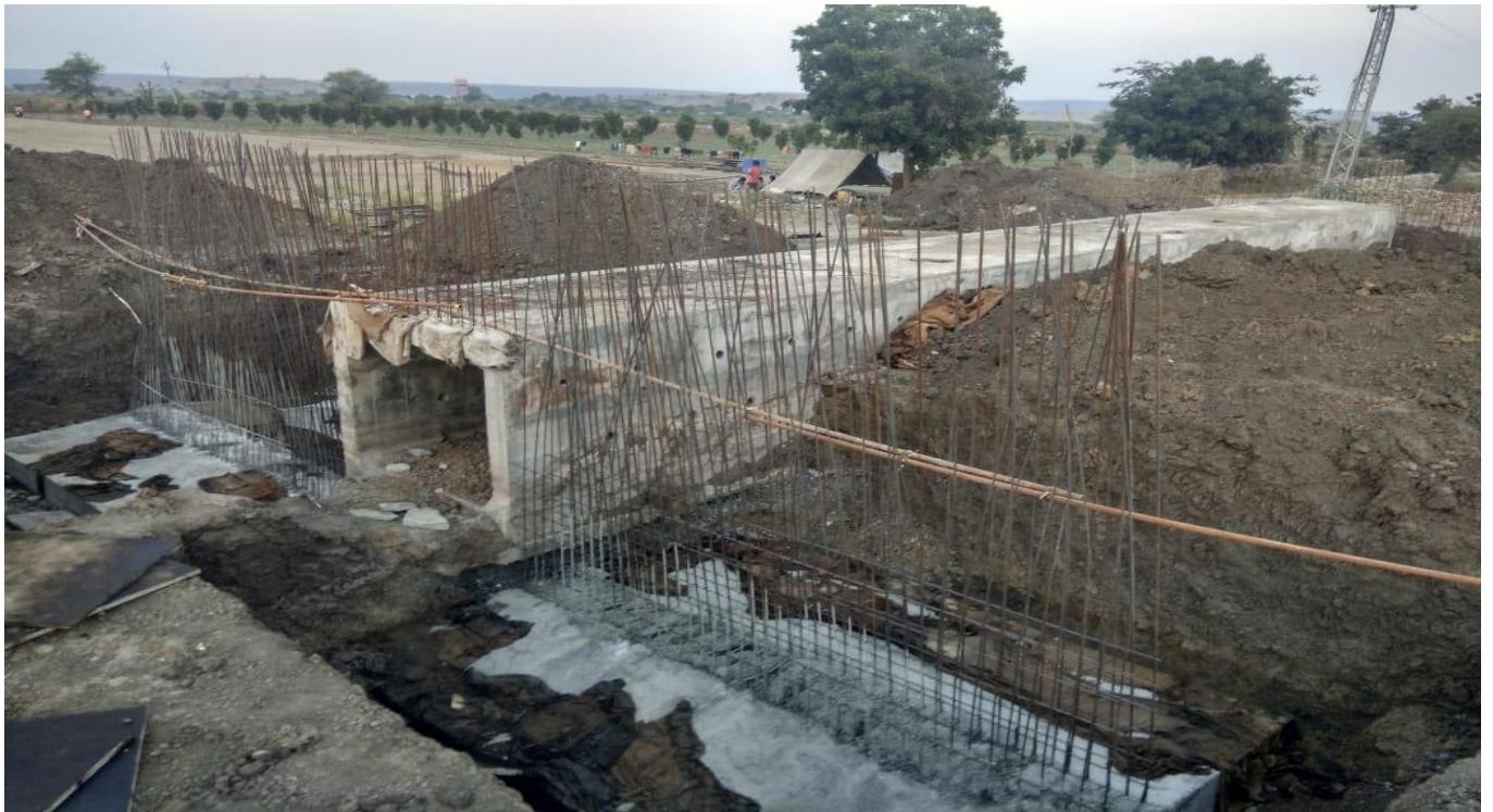
Box Culvert at Ch.13+400
