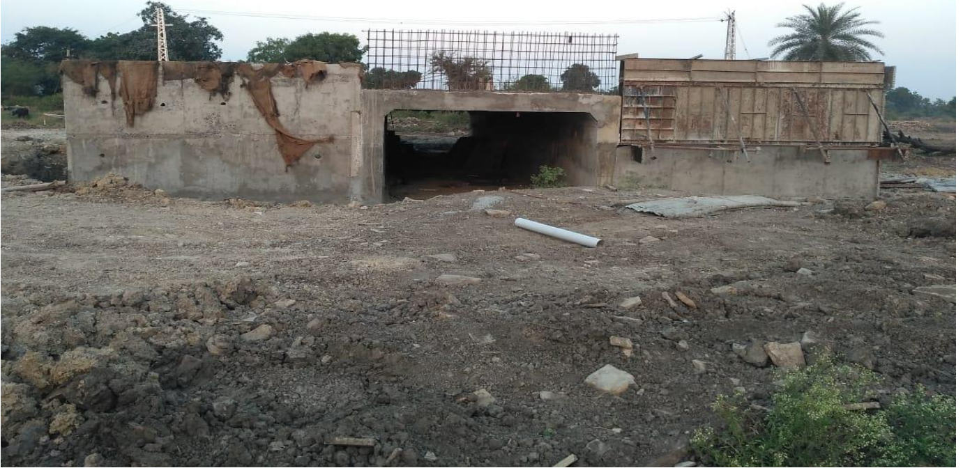
Box Culvert at Ch.16+570
