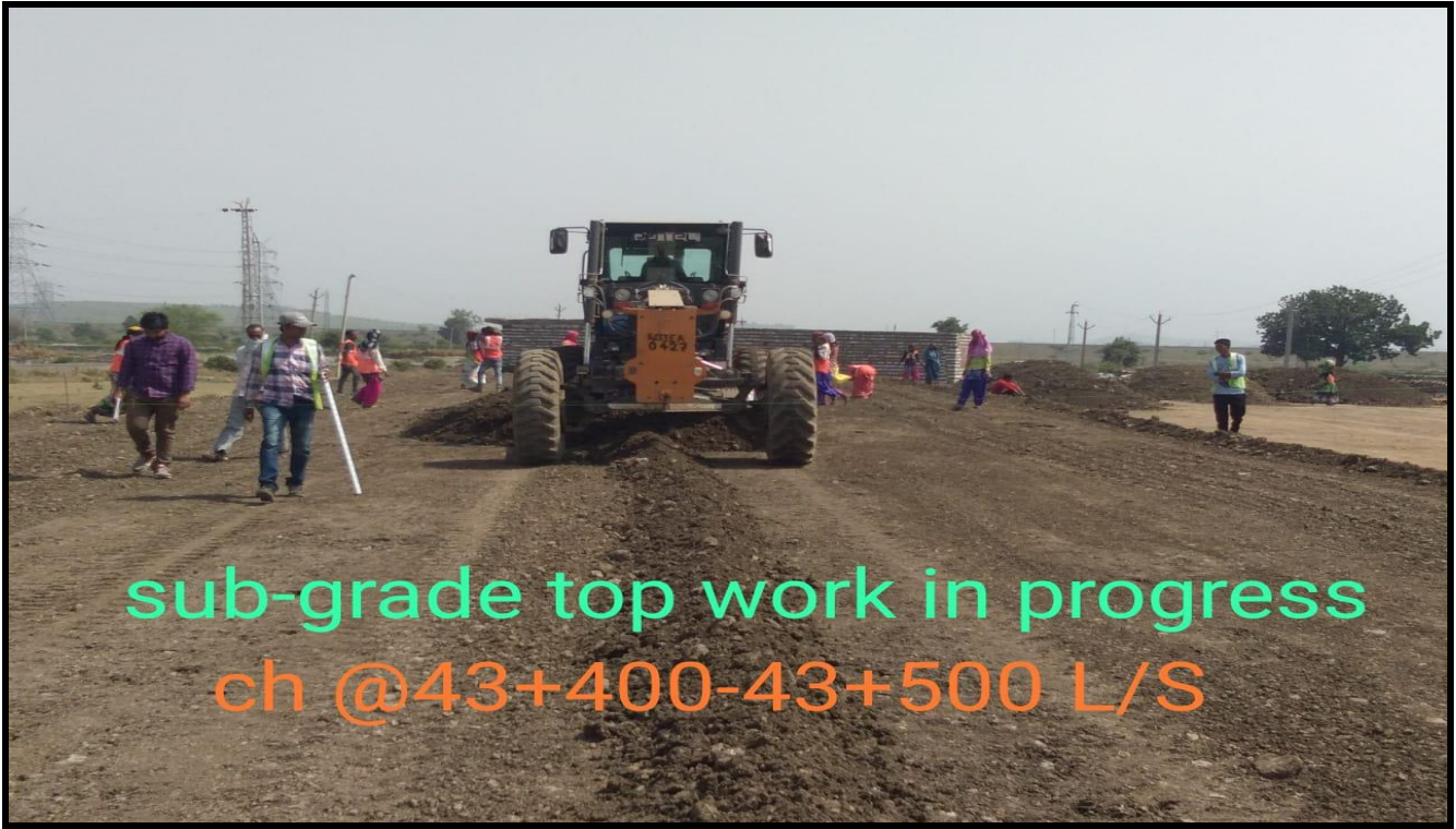
Subgrade Top at Ch.43+400 to 43+500.
