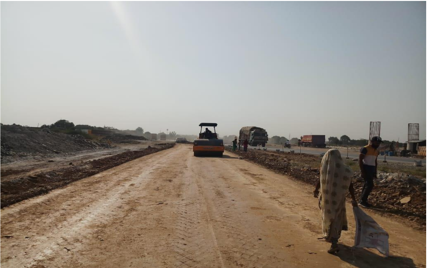
Subgrade Top Layer (SR) Ch.25+000 to 25+120
