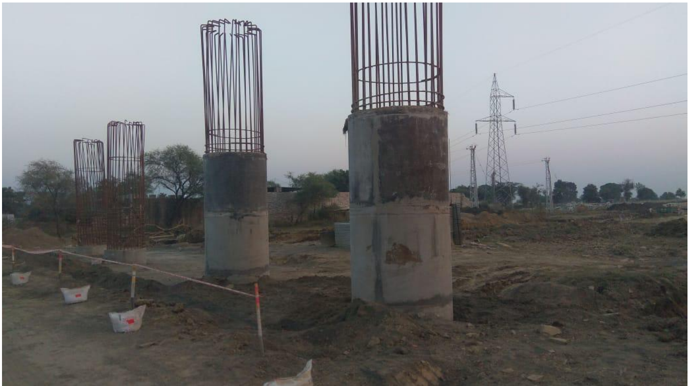
Pier Lift of LVUP at Ch.27+029
