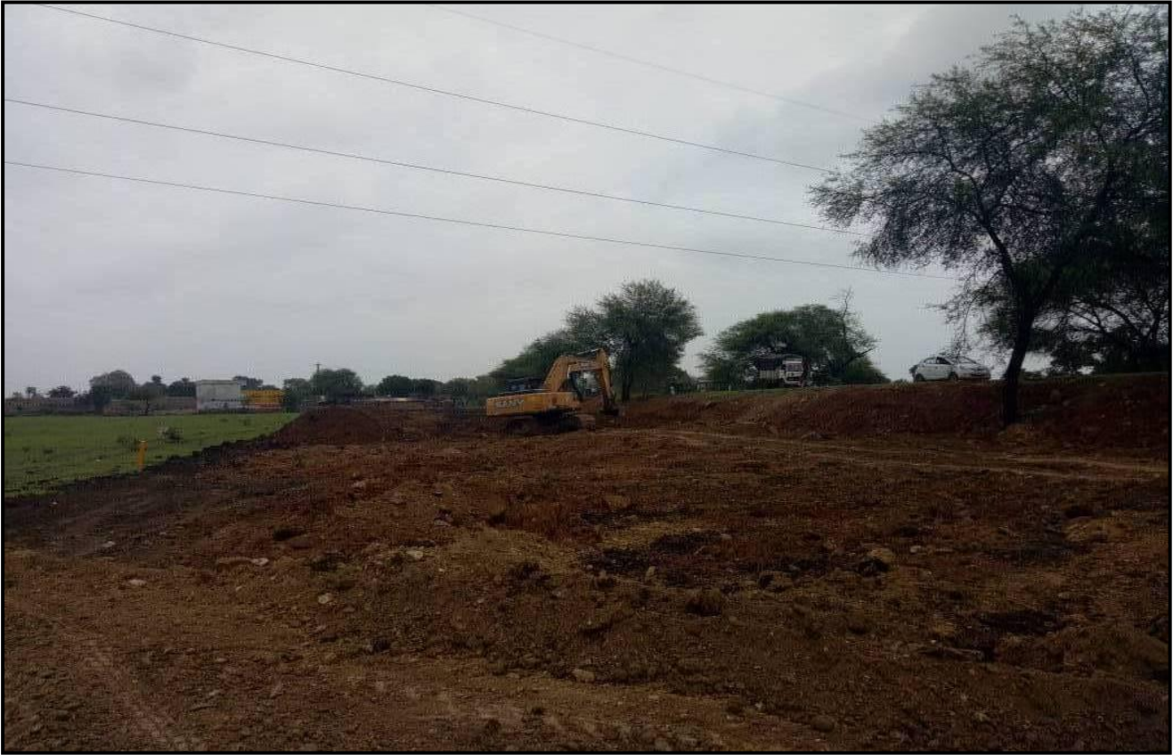
Earthwork at Ch.53+700
