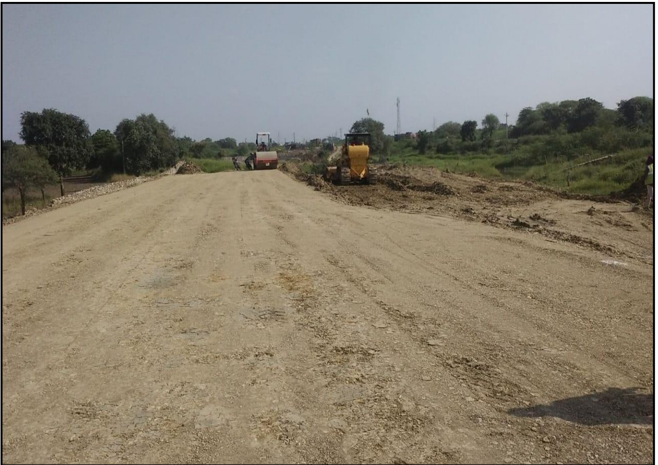
Embankment Layer at Ch.22+100
