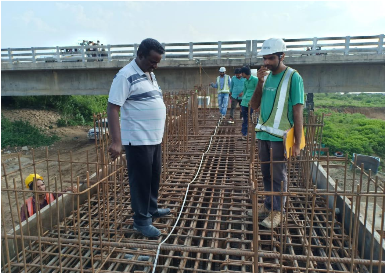
IE is inspecting P-2 Pier cap Reinforcement
