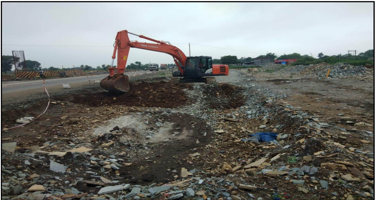
Service Road Excavation at Ch.25+100
