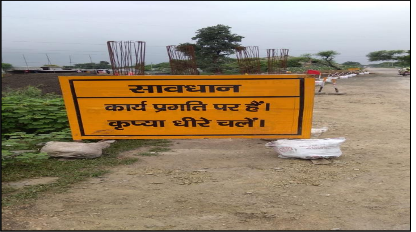
Safety Work at Site Work
