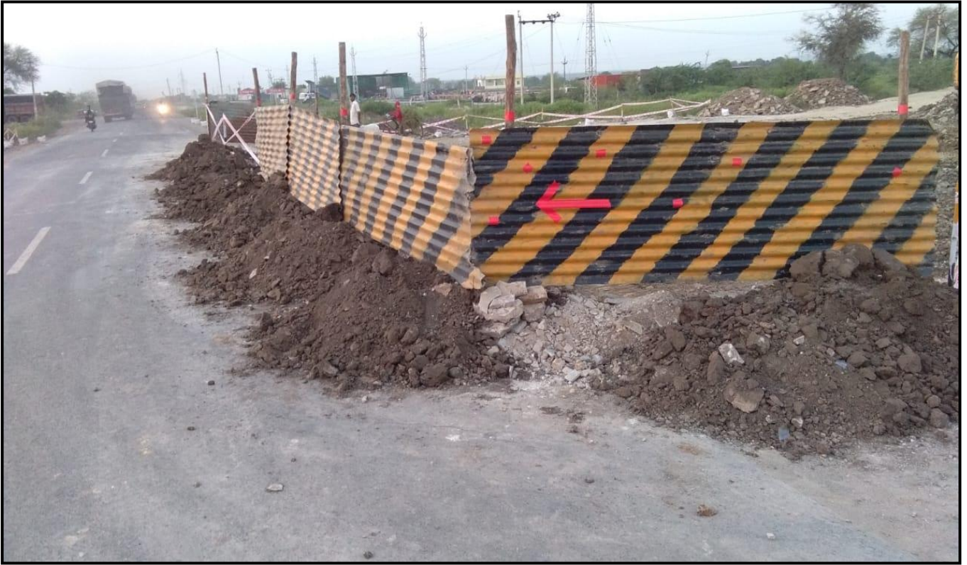
Safety Work at Site Work
