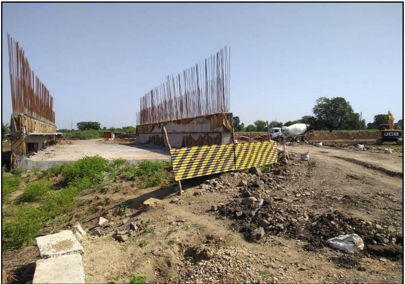
Raft & Wall of LVUP at Ch.37+050
