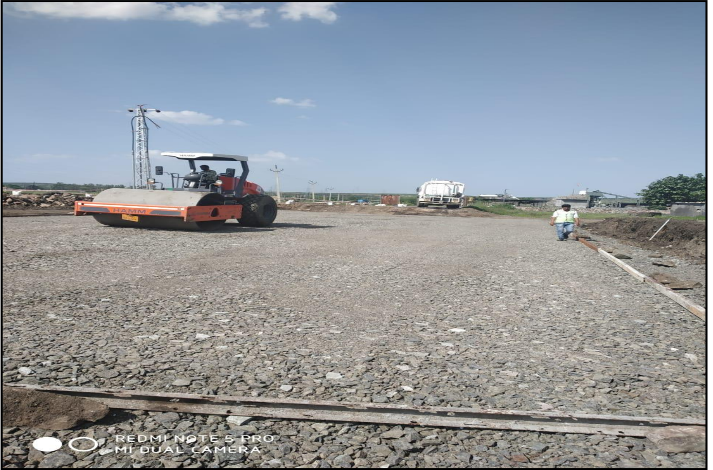
Bed Compaction Complete for LVUP Ch. 42+263
