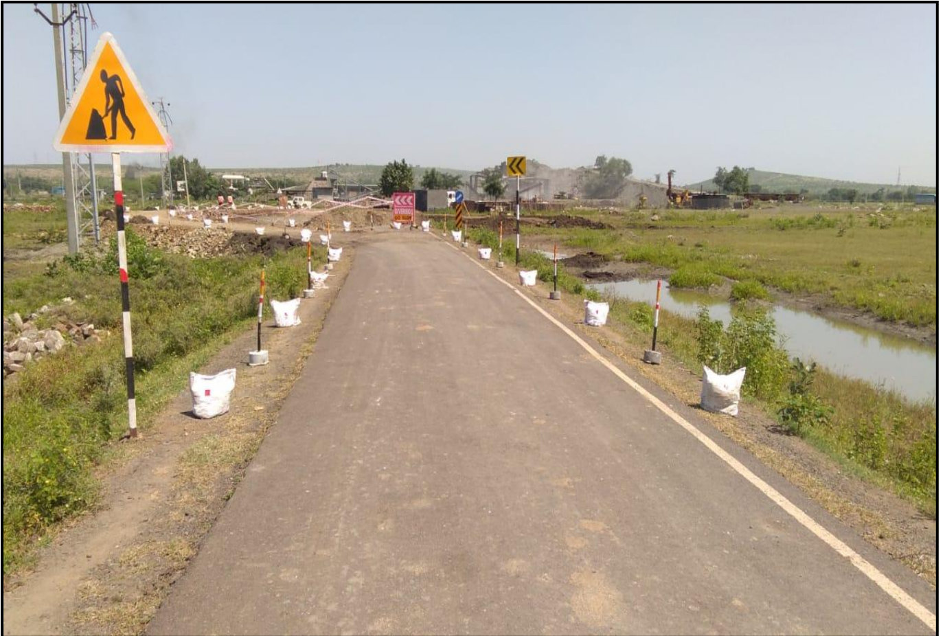
Safety Work at Site Work
