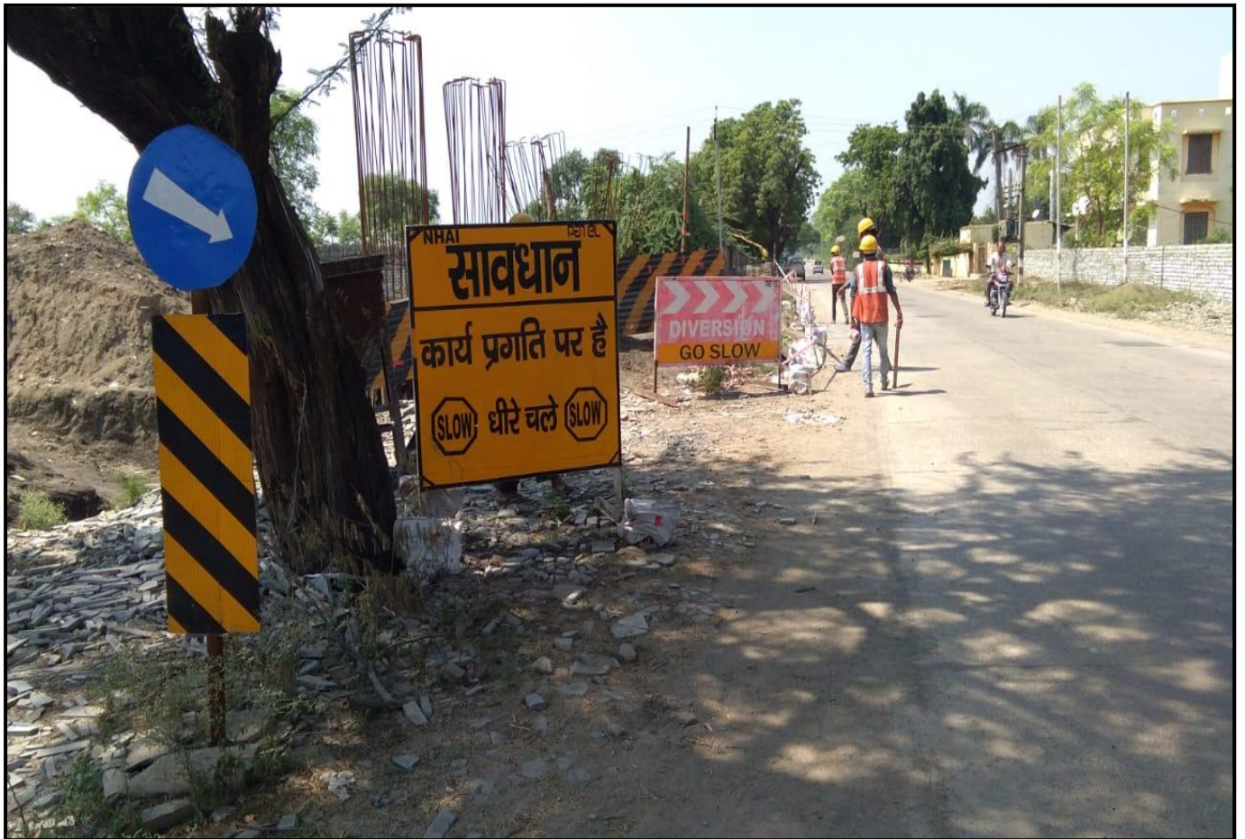
Safety Work at Site Work
