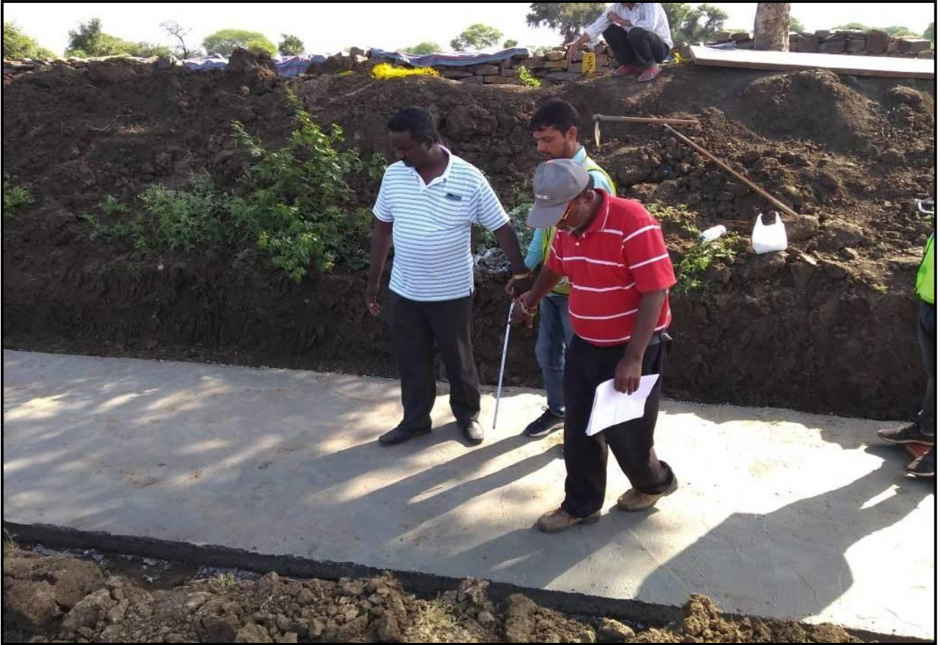
Checking Of Drain Bed Level
