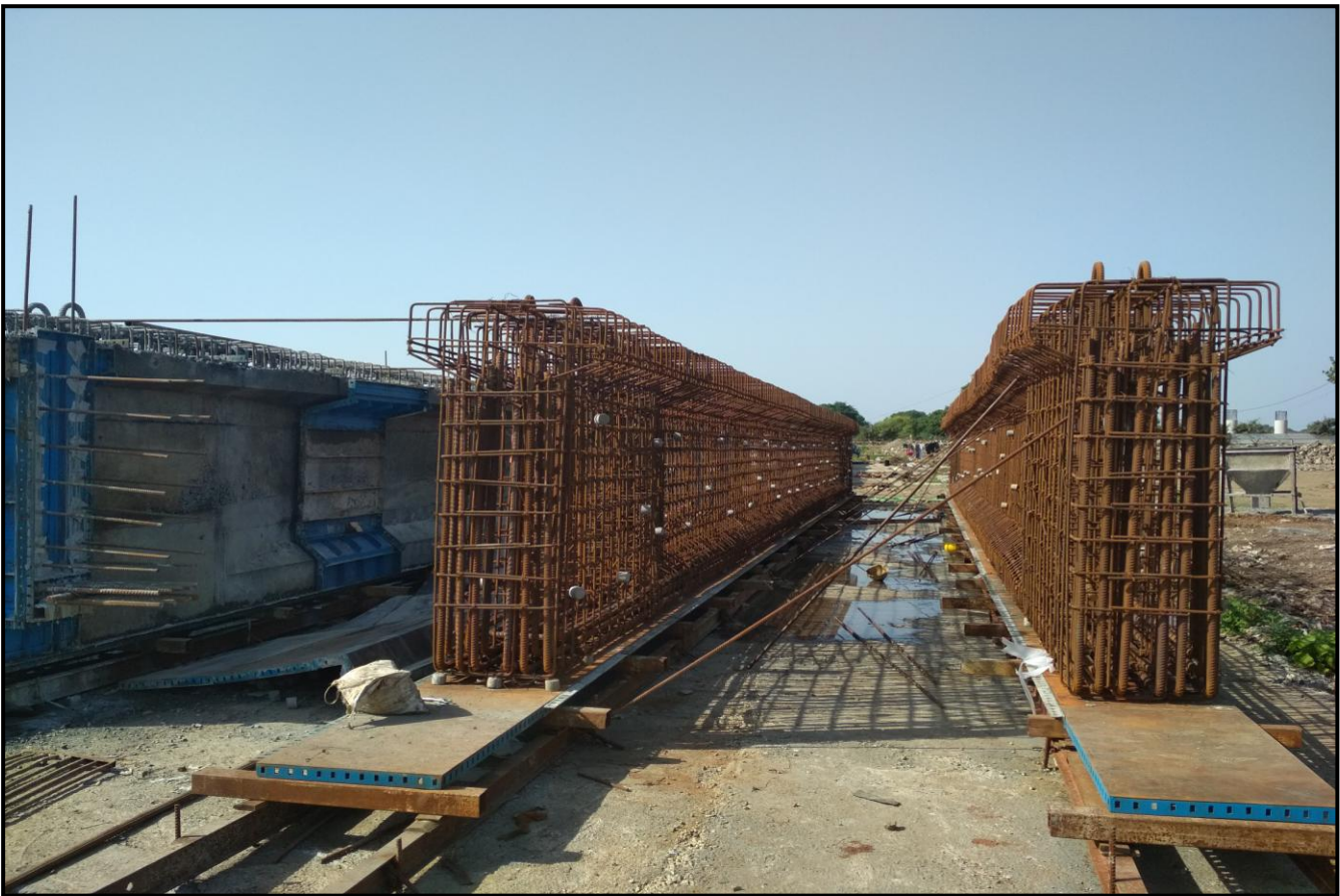
GIRDER Reinforcement Checking at Ch.47+ 650
