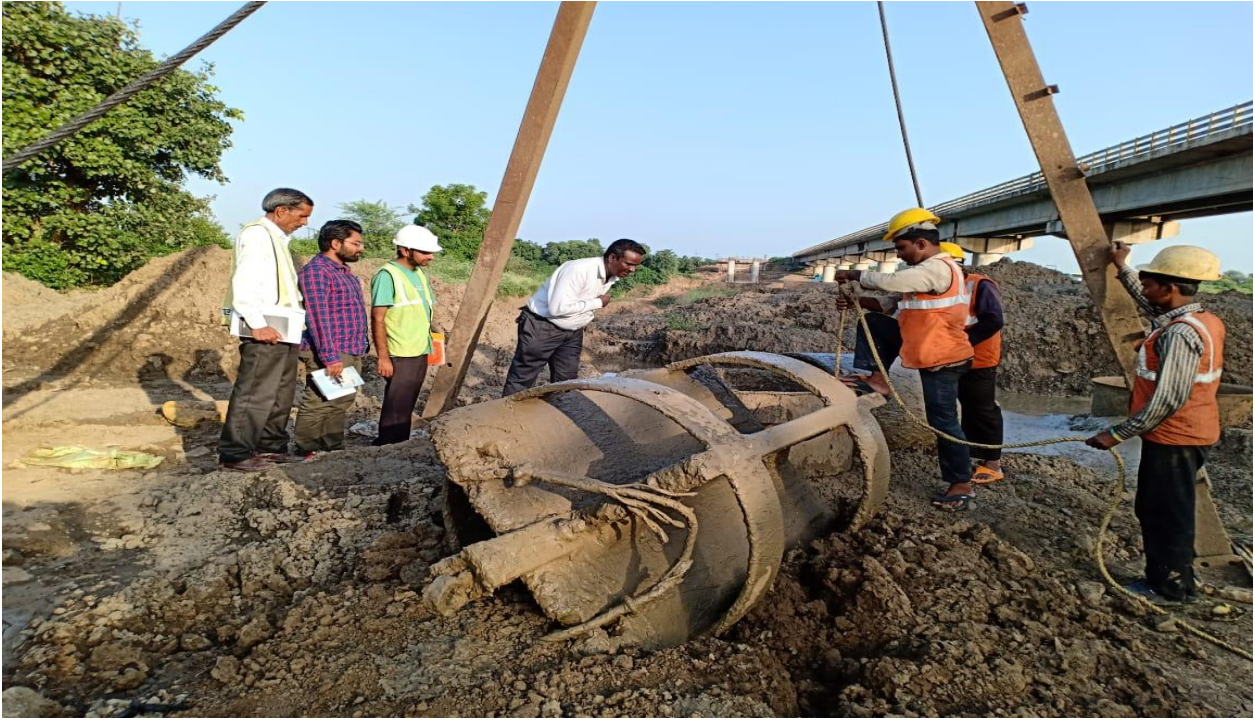
IE inspecting the Pile Work
