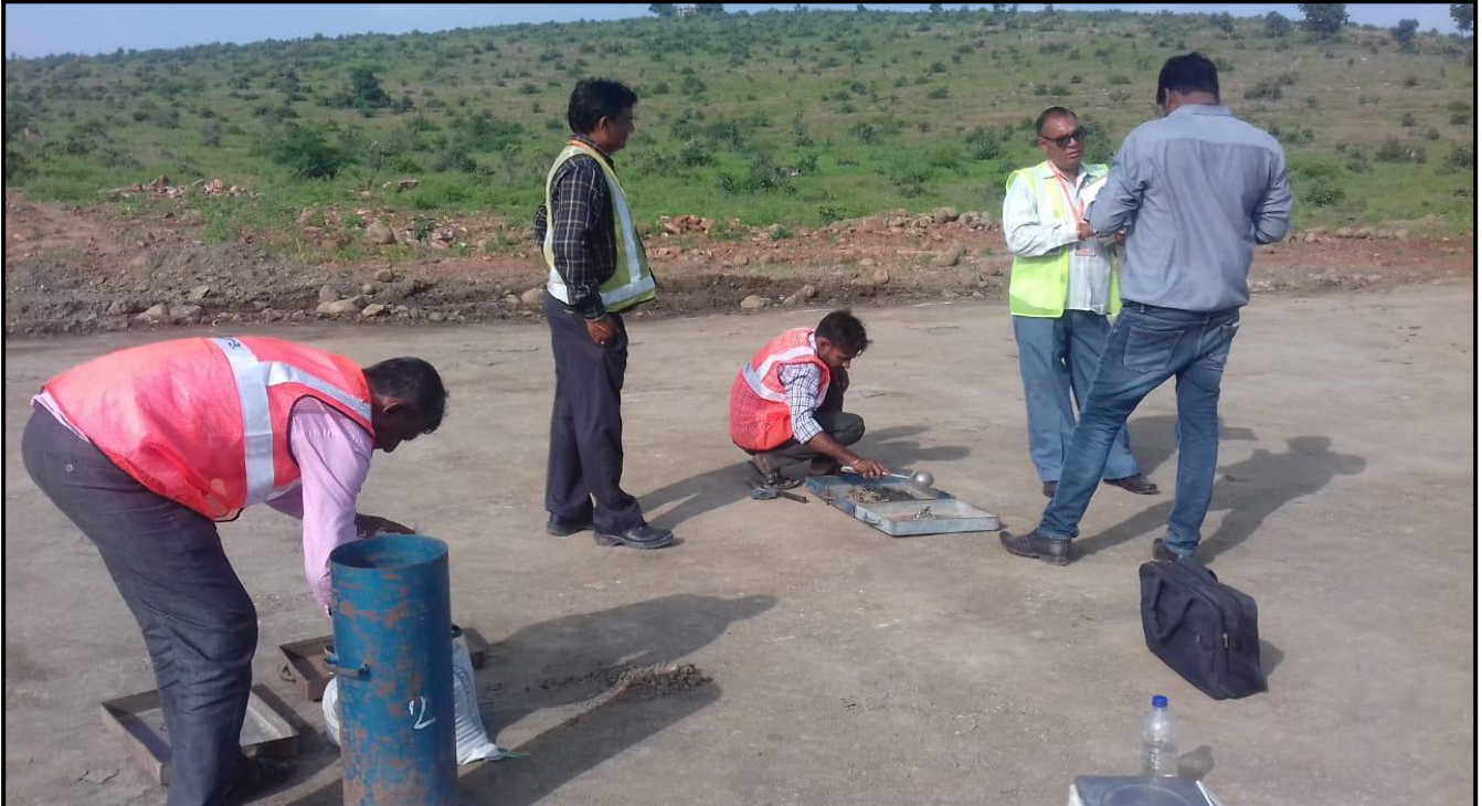
EARTH WORKS- FDD Checking at Ch.53+050
