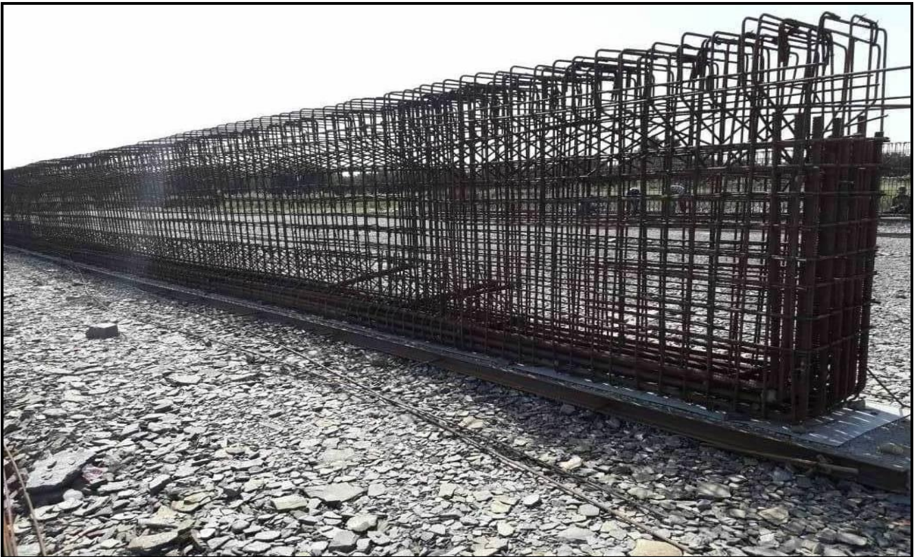
Girder Reinforcement at CH 36+070 MJBR
