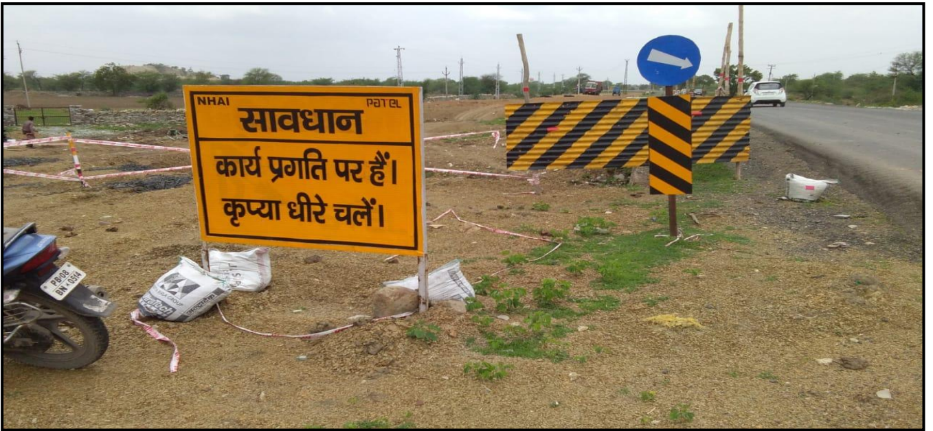
Safety Work at Site Work
