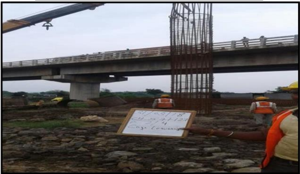
CH 57+127 PIER- 02 PILE NO : 4 ( LOWERING OF CAGE )
