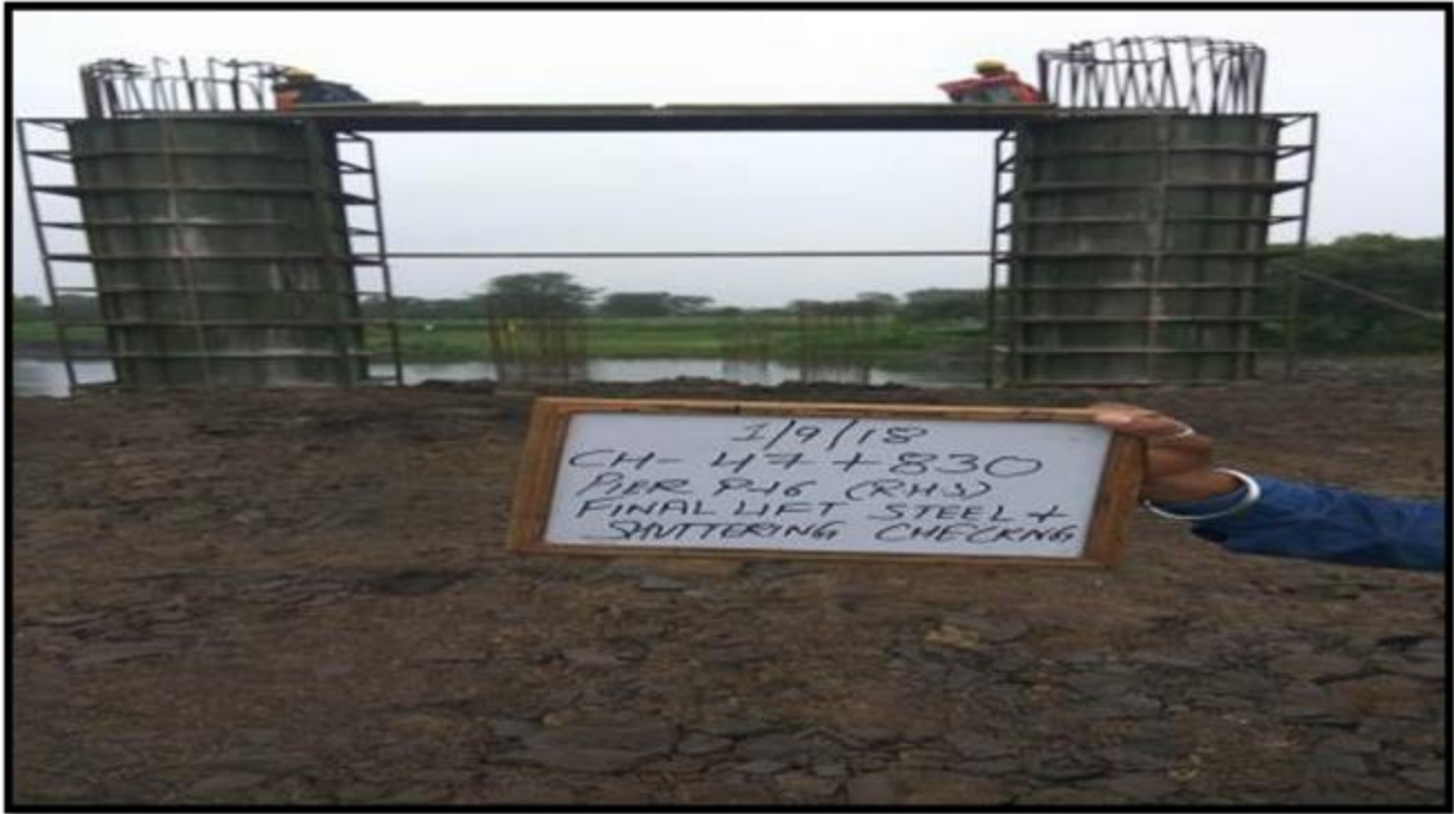
CH -47+ 830 PIER P16 (RHS) FINAL LIFT
