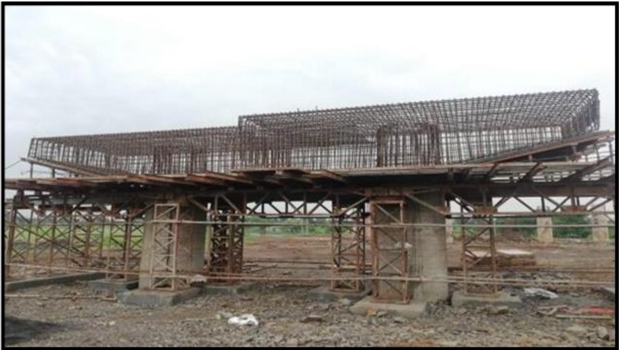
CH -47+ 830 PIER CAP P12 REINFORCEMENT STEEL
