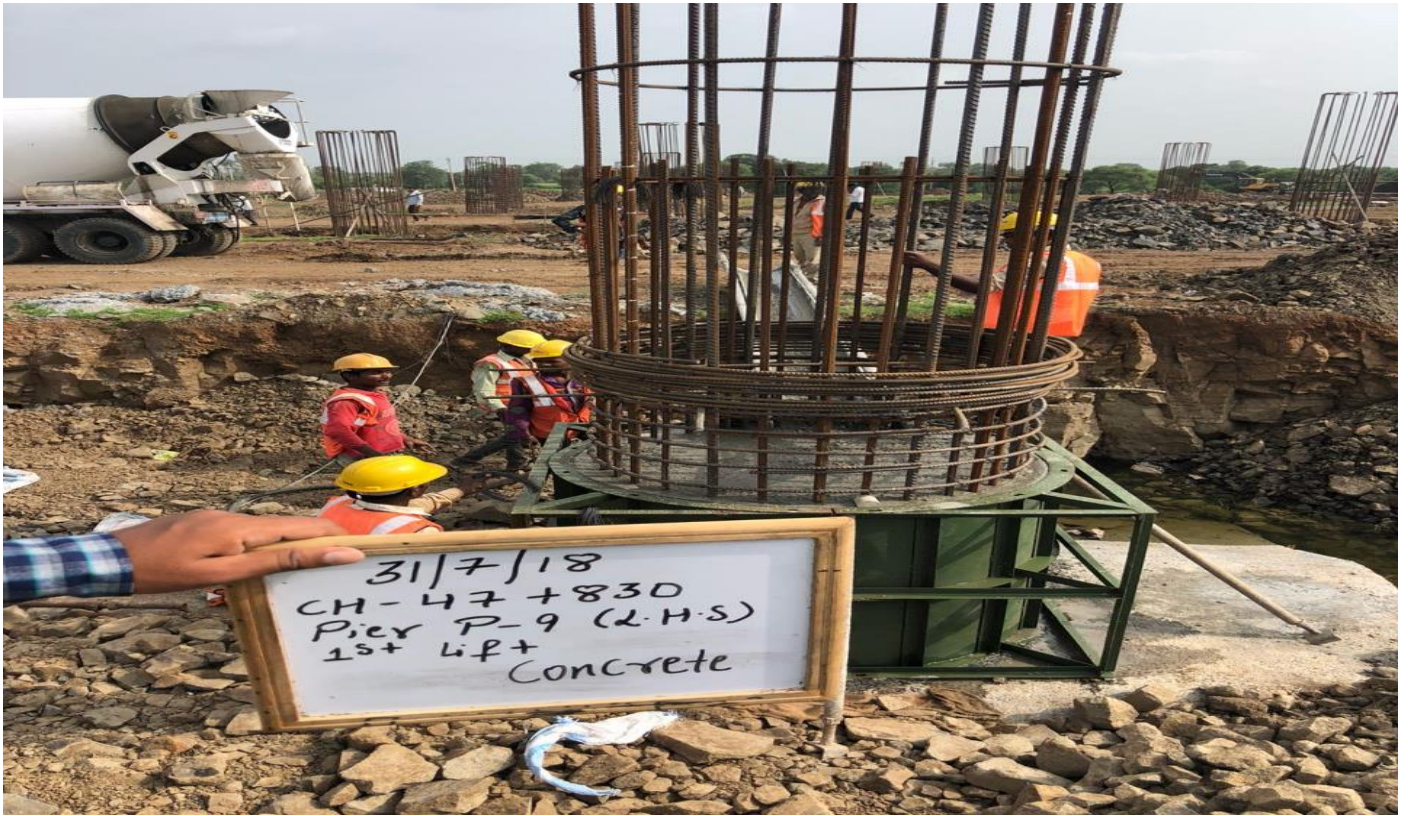
47+830 Elevated Highway Pier P-10 Raft Concrete (RHS)
