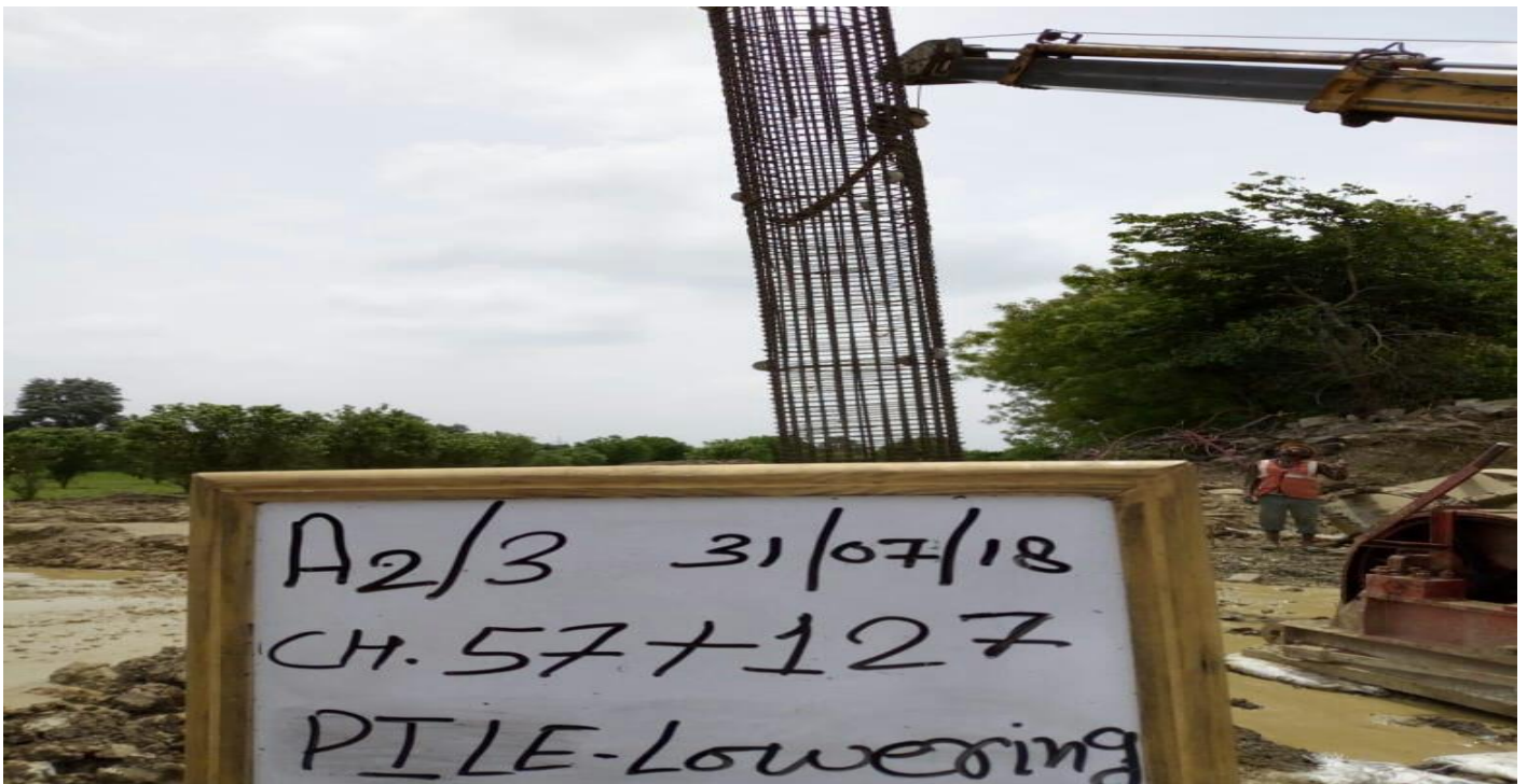
57+127 Major Bridge Abutment A-2 Pile-03 Cage Lowering
