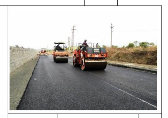
48+892 to 49+330 Rolling work of DBM in SR in progress
