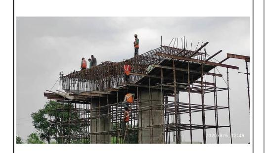
46+950 **FOB**  Reinforcement work of P3 pier cap in progress
