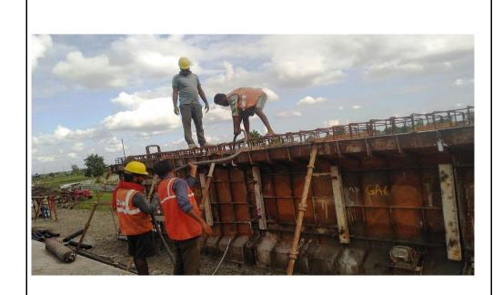
VUP @ 41+102 Concrete pouring work of PSC girder completed
