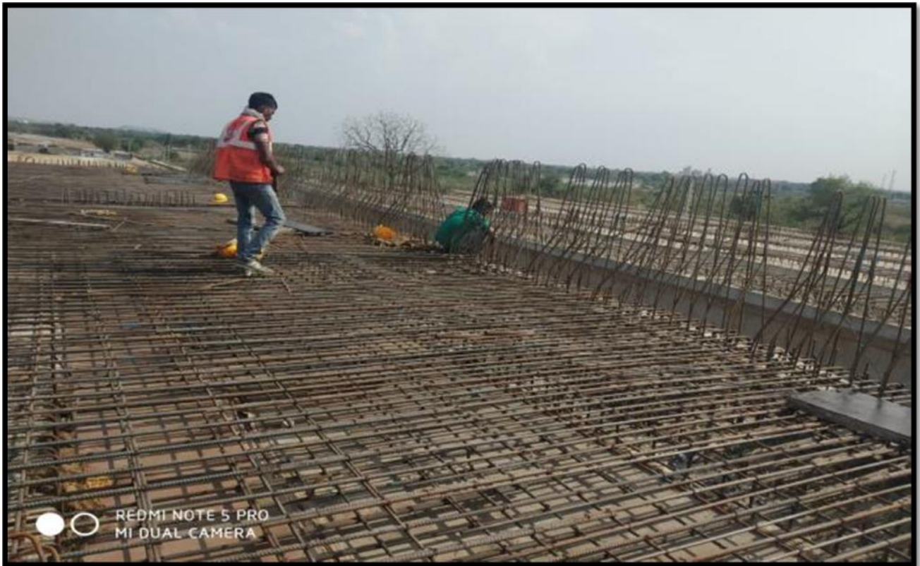
Re-inforce steel work for Slab 15+725
