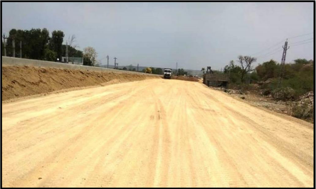
Embankment 5th layer @ Ch. 10+600 to 10+800
