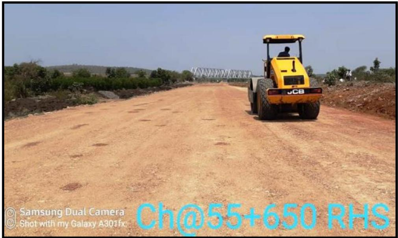
Embankment work in progress @ ch.55+650
