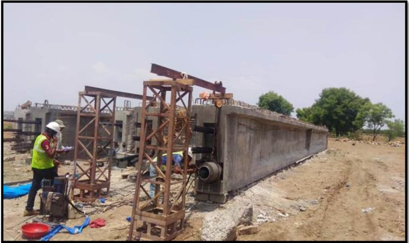
Girder prestressing work of MJB @ ch. 57+127
