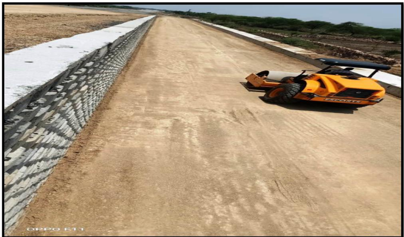
Subgrade top layer @ Ch. 38+290 to 38+530 LHS SR
