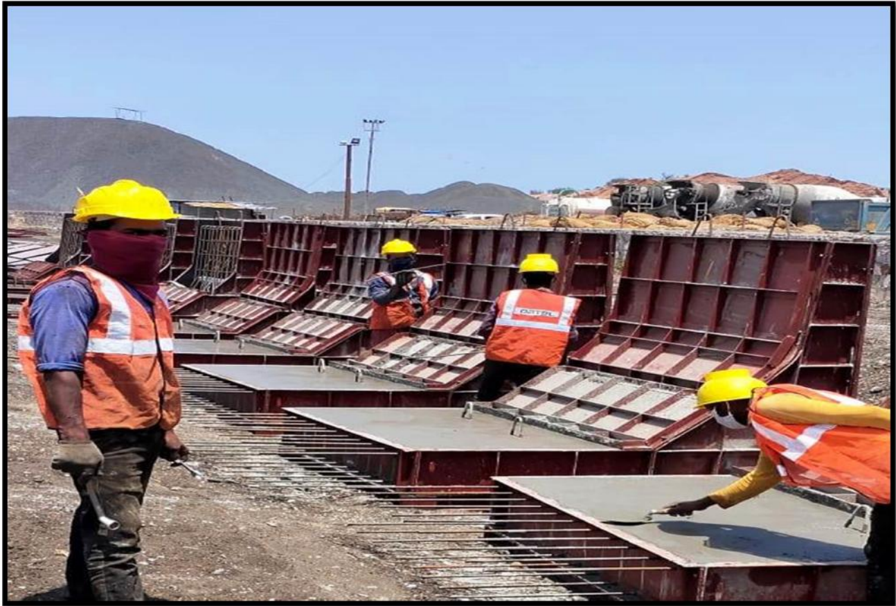
Work in progress of Friction slab with crash barrier
