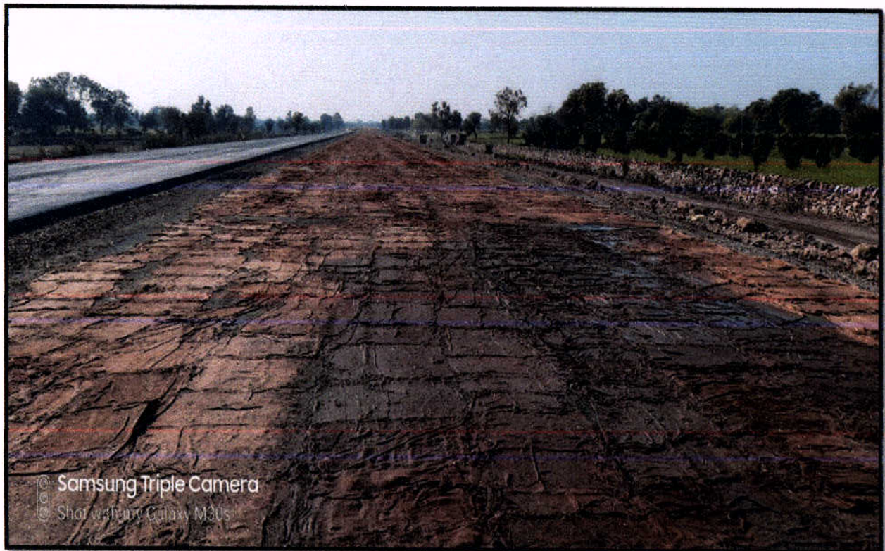
DLC Laying at ch.38+000 to 38+140
