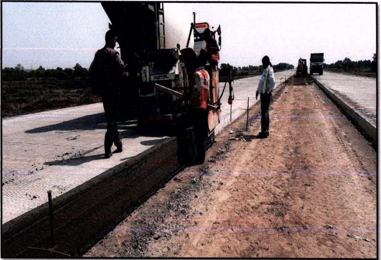
Kerb Laying at Ch 39+300 to 39+400 (LHS)
