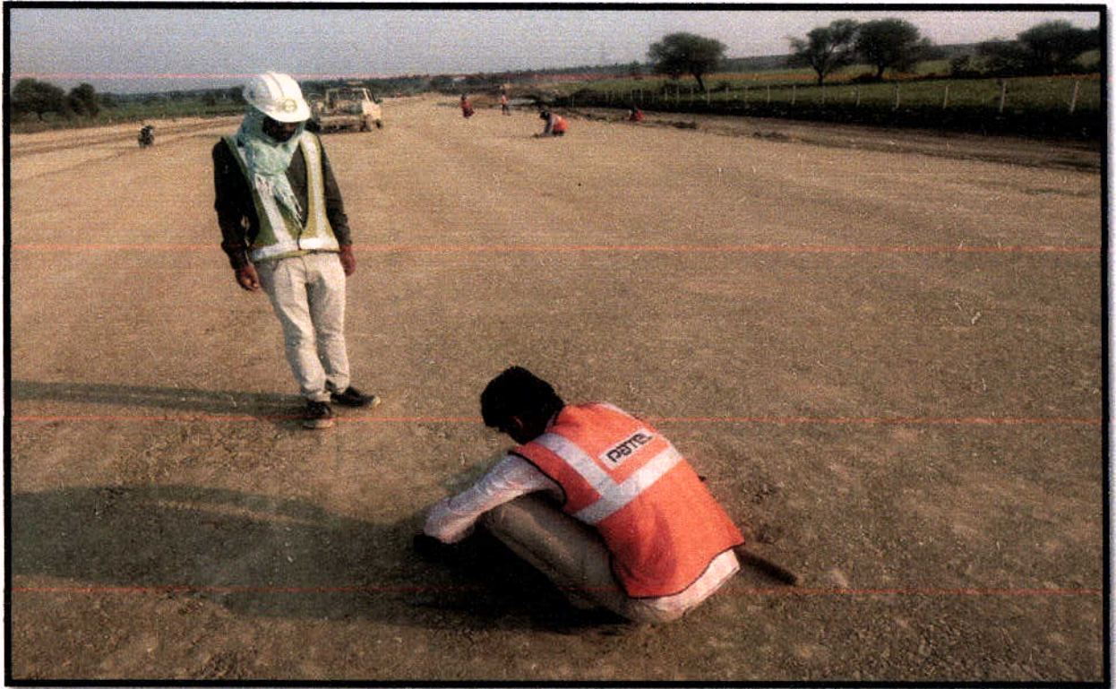
FDD Checking of Subgrade Top at Ch 33+200 to 33+300
