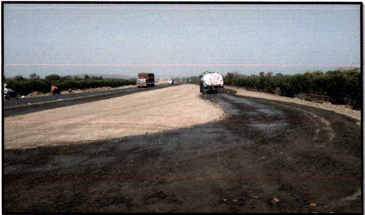
Subgrade Top at Ch 56+200 to 56+400 (LHS)
