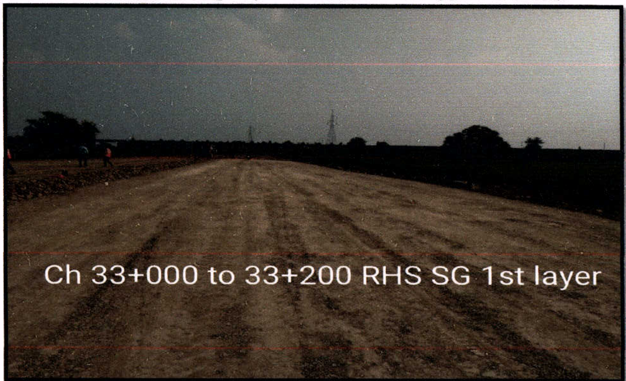
Subgrade 1st Layer at Ch 33+000 to 33+200 (RHS)
