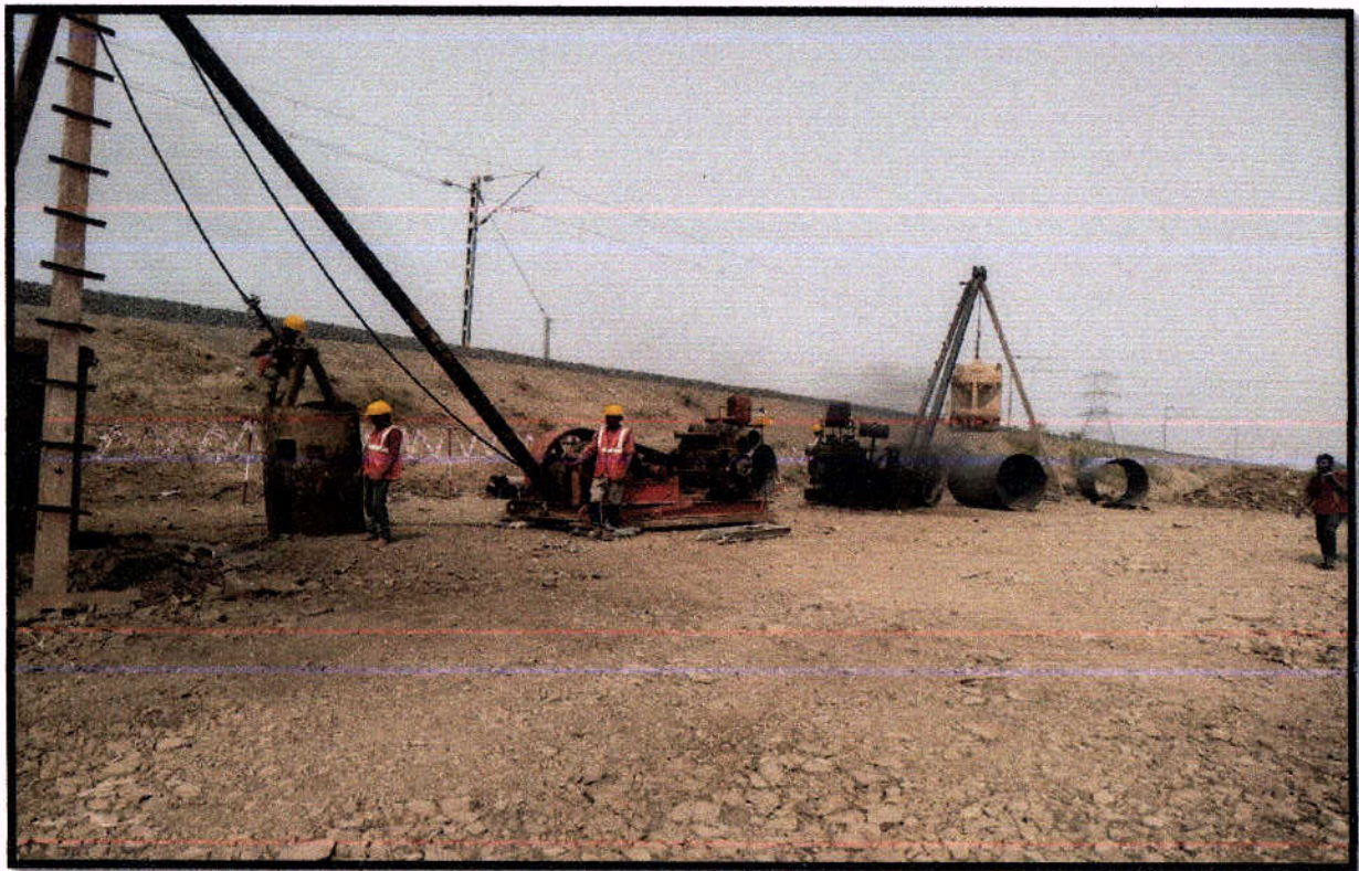
Piling Work in Progress at ROB @ Ch 44+158
