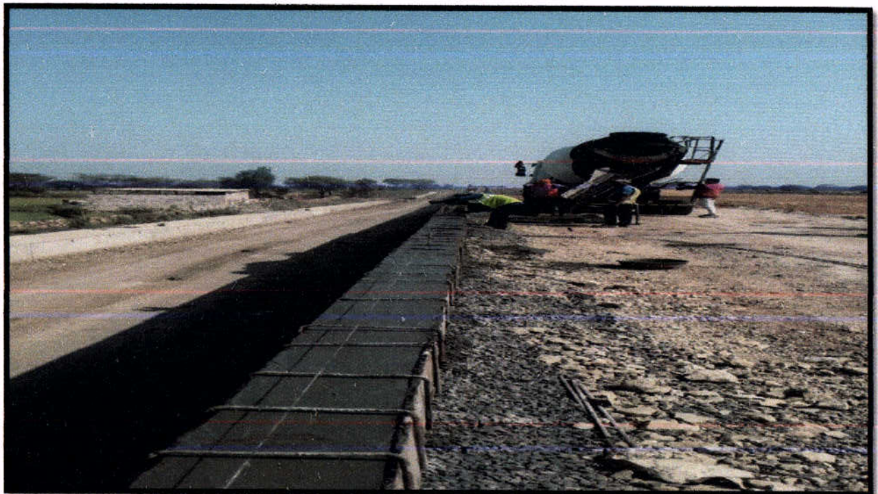
Cooping Beam at Ch 38+300 to 38+400 (LHS)
