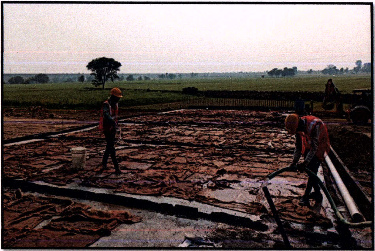
MNB Slab at Ch. 33+000
