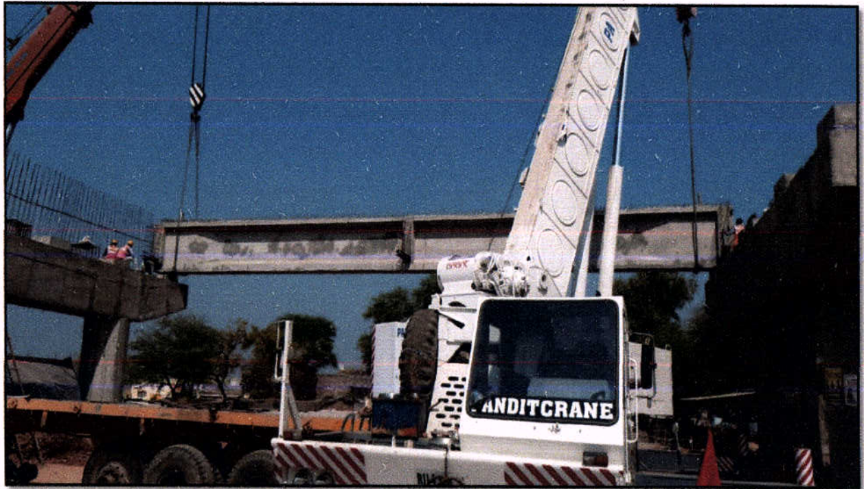
Girder Launching at Flyover @ Ch 58+128
