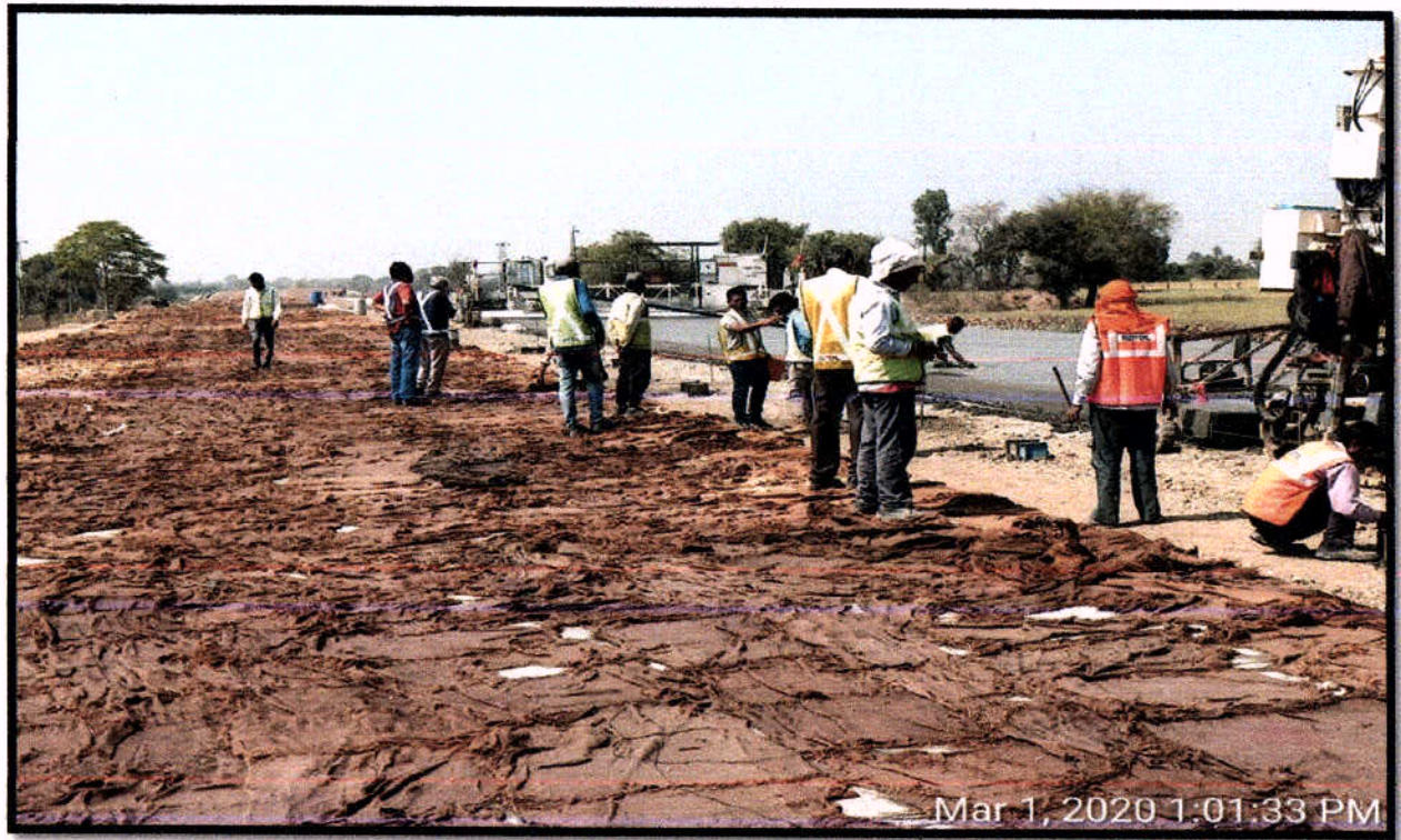
Laying of PQC at Ch37+540
