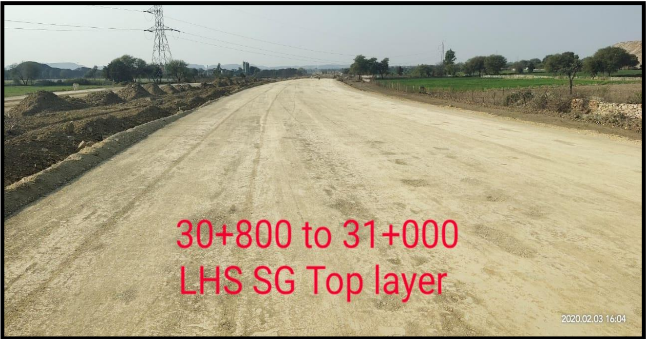
Subgrade Top Layer at Ch 30+800 to 31+000 (LHS)
