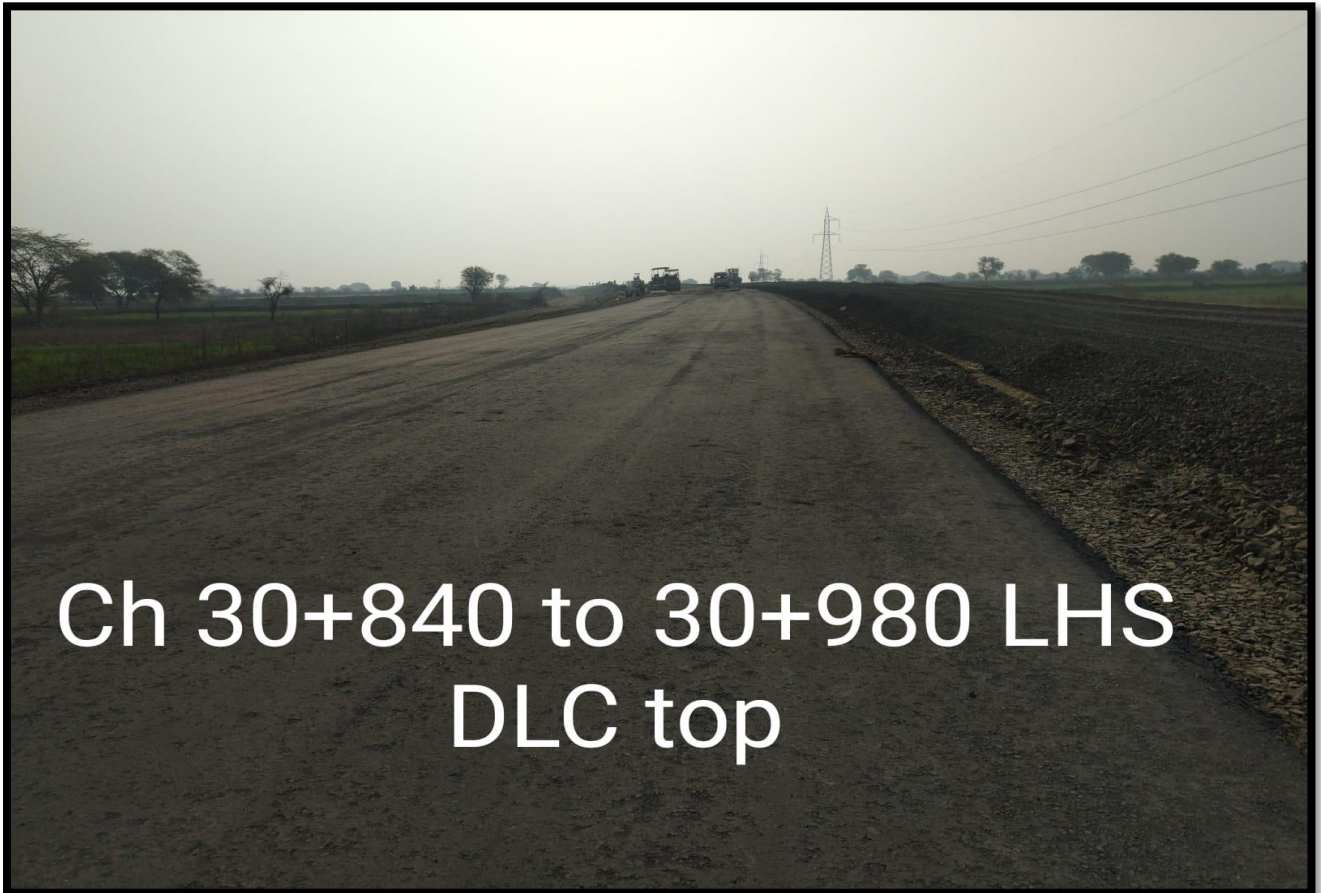
DLC Laying at ch.30+840 to 30+980 (LHS)
