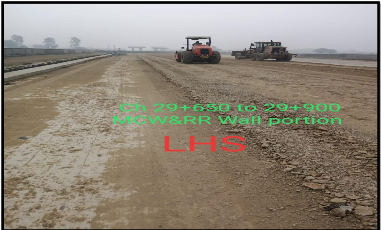
RE Wall portion soil filling & MCW at Ch. 29+650 to 29+900
