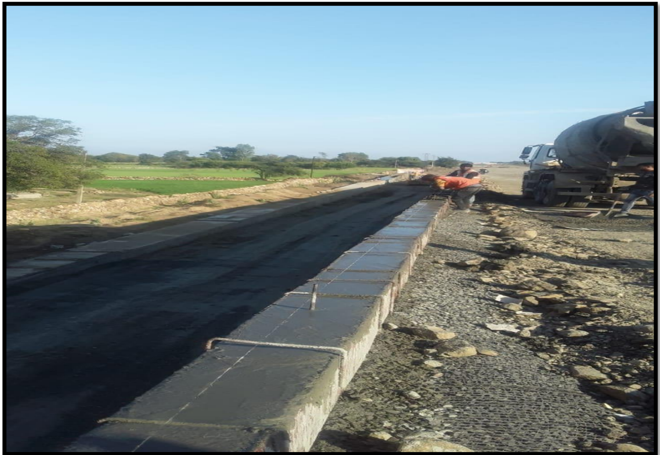
RE Wall Cooping Beam at Ch.37+055 to 37+206 (LHS)
