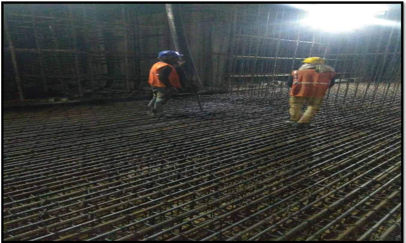
Raft of Minor Bridge MCW at Ch. 12+380 (BHS)
