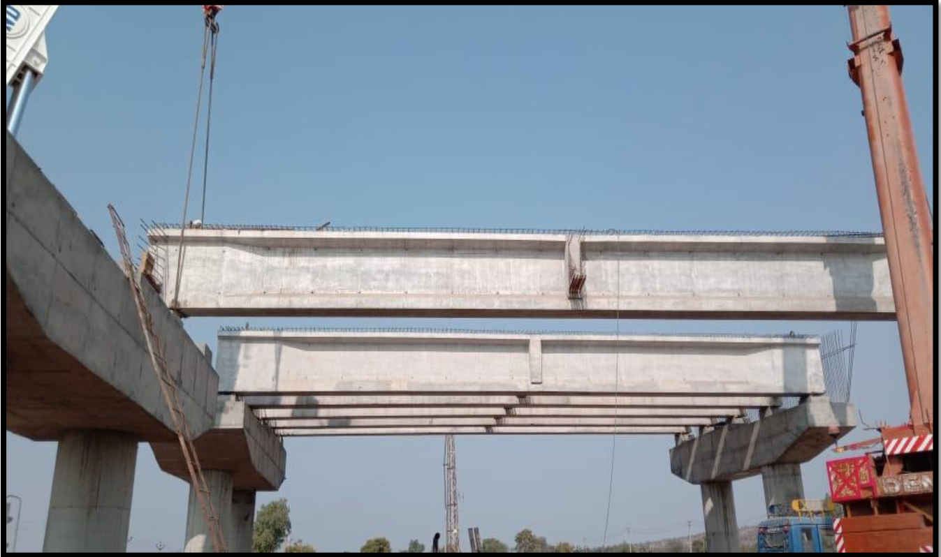
Girder Launching from Pier P-2 to A-2 at FOB Ch 50+095 (RHS)
