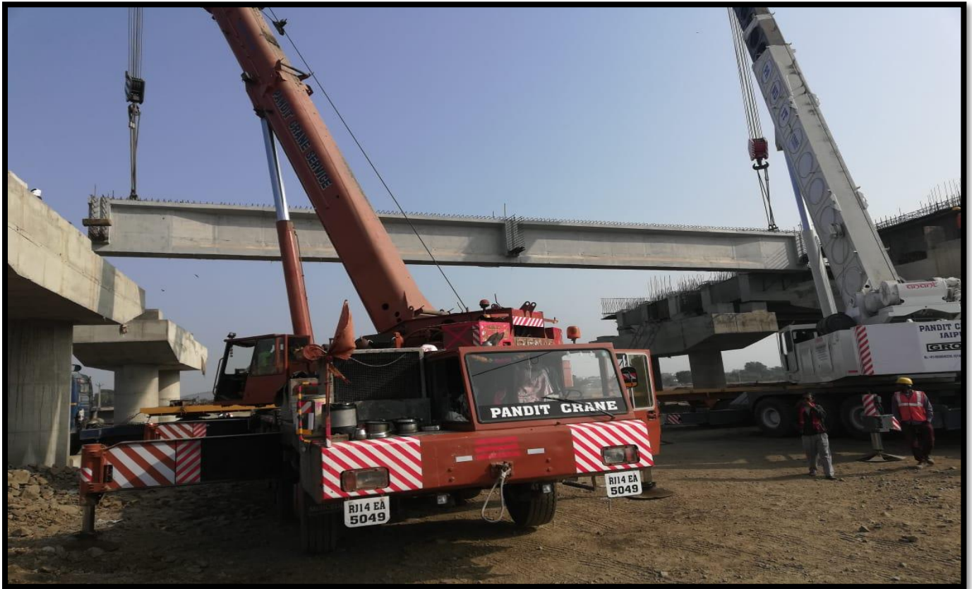
Girder Erection on P-4 to P-5 at Elevated Highway @ Km 47+830
