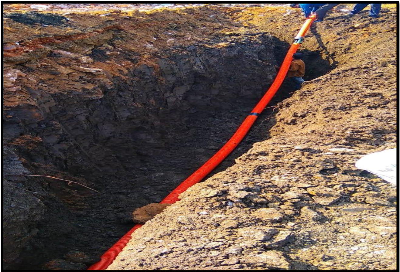
Signal Cable Shifting in Presence of Railway Representatives at RUB Ch 33+585
