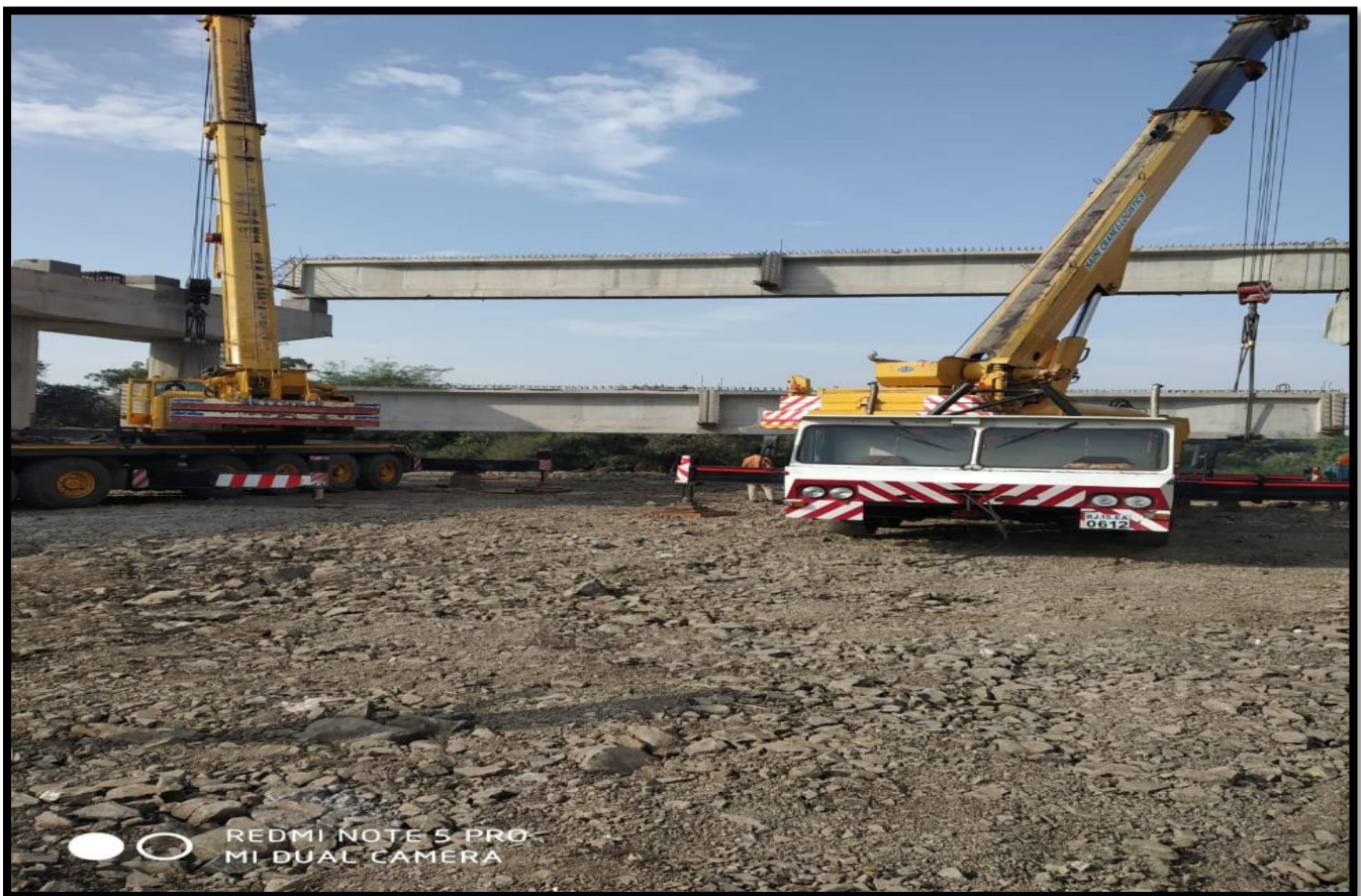
Girder Erection from P-16 to P-17 at Elevated Highway Ch.47+830
