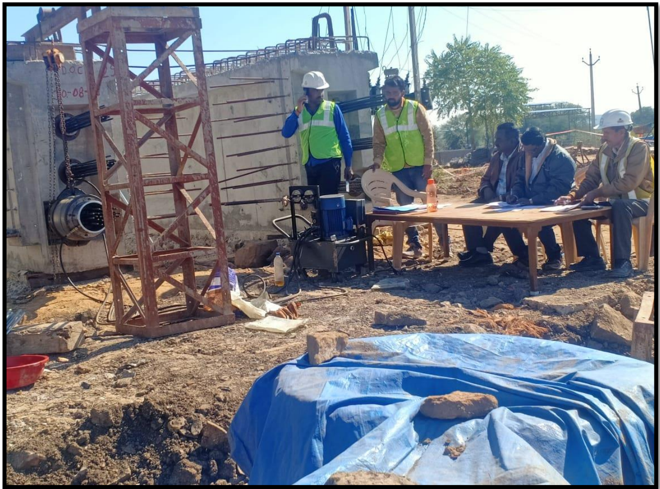
Prestressing of Girder No-29 of MJB Ch 57+127
