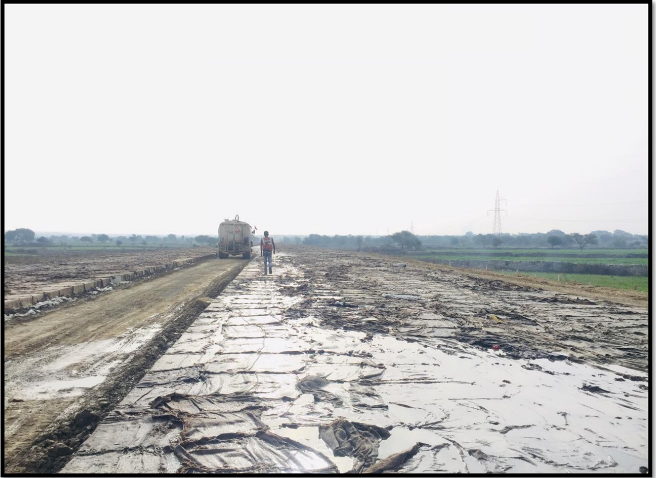
Curing of PQC at Ch 31+200
