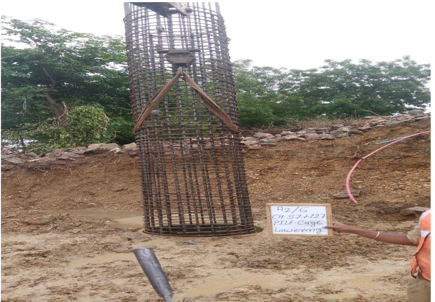
Pile Cage Lowering at MJB 57+127
