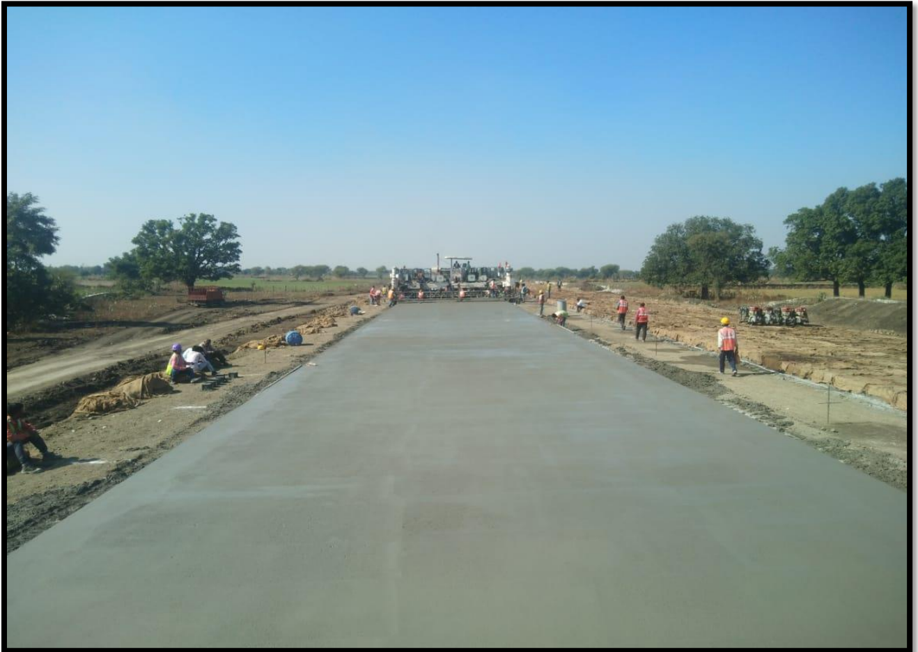
PQC Laying at ch. 9+860 to 10+500 (RHS)
