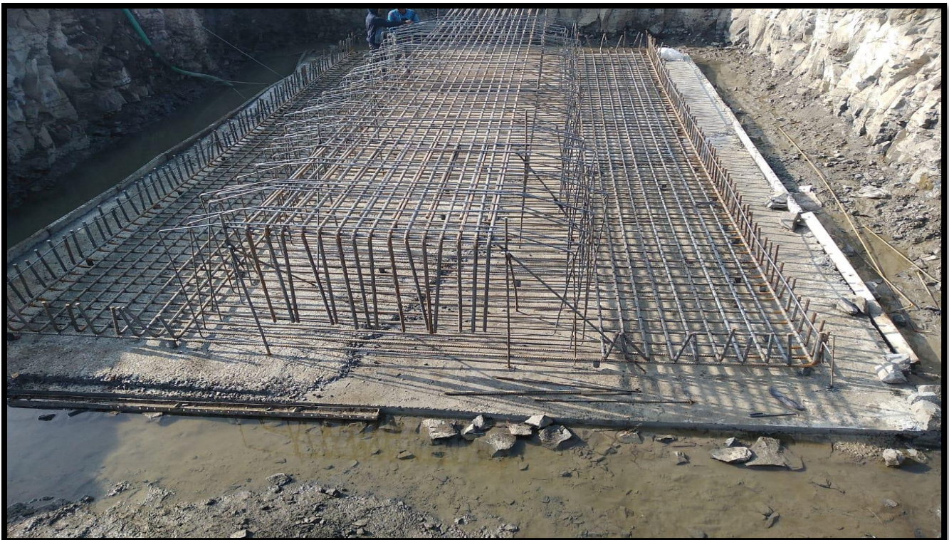
Raft Reinforcement Binding of A-2 (LHS) of ROB at Ch.44+158
