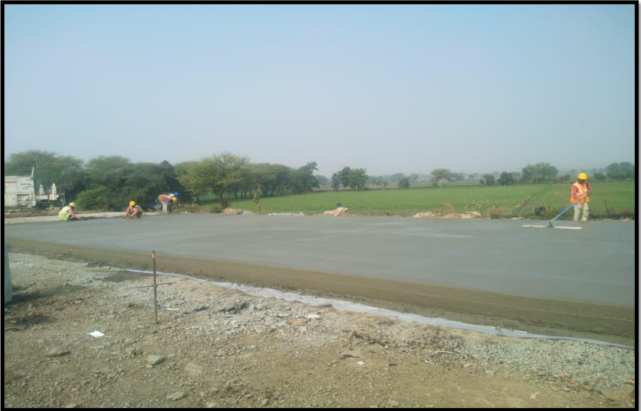
PQC Laying at ch.39+990 to 40+730 (LHS)
