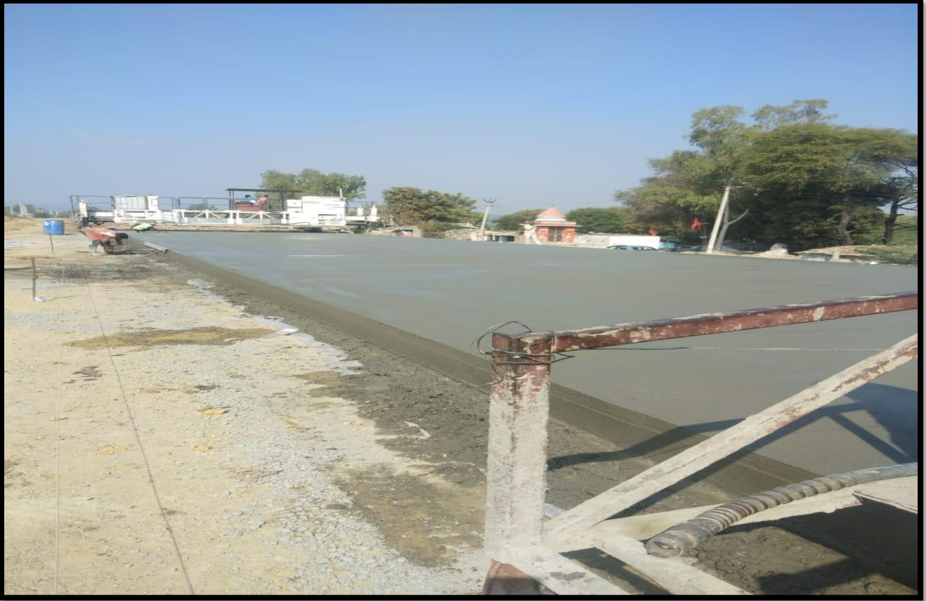
PQC Laying at ch. 9+860 to 10+500 (RHS)
