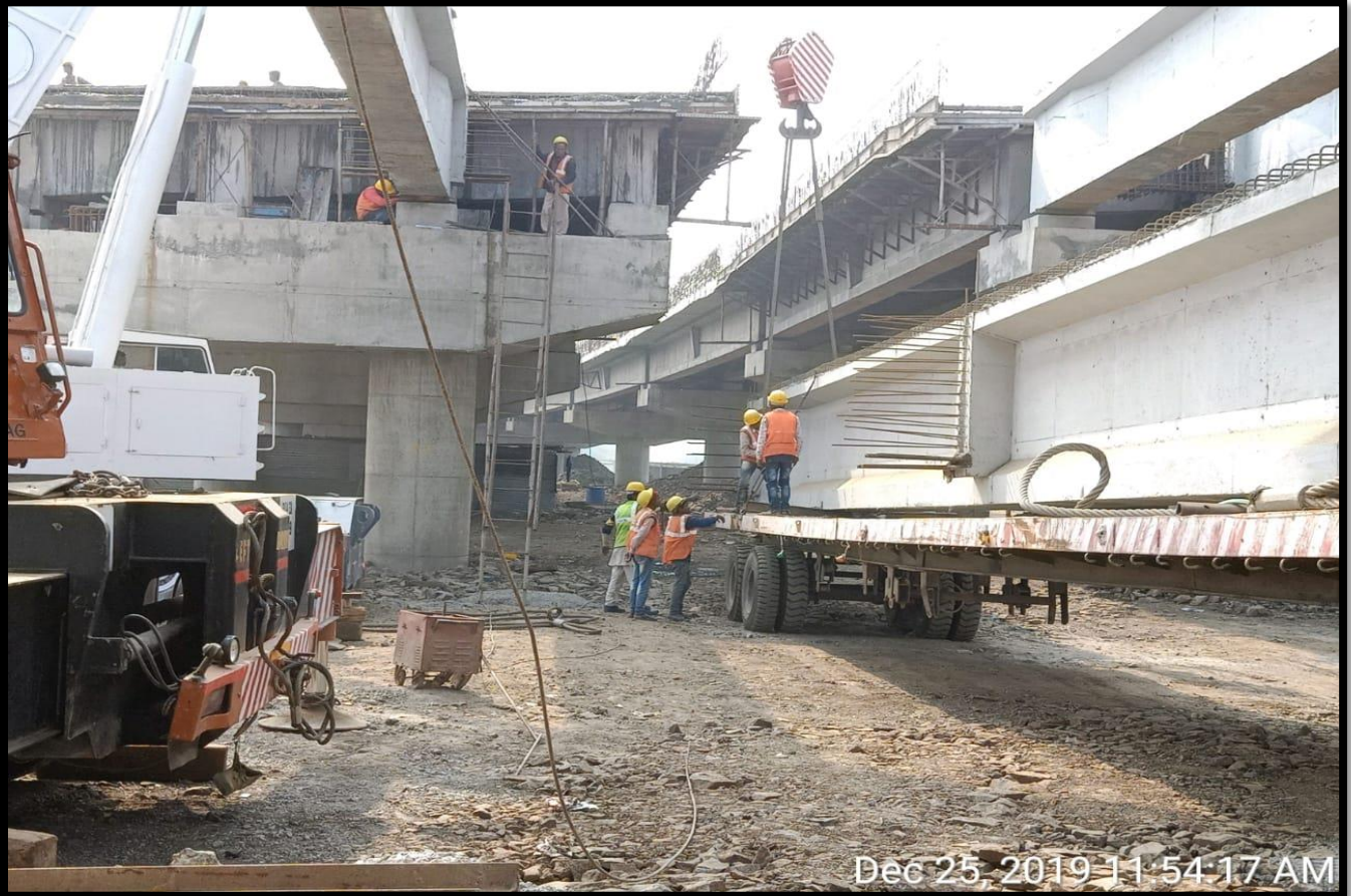
Girder Erection at Elevated Highway Ch.47+830
