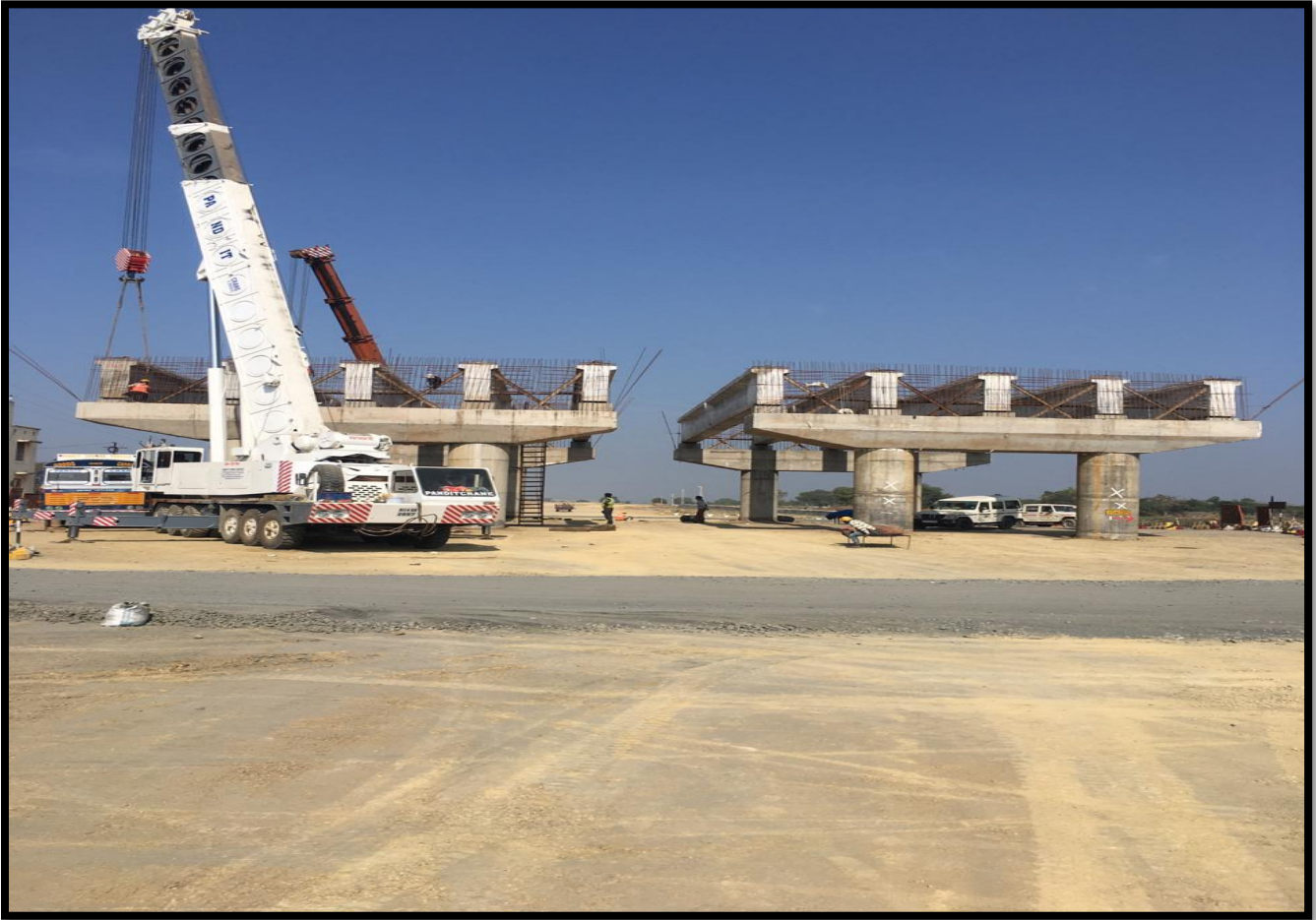
Girder Erection at VUP Ch 15+725
