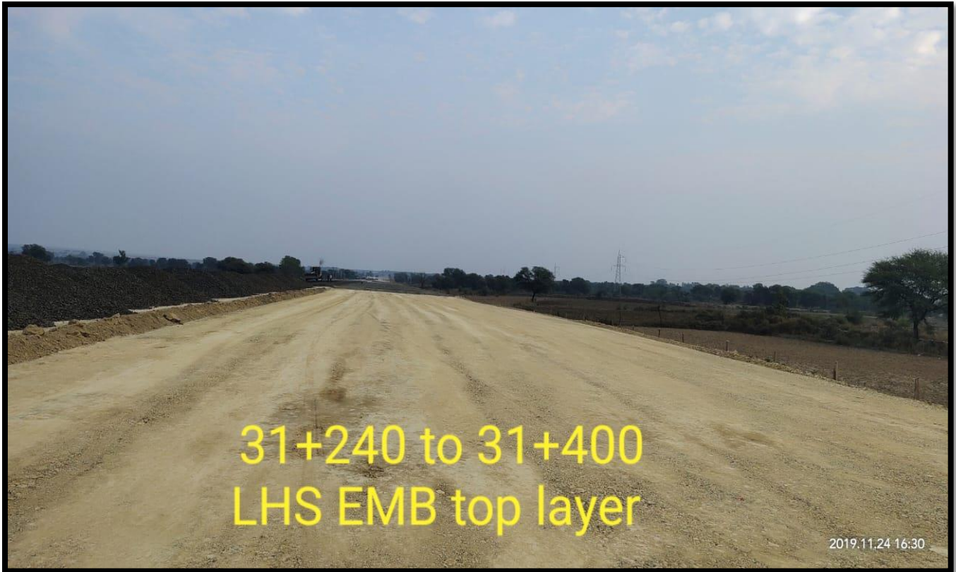
Embankment Top Layer at Ch 31+240 to 31+400 (LHS)
