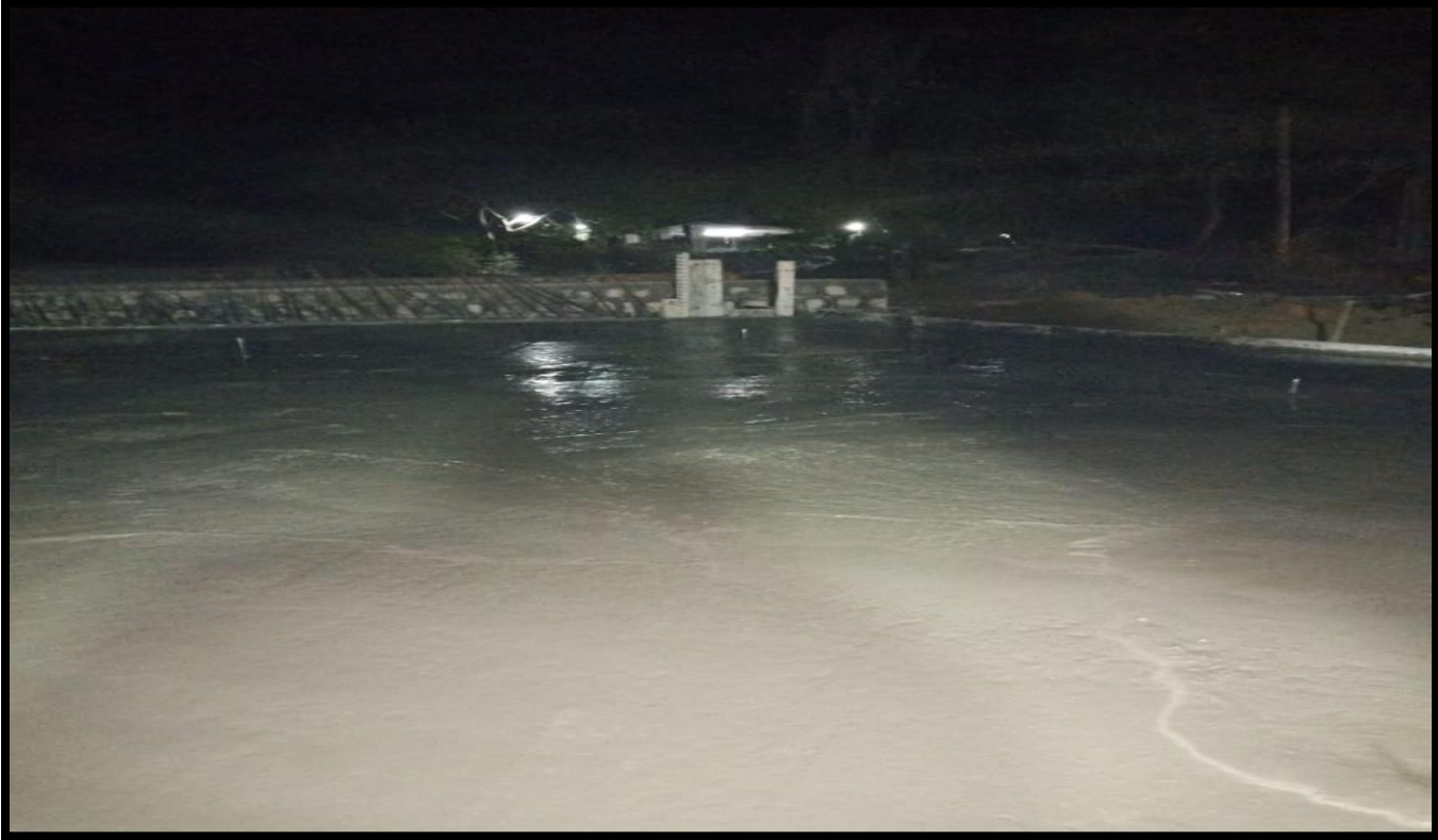
Box Culvert Slab @ Km 24+610
