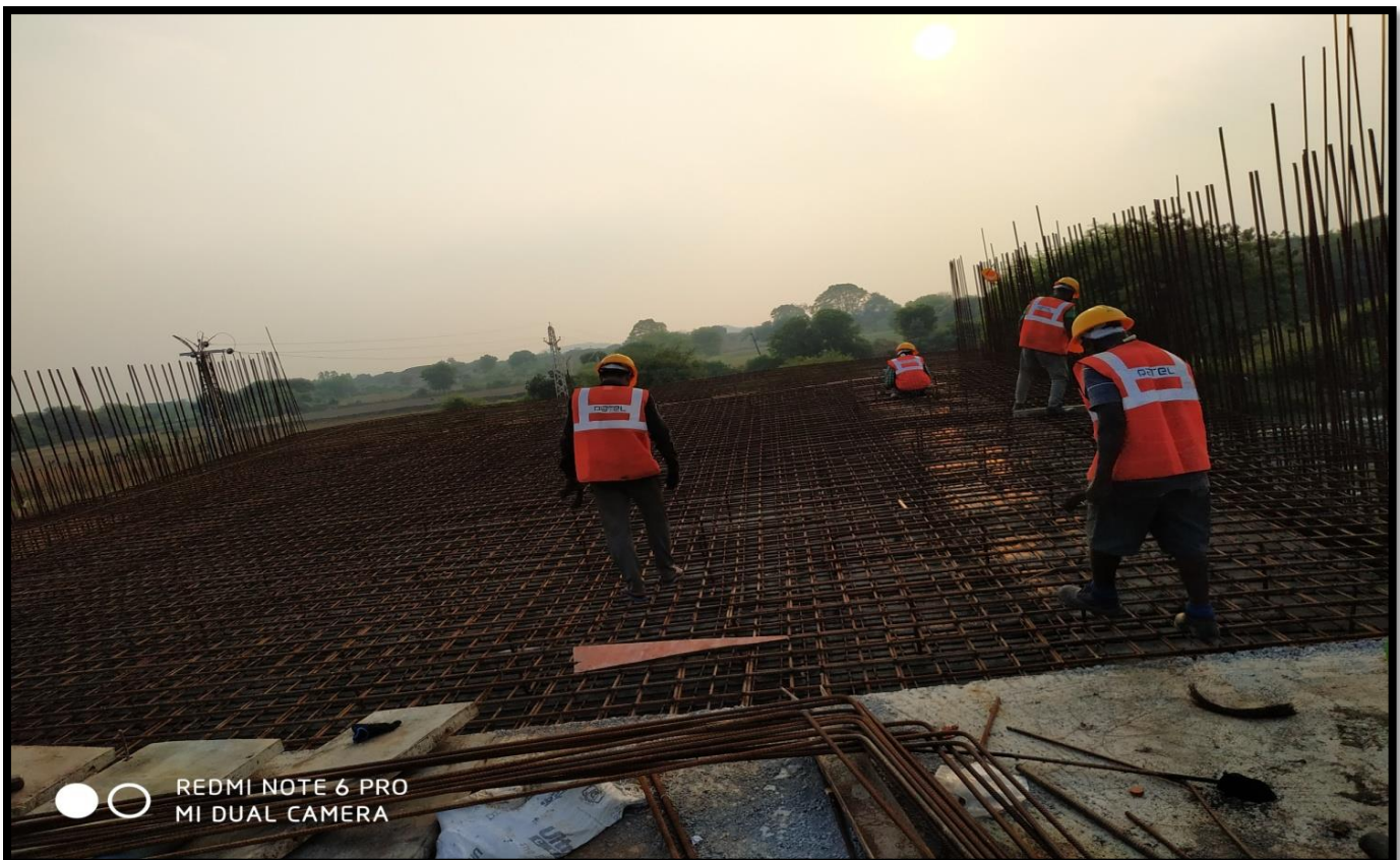
LVUP SLAB REINFORCEMENT AT CH. 21+183 (LHS)
