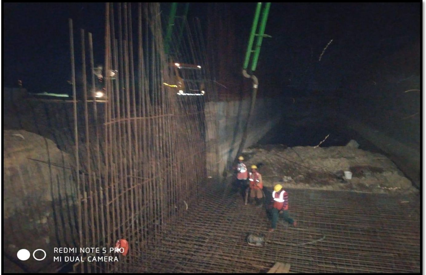
MNB Raft (2-Cell) LHS @ Km. 16+060
