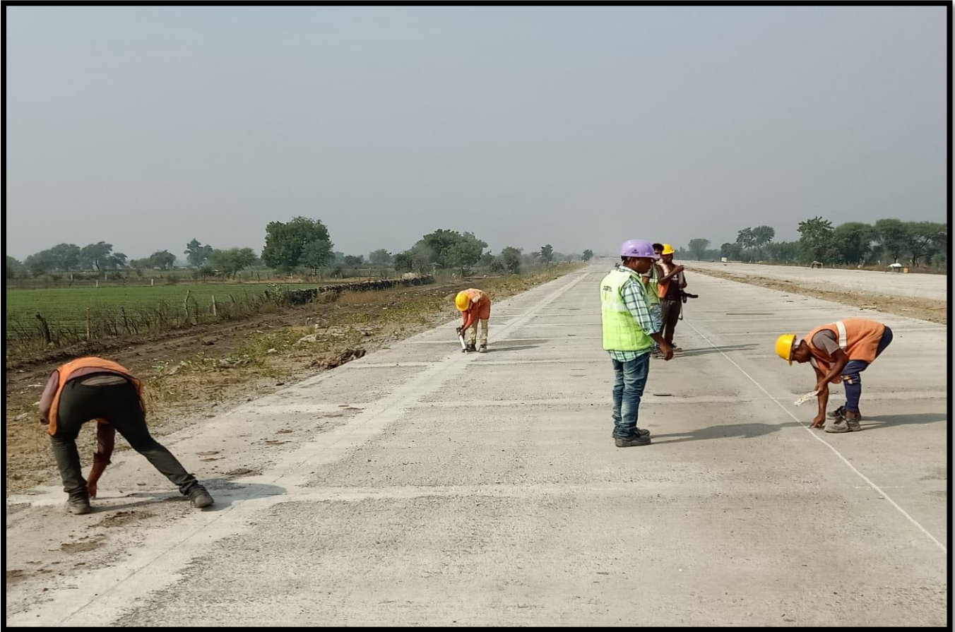
Sealant Filling at ch. 39+160
