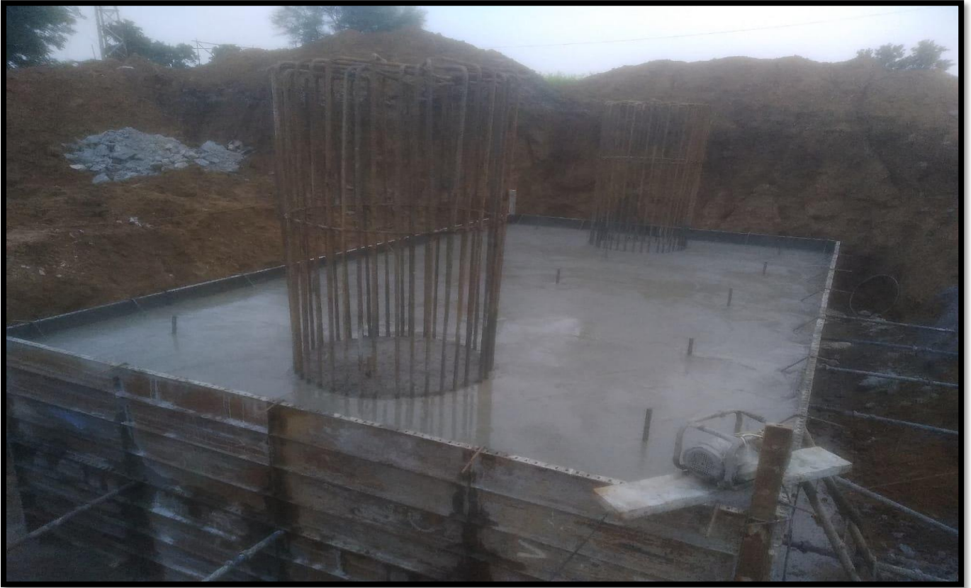
PILE CAP P-11 (LHS) OF MJB @ Km. 36+070
