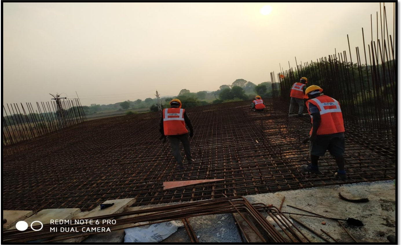
LVUP SLAB REINFORCEMENT AT CH. 21+183 (LHS)
