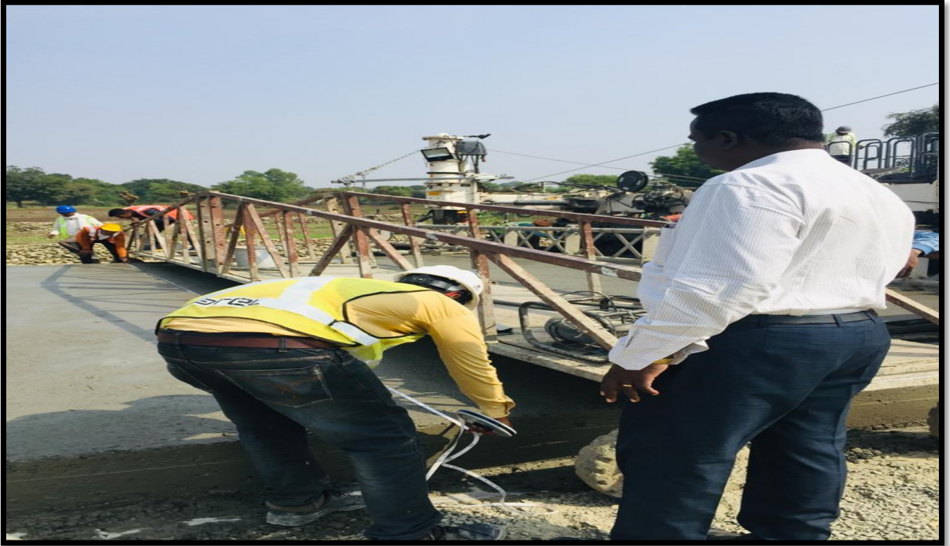
PQC Laying Checking at ch.18+100 to 18+272
