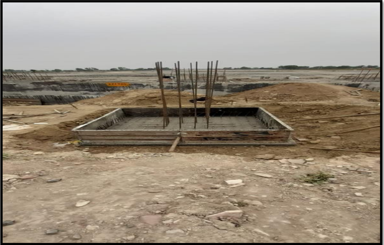
CANOPY FOUNDATION AT TOLL PLAZA@ CH. 27+700
