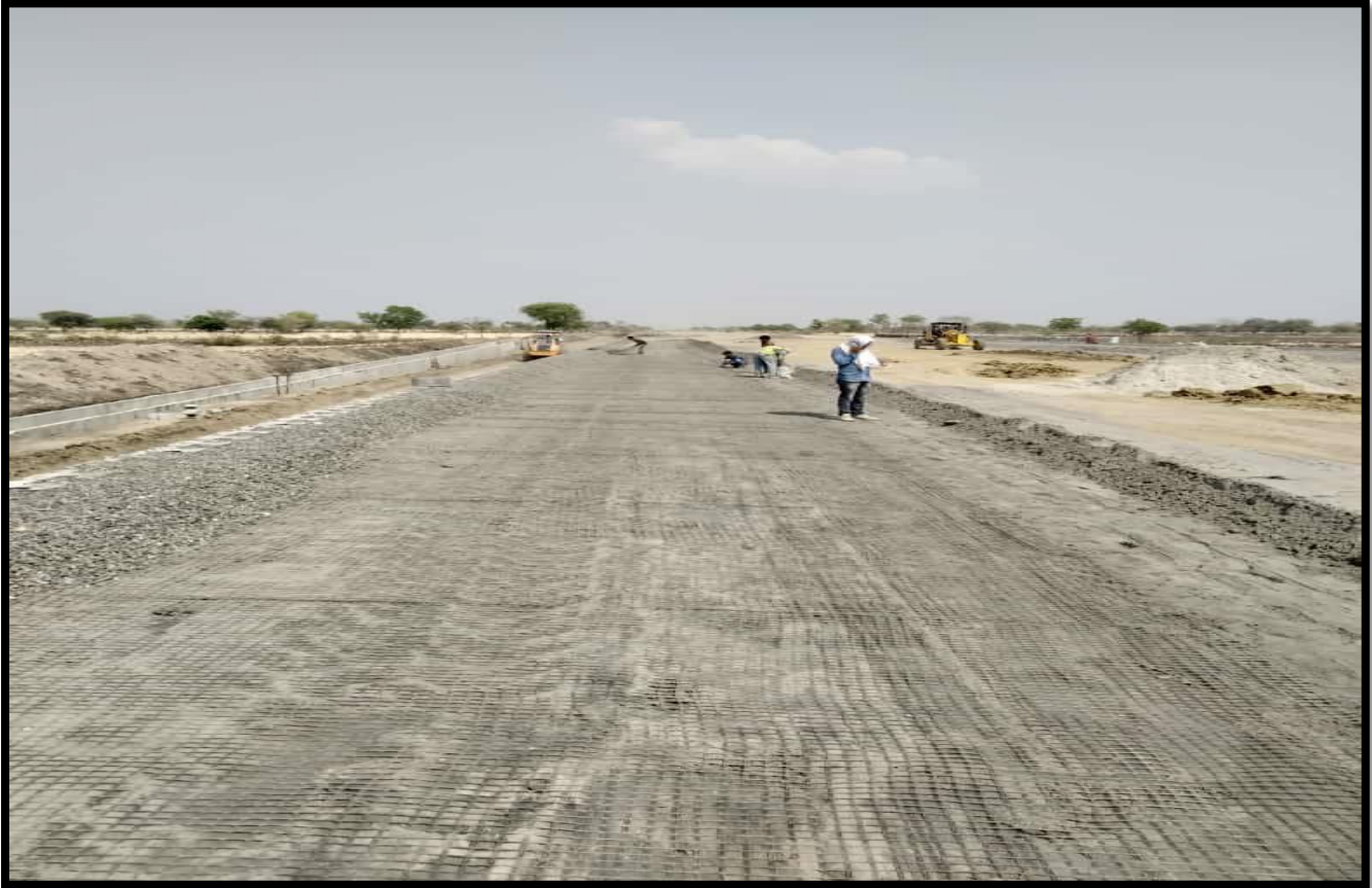
Geogrid Fixing at RE Wall Ch. 41+095
