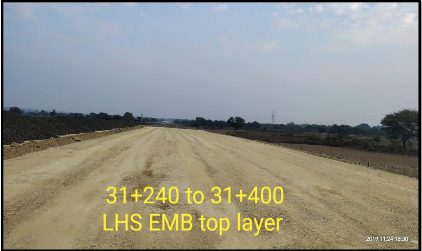
Embankment Top Layer at Ch 31+240 to 31+400 (LHS)
