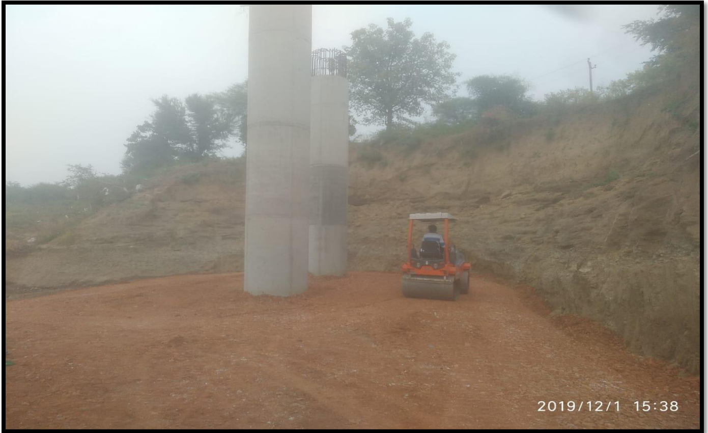
PIER P-9 BED COMPACTION FOR PIER CAP AT CH 36+070 MJB
