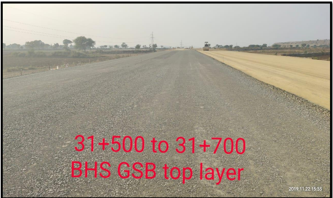
GSB Top Layer at Ch 31+500 to 31+700 (BHS)
