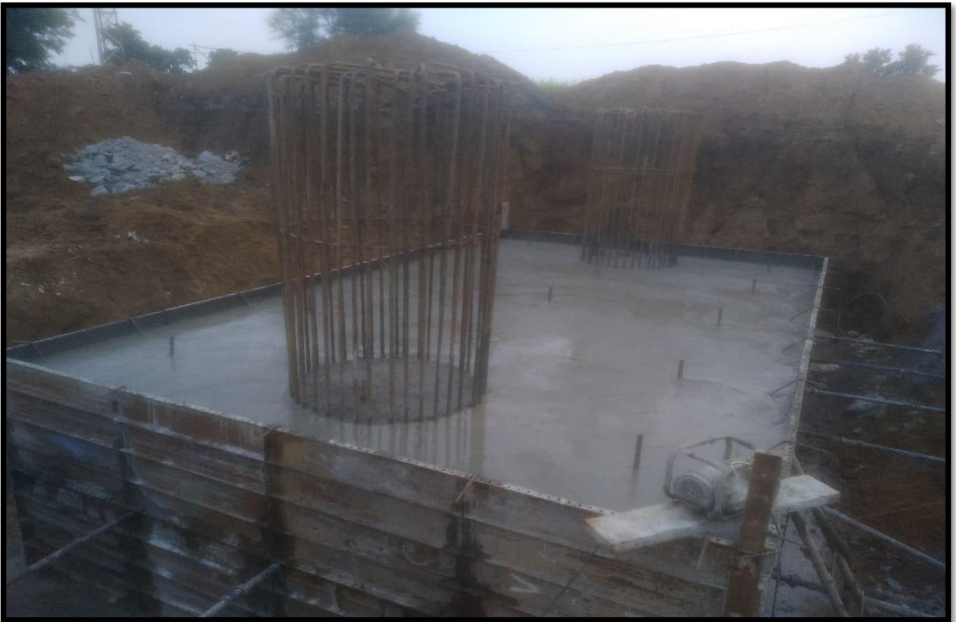
PILE CAP P-1 1 (LHS) OF MJB @ KM. 36+070
