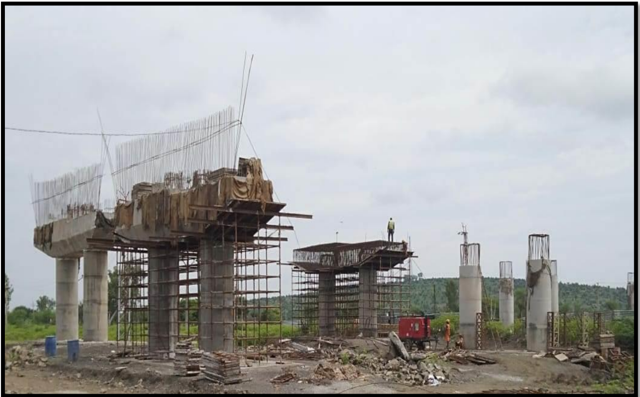
PIER CAP OF FLYOVER @ CH.50+095
