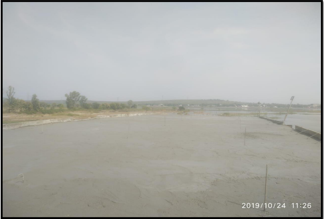
Deck Slab of lvup at ch,45+876
