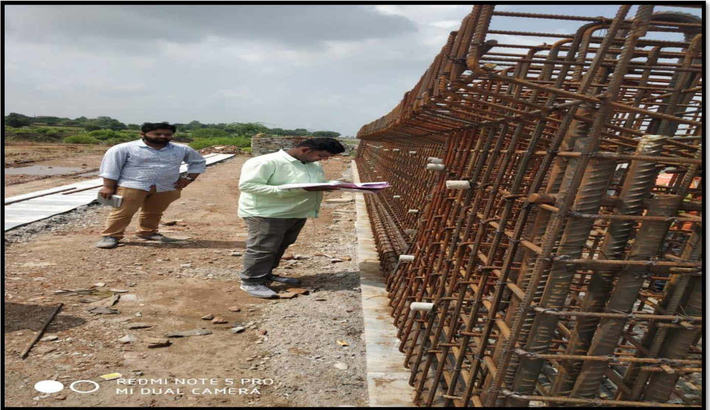
CHECKING OF GIRDER REINFORCEMENT AT CH. 50+095 (FLYOVER)
