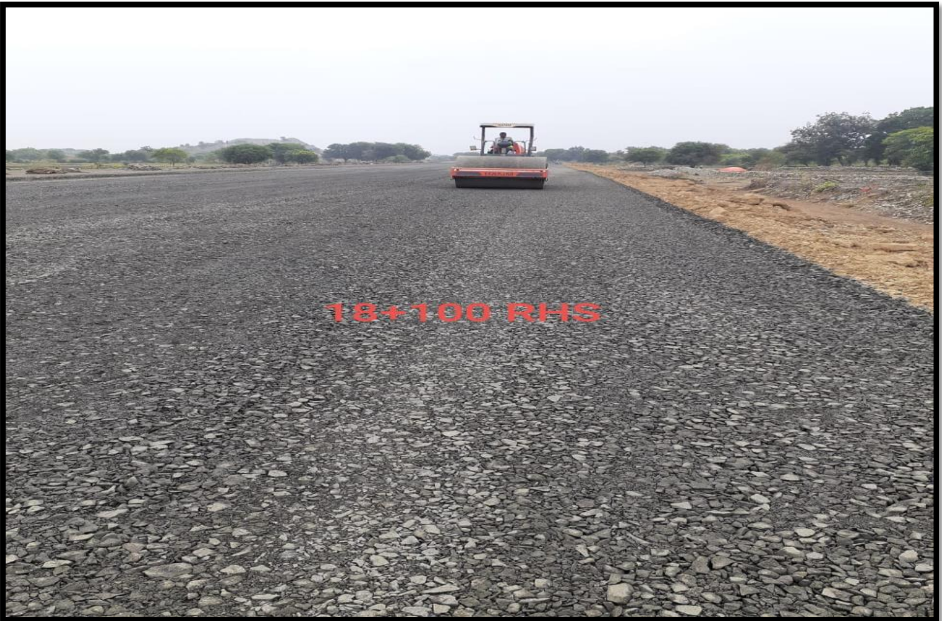
GSB Layer at Ch.18+100 (RHS)
