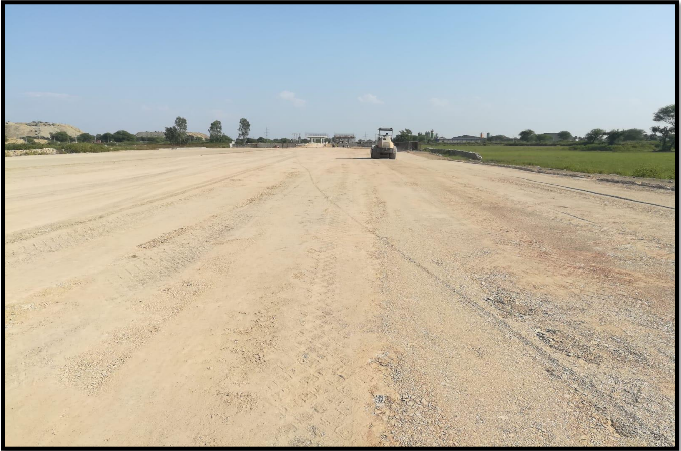
RE Wall Levelling Pad and Service Road Embankment 4 th layer at Ch 29+670 to 29+900 (RHS)
