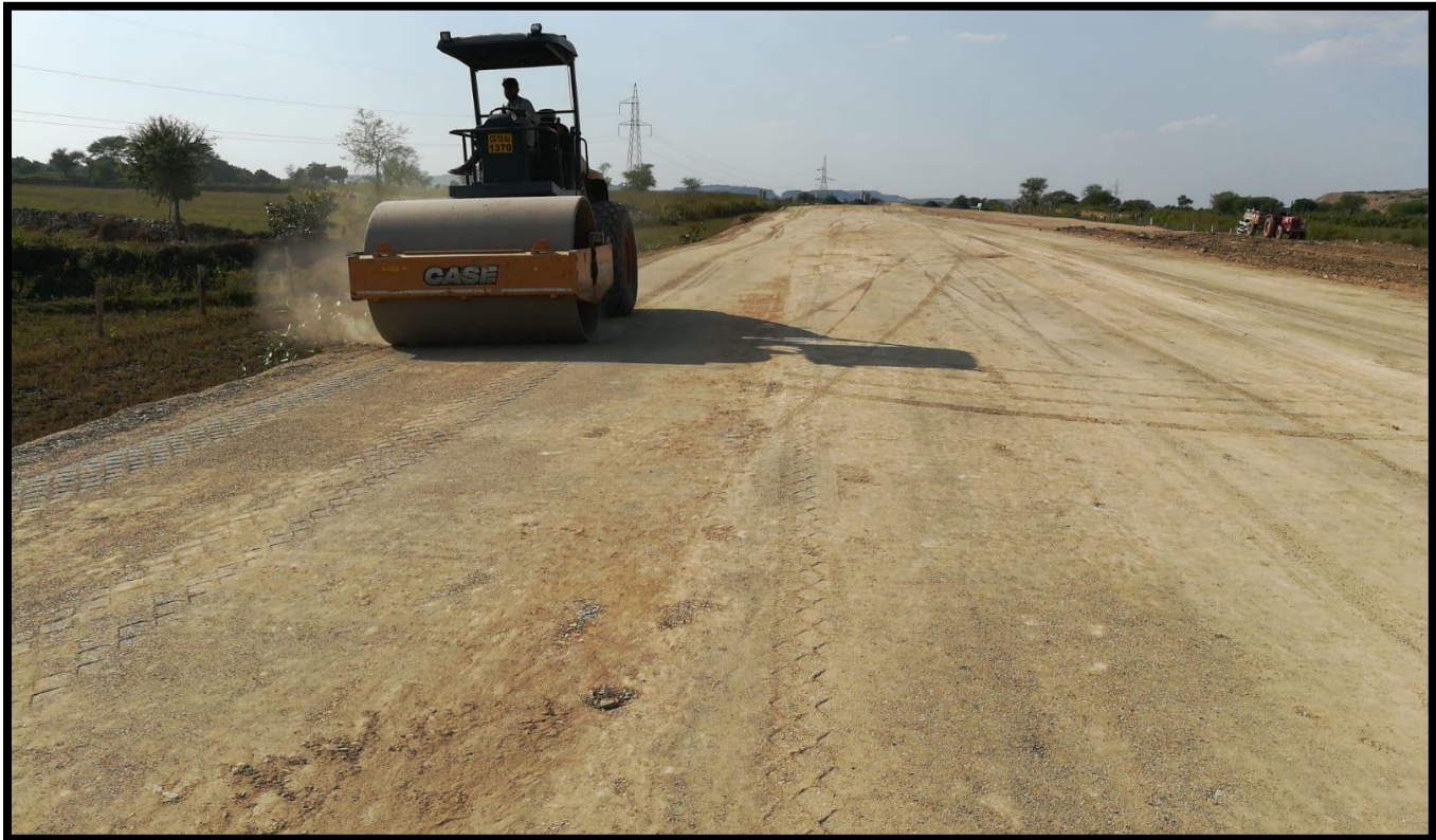
RE Wall Levelling Pad and Service Road Embankment 4 th layer at Ch 29+670 to 29+900 (RHS)
