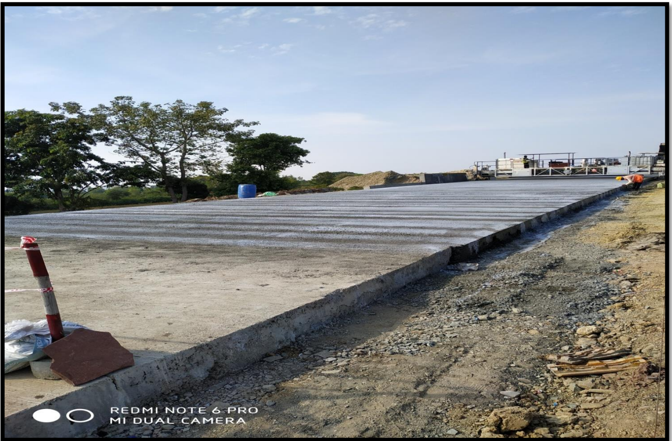
PQC Laying at ch.27+800
