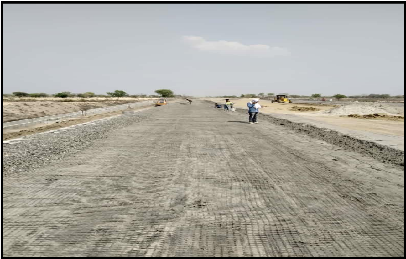
Geogrid Fixing at RE Wall Ch. 41+095
