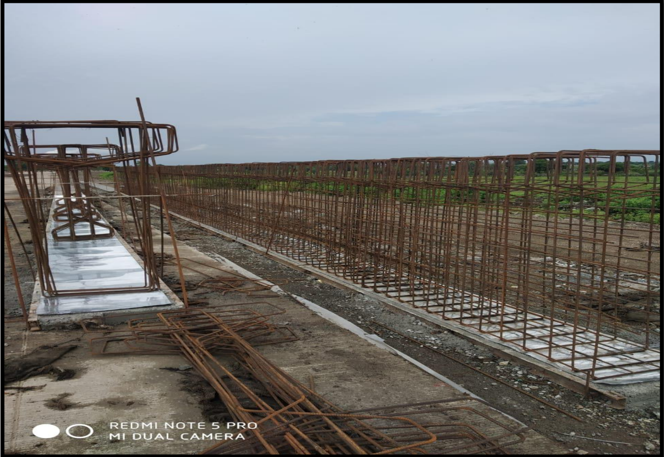
GIRDER REINFORCEMENT WORK AT CH.49+330 (VUP)
