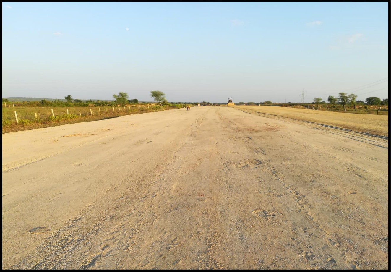
Embankment Layer at Ch. 31+240 to 31+500
