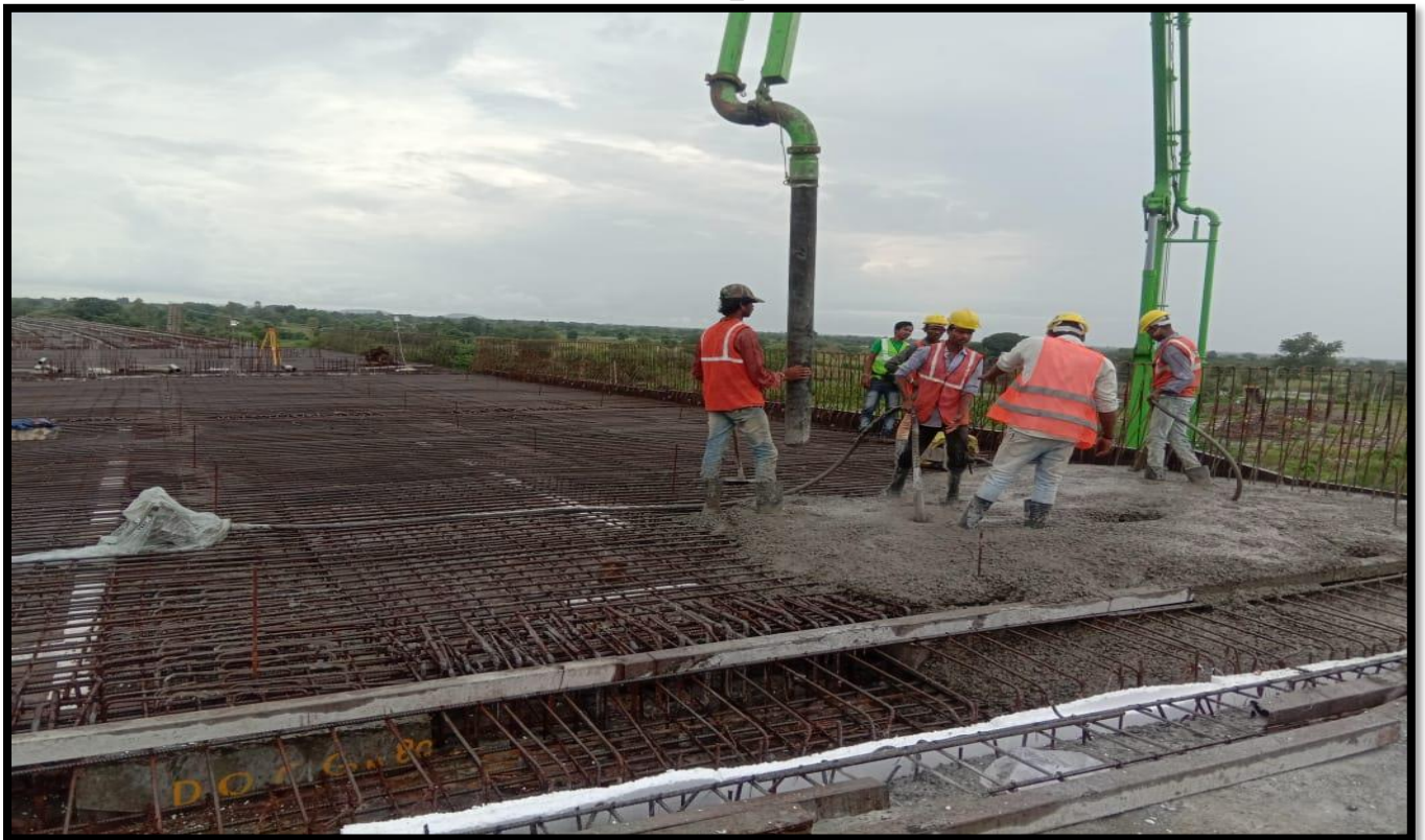
Deck Slab P-9 to P-10 (RHS) (elevated highway) ch.47+830
