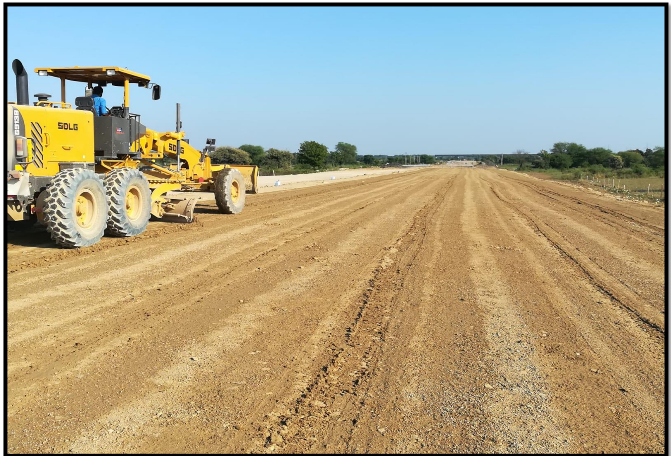
Subgrade 1st Layer at Ch. 31+500 to 31+700 (RHS)
