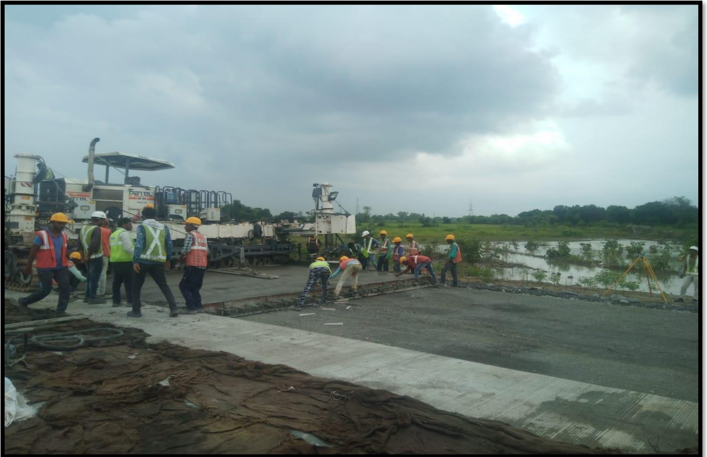
LAYING WORK OF PQC AT TOLL PLAZA
