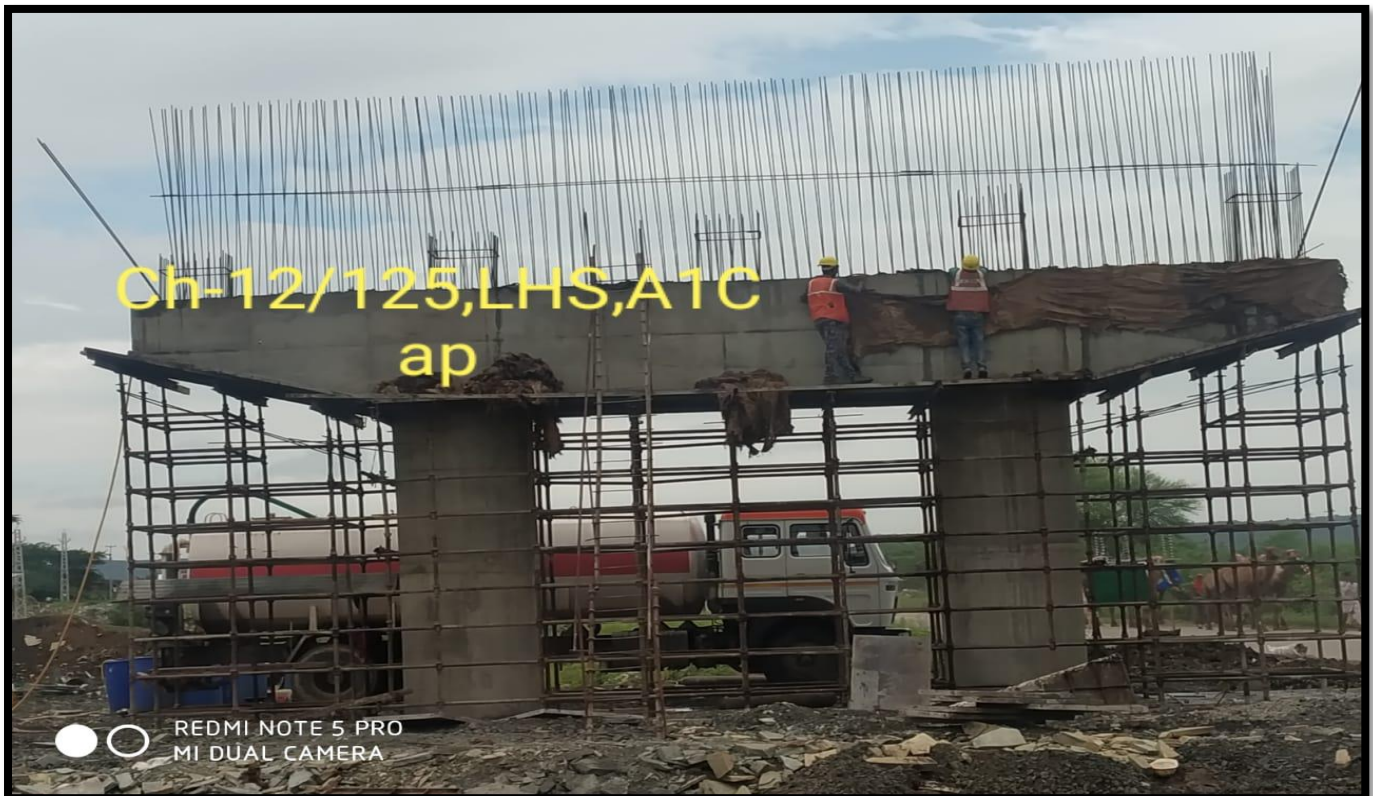
A-1 PIER CAP (LHS) OF VUP @ CH. 12+ 125
