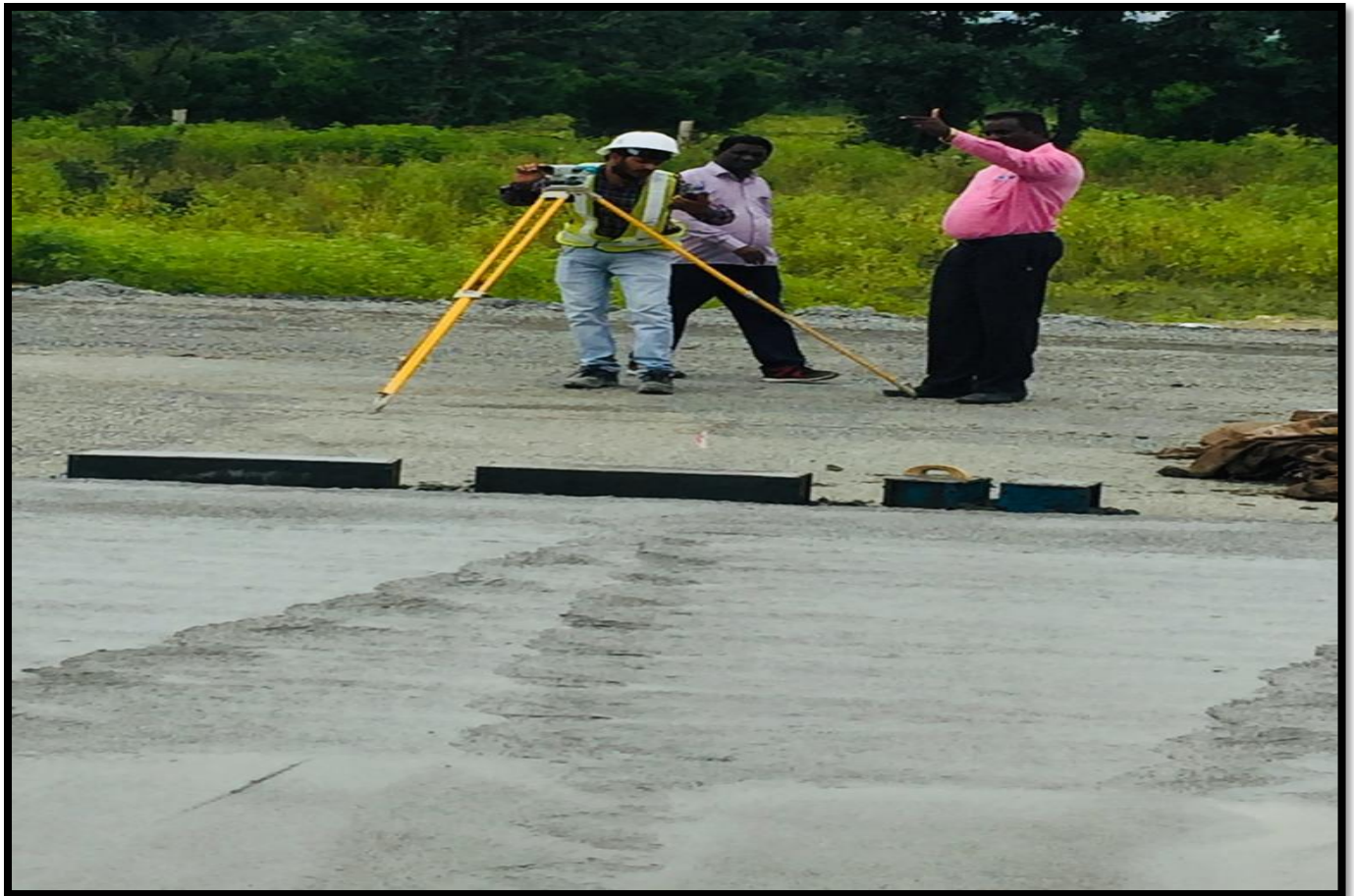
CHECKING OF PAQC LAYING BY IE REPRESENTATIVE
