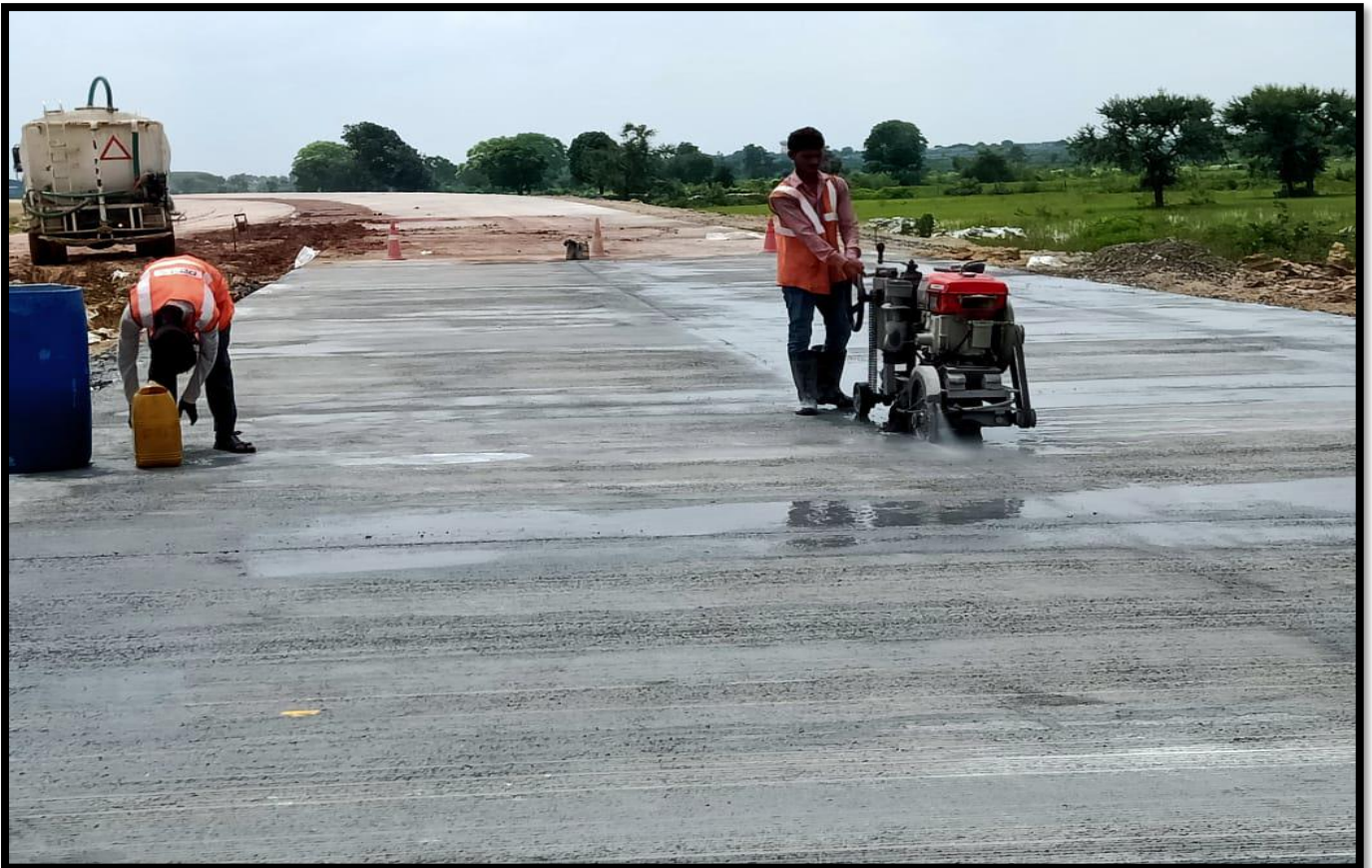
CUTTING WORK OF PQC
