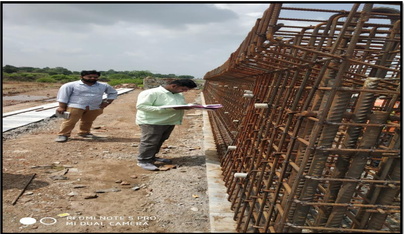
CHECKING OF GIRDER REINFORCEMENT AT CH. 50+095 (FLYOVER)
