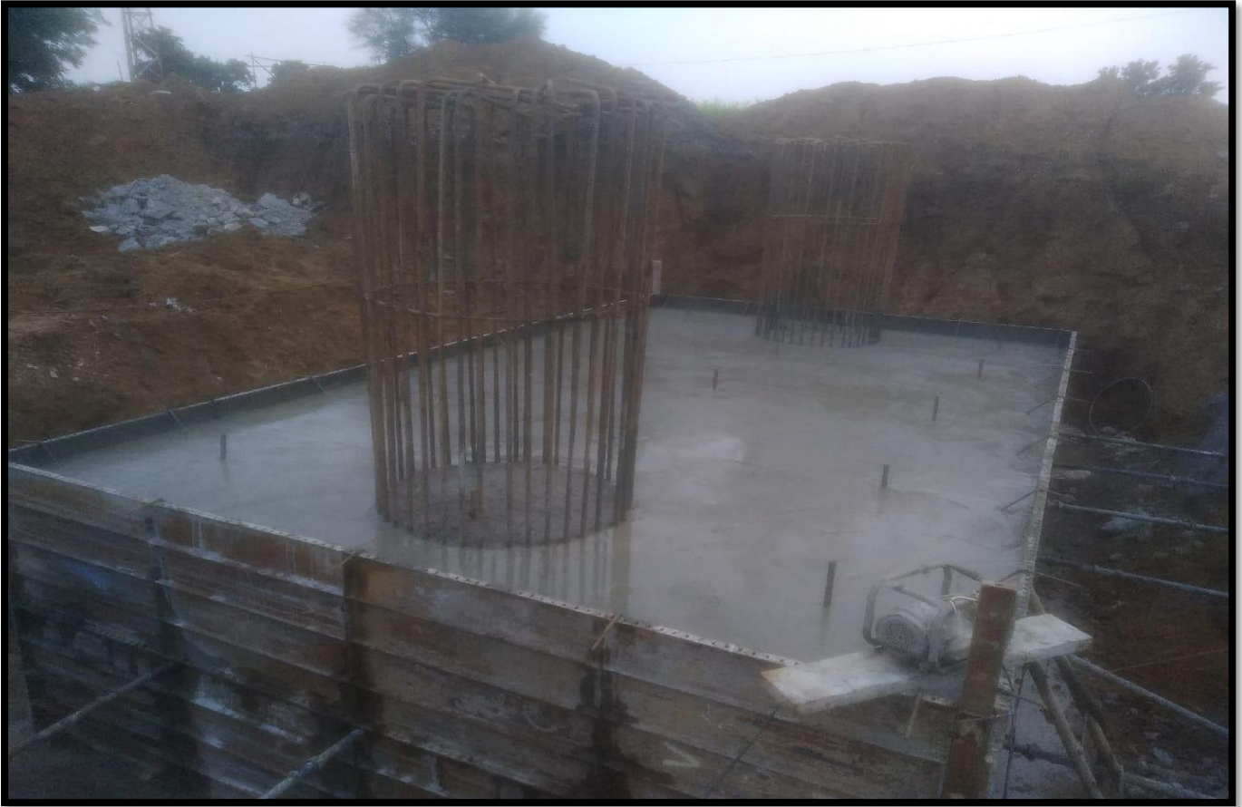
PILE CAP P-11 (LHS) OF MJB @ Km. 36+070
