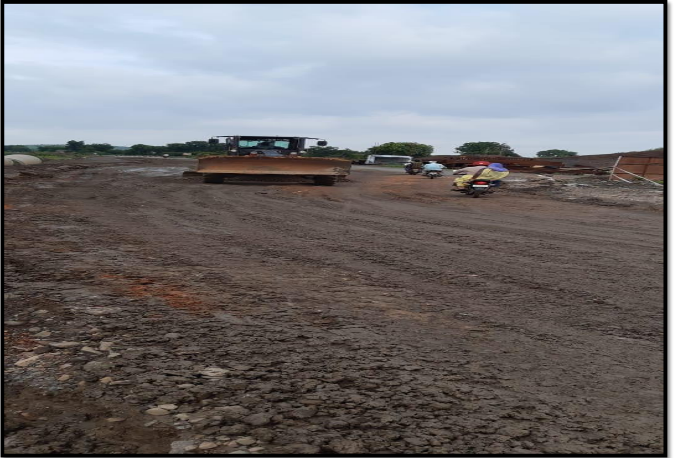
DIVERSION WORK@ CH:50+095
