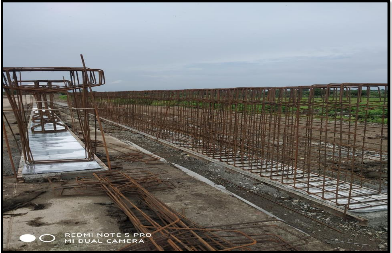
GIRDER REINFORCEMENT WORK AT CH.49+330 (VUP)
