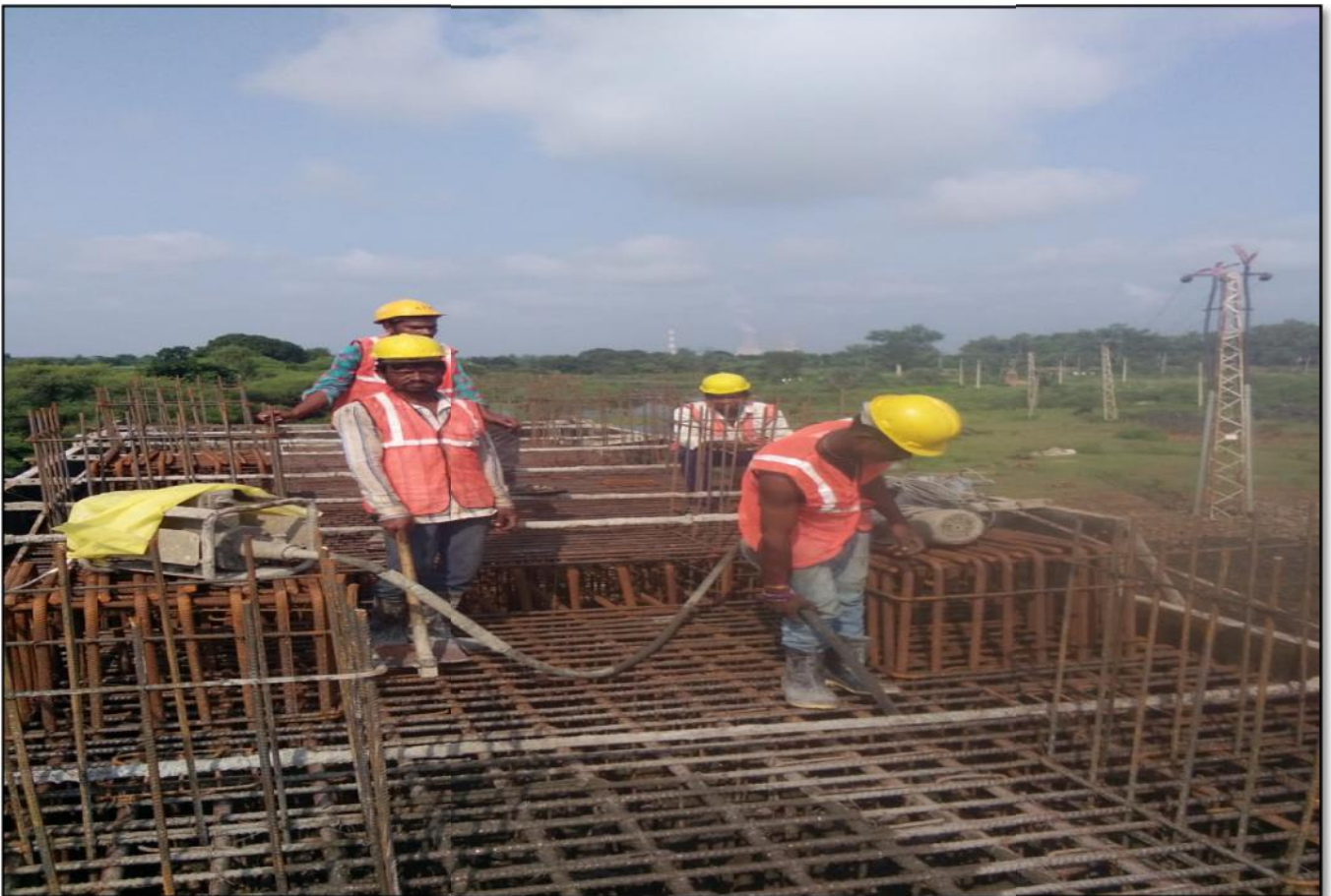
CASTING OF PIER CAP P16 RHS @ KM. 47+830
