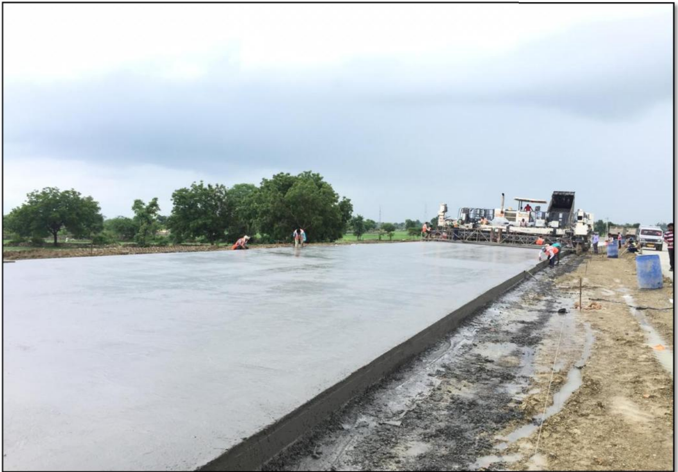
LAYING WORK OF PQC
