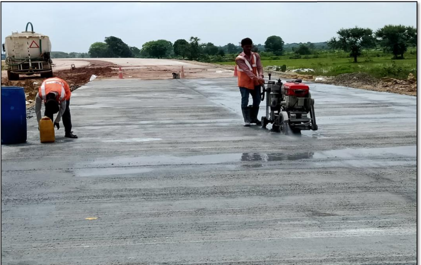
CUTTING WORK OF PQC
