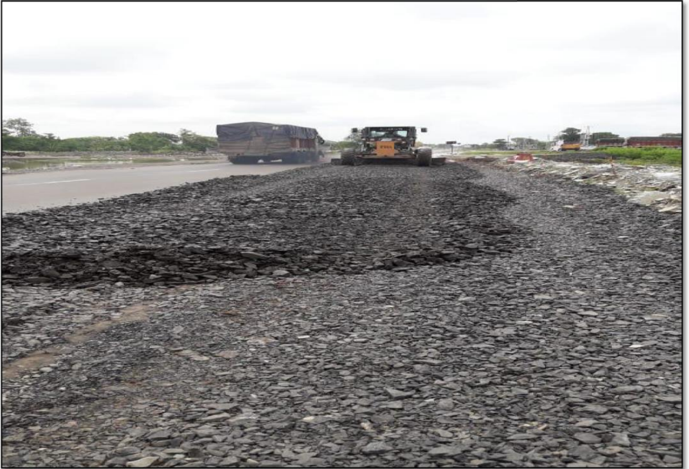
DIVERSION REPAIRING WORK @ CH: 23+675
