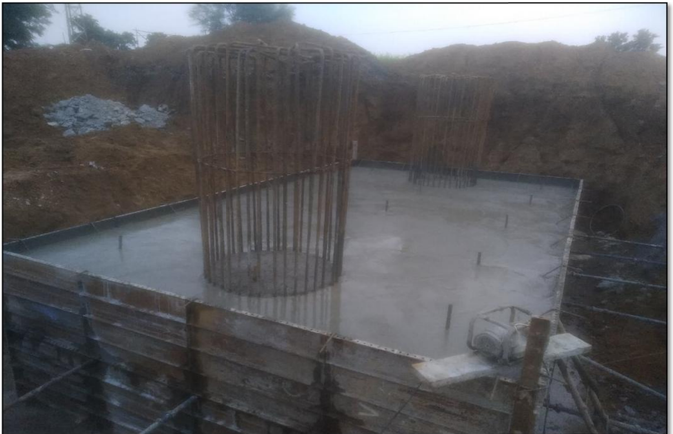
PILE CAP P-11 (LHS) OF MJB @ Km. 36+070
