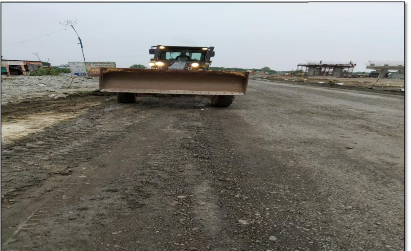
DIVERSION REPAIRING WORK @ CH: 25+ 100
