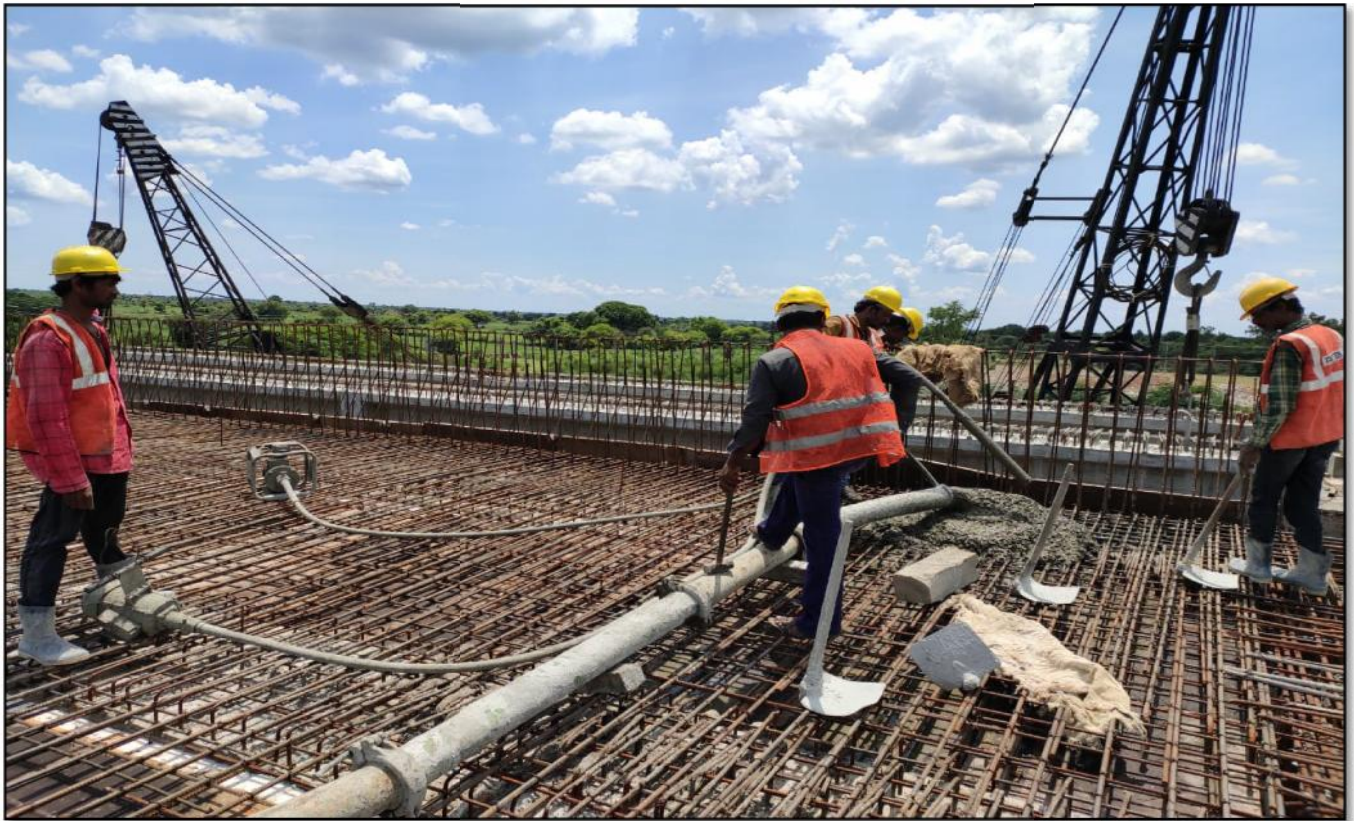
SLAB CASTING OF ELEVATED @ KM.47+830
