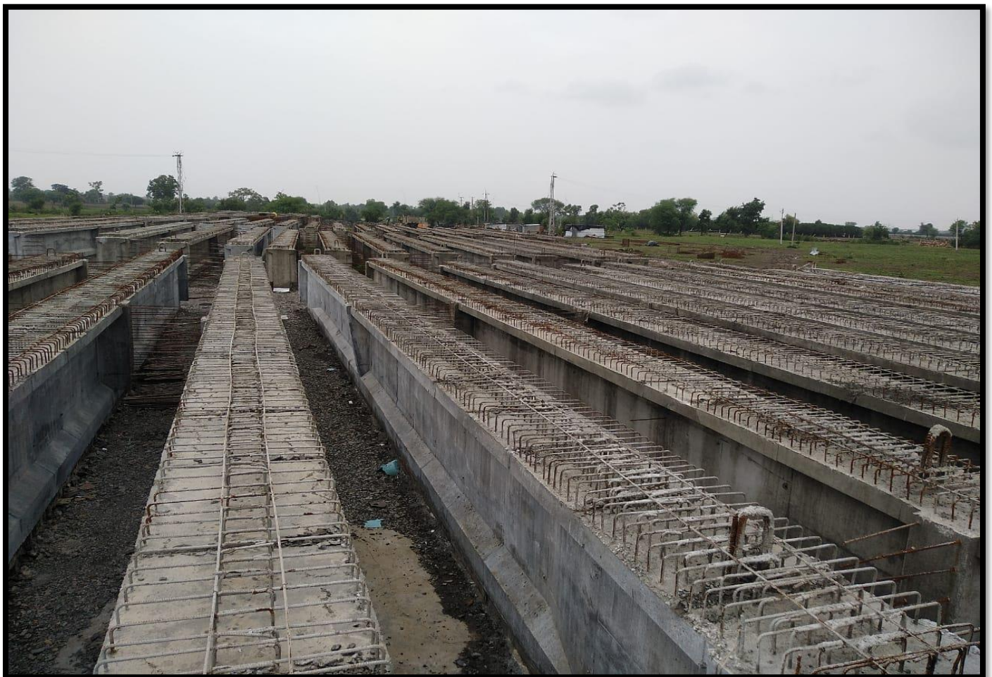
Girder casting @ Ch.36+070(Major Bridge)
