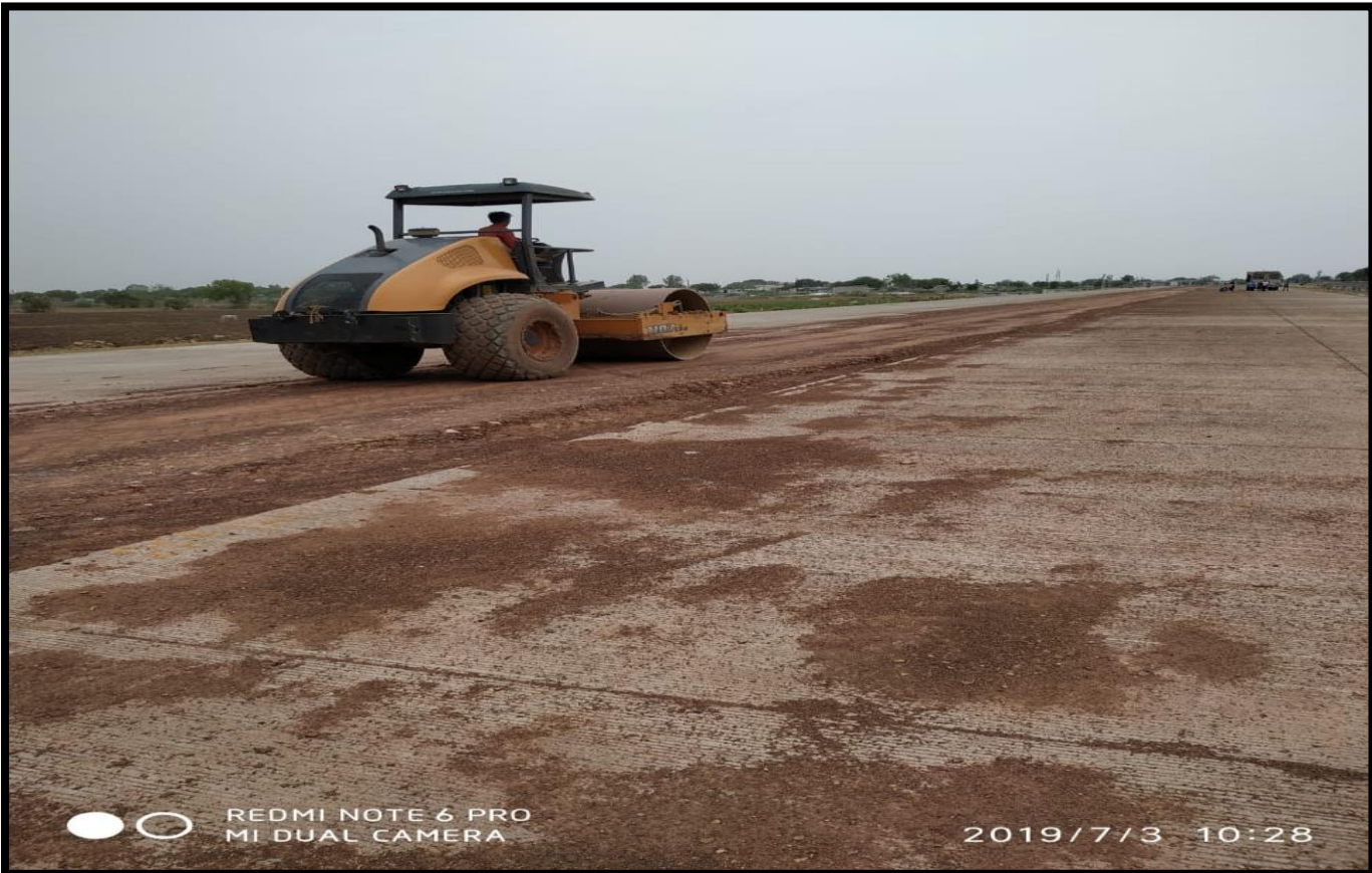
PQC Median Filling at Ch.23+100
