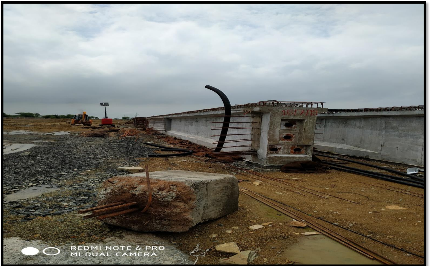
VUP Girder Reinforcement Checking at Ch.30+075
