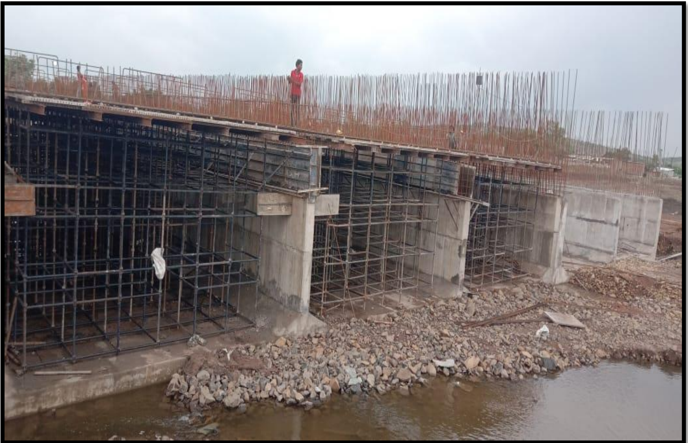
Slab Casting @ Ch. 49+785
