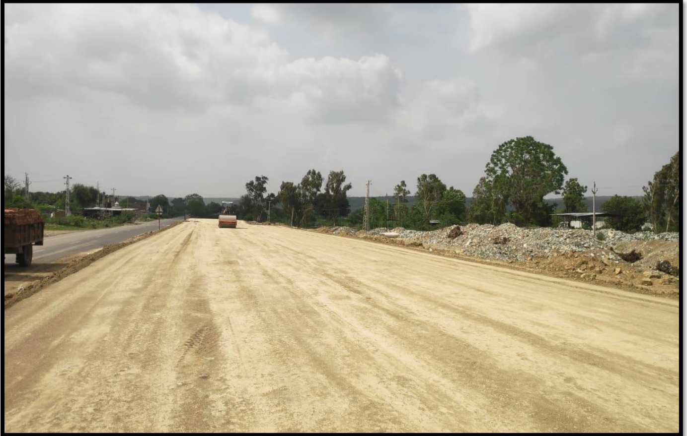
Subgrade Top at Ch.9+960 to 10+150
