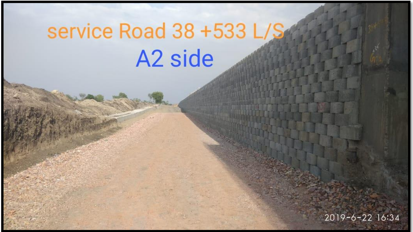
RE Wall Work @ Ch.38+533
