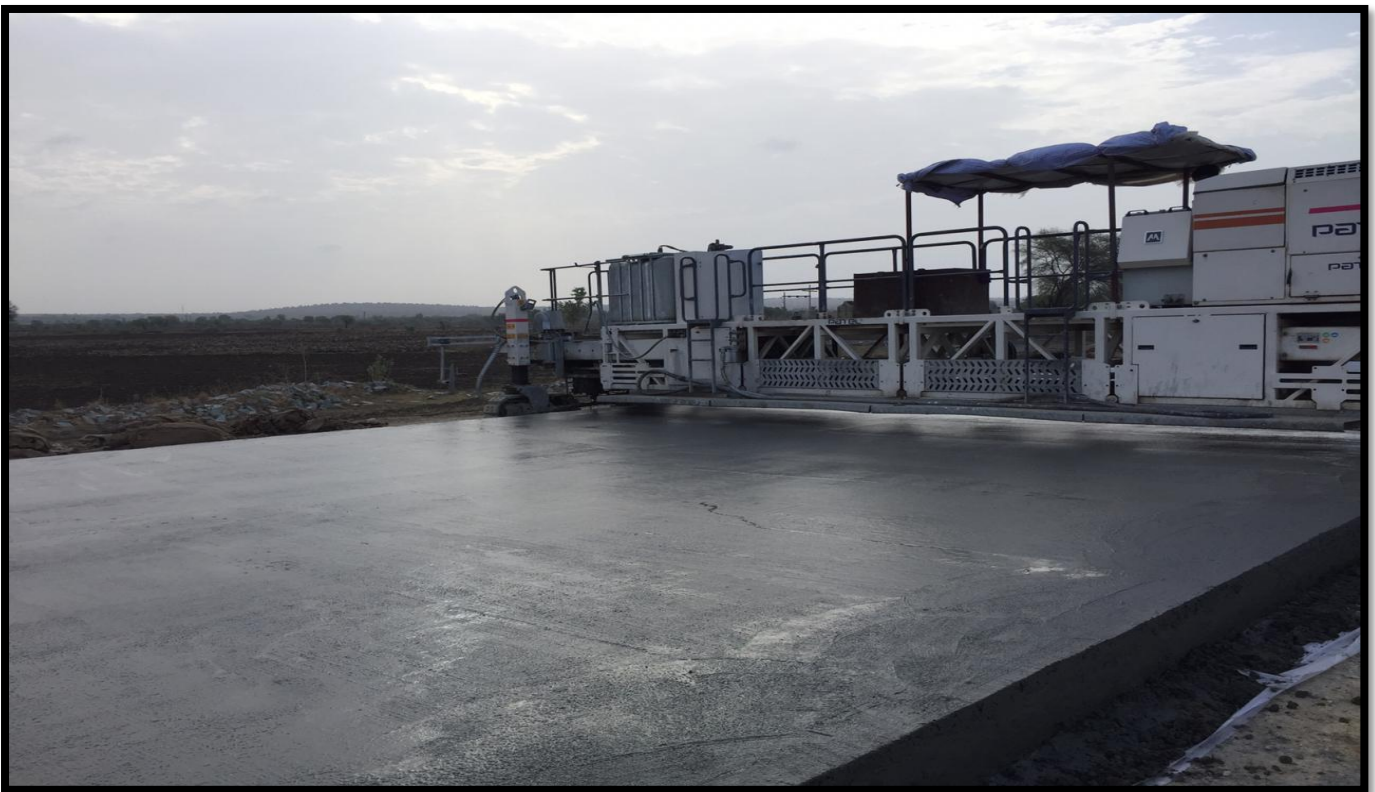
PQC Laying at Ch.25+540 (LHS)
