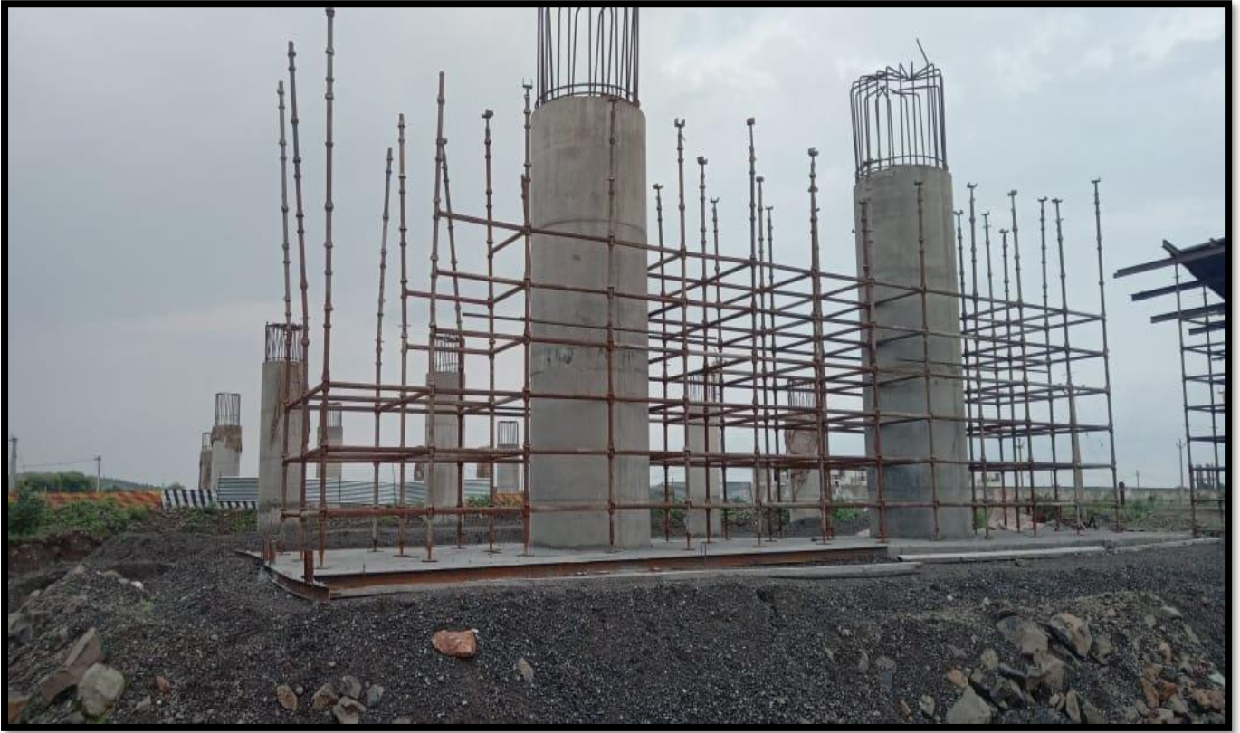
Pier Completion @ Ch.50+095
