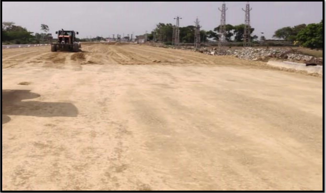
Embankment Top at Ch. 10+400 to 10+650
