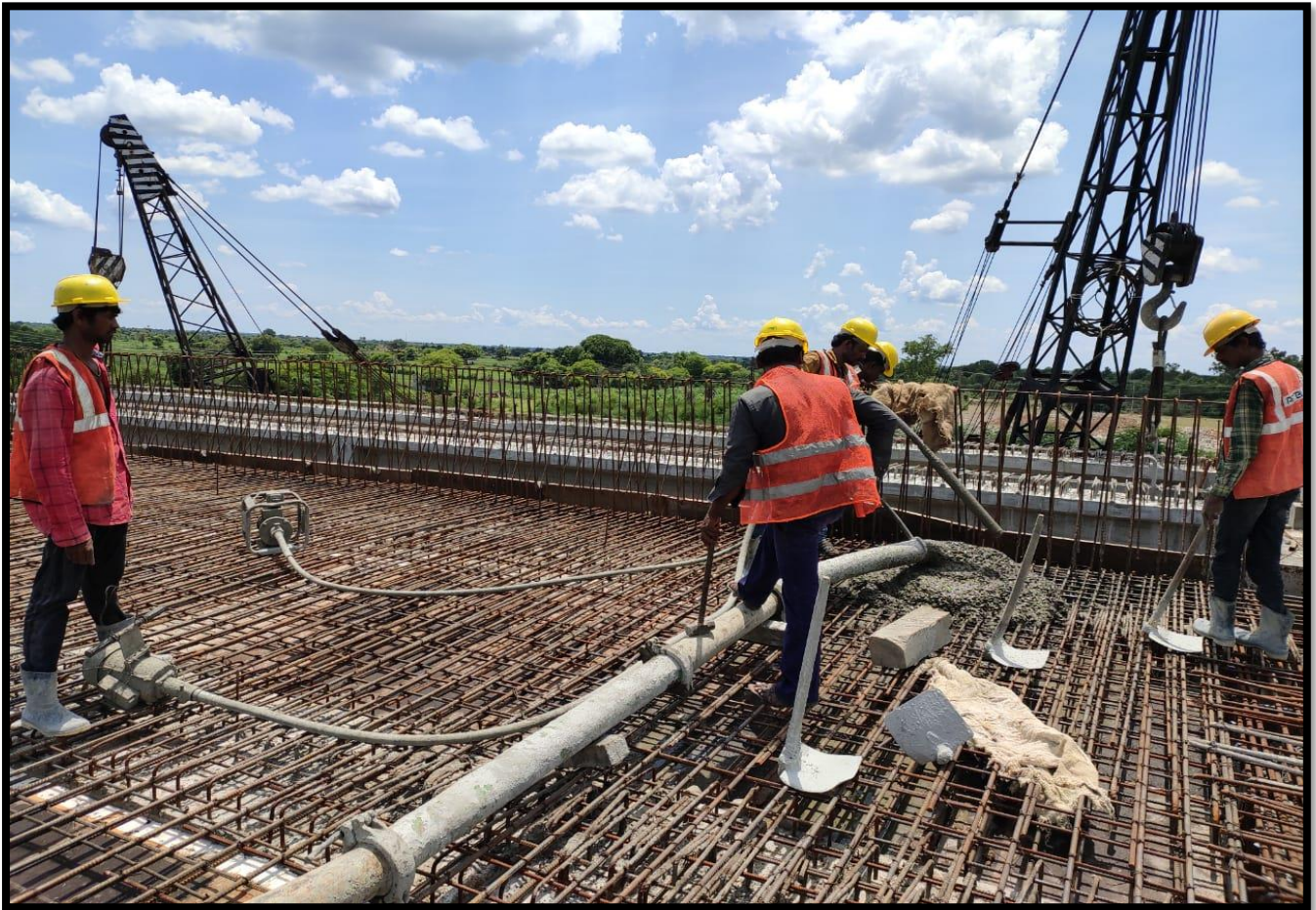
Slab Casting at Elevated Highway @ Ch. 47+830
