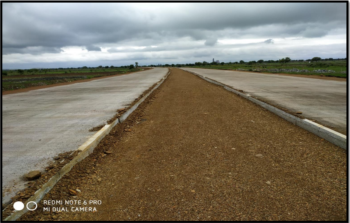
Kerb Laying at Ch. 13+300
