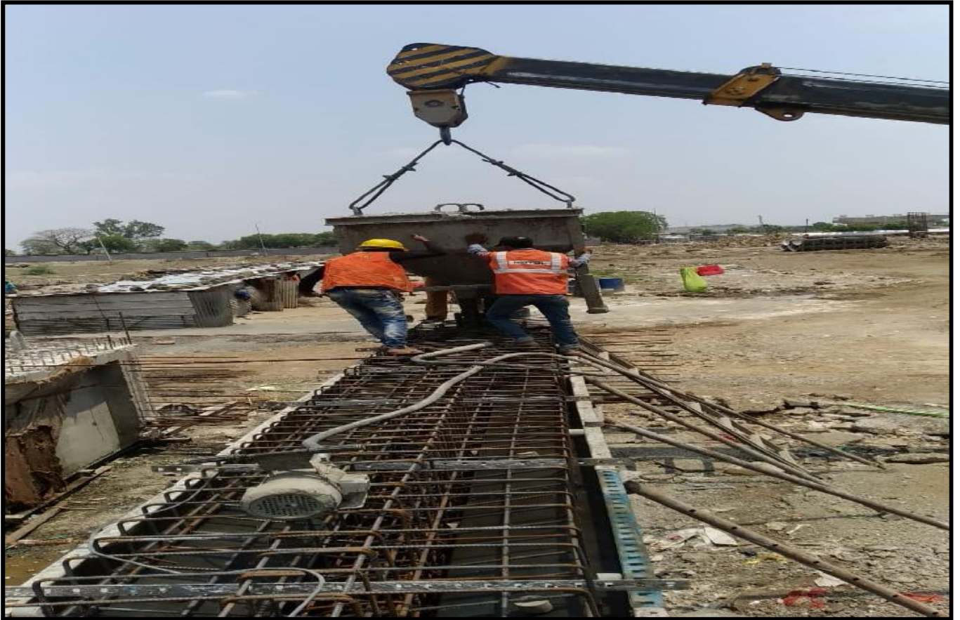
Girder casting @ Ch.47+830 (Elevated Highway)
