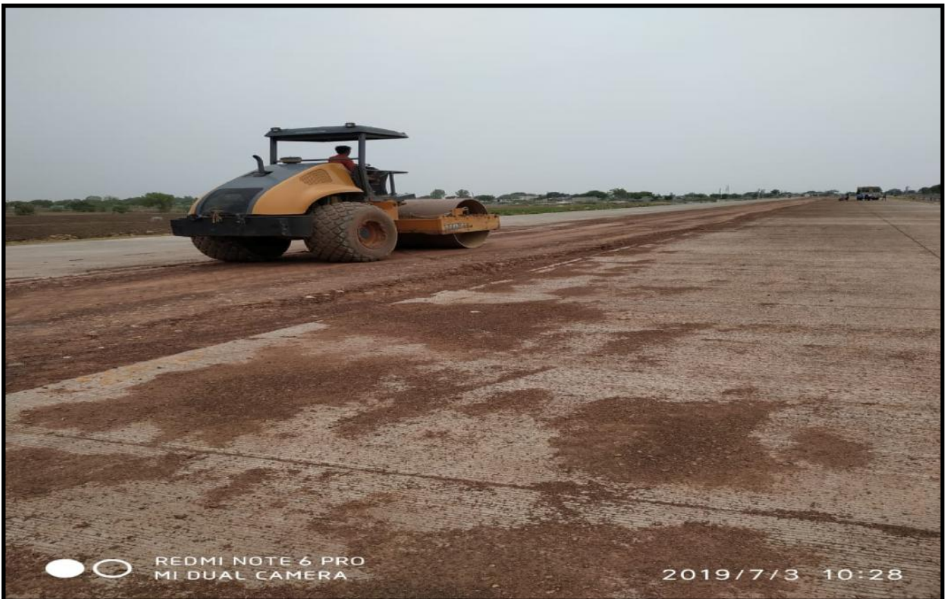
PQC Median Filling at Ch.23+100
