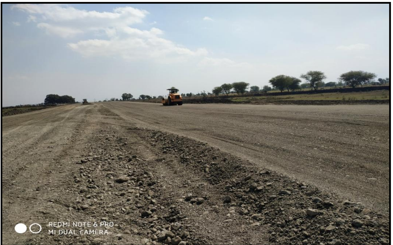
Subgrade Top at Ch.31+000
