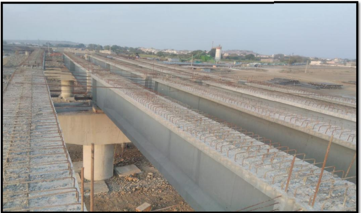
Elevated Highway@ Ch. 47+830
