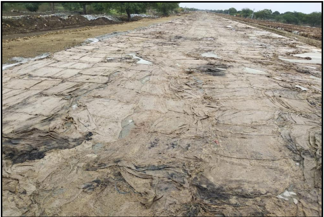
PQC Laying at Ch.16+327 to 16+600 (BHS)
