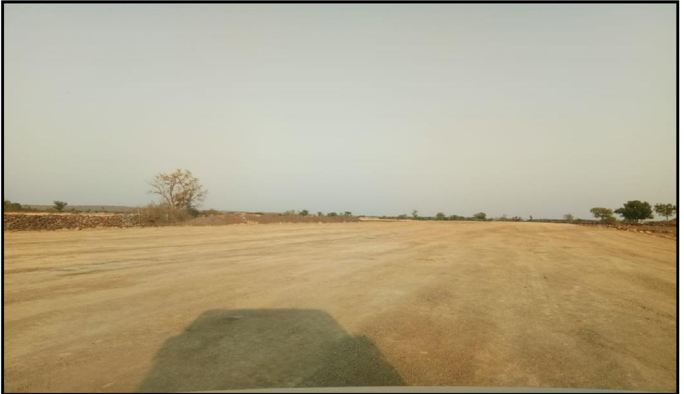
Embankment Top at Ch. 31+500 to 31+700 (LHS)
