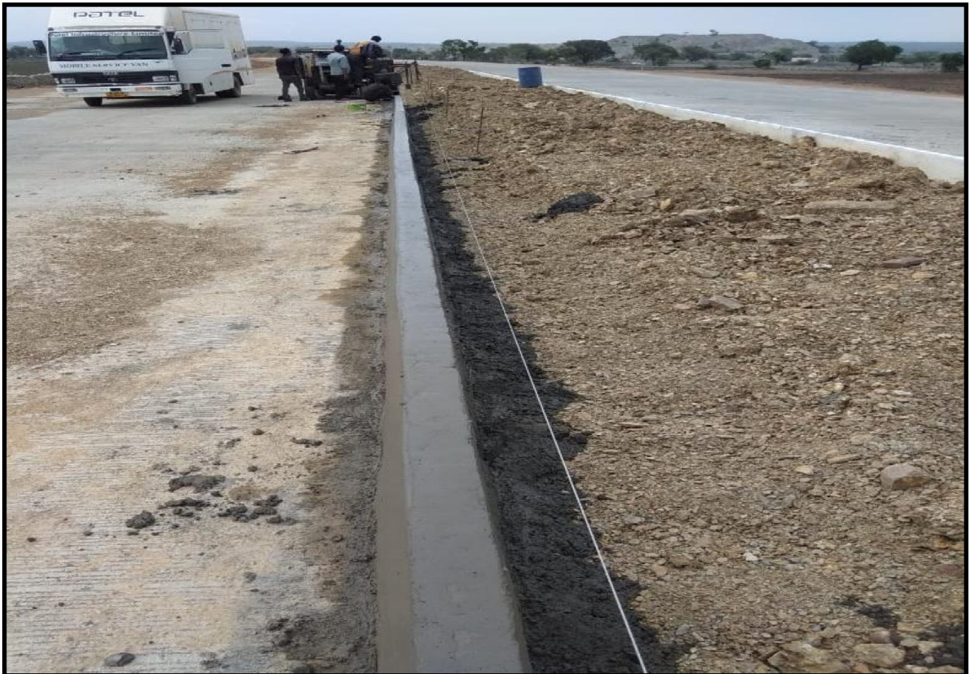
Kerb Laying at Ch. 13+300
