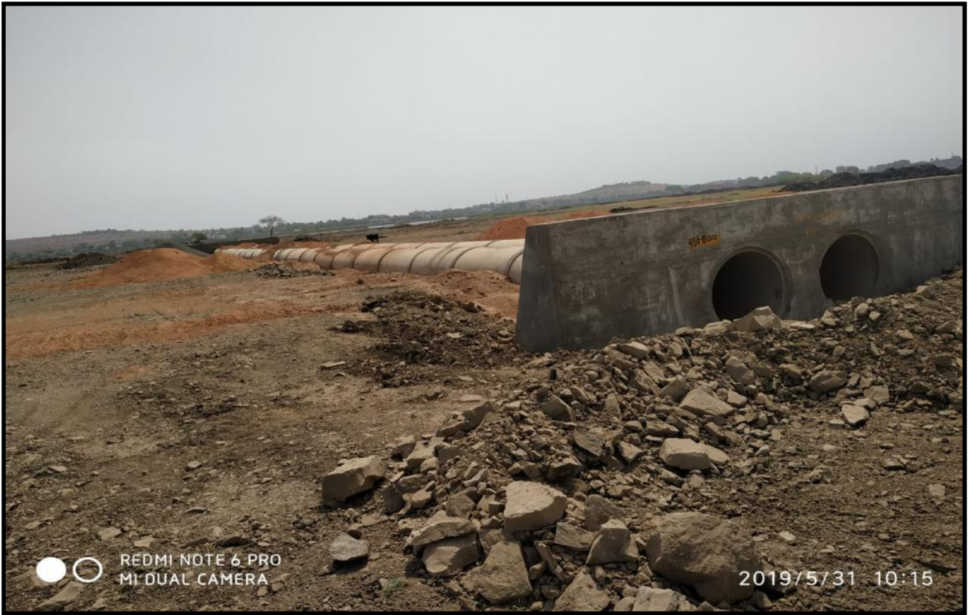
Hume Pipe Culvert @ Ch.45+800
