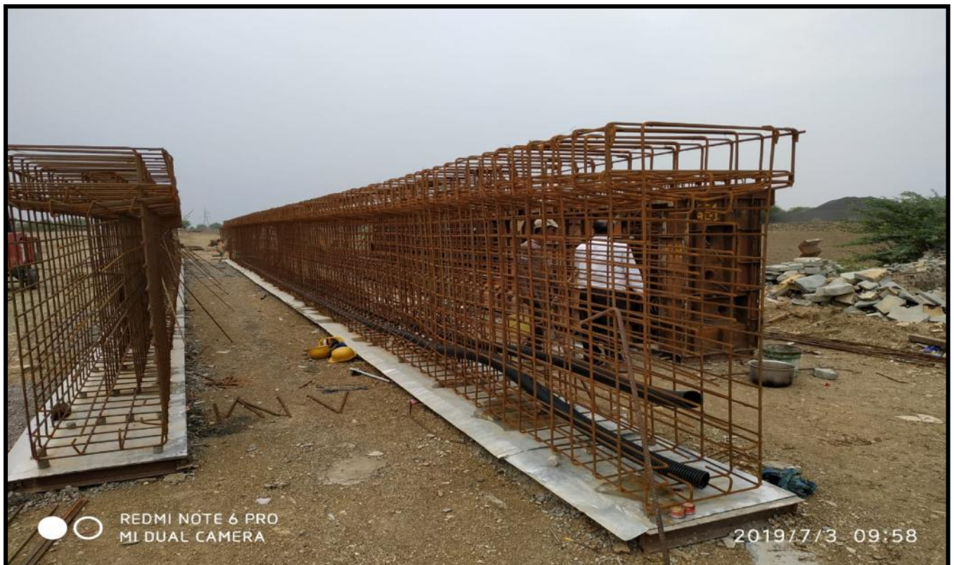
VUP Girder Reinforcement Checking at Ch.30+075
