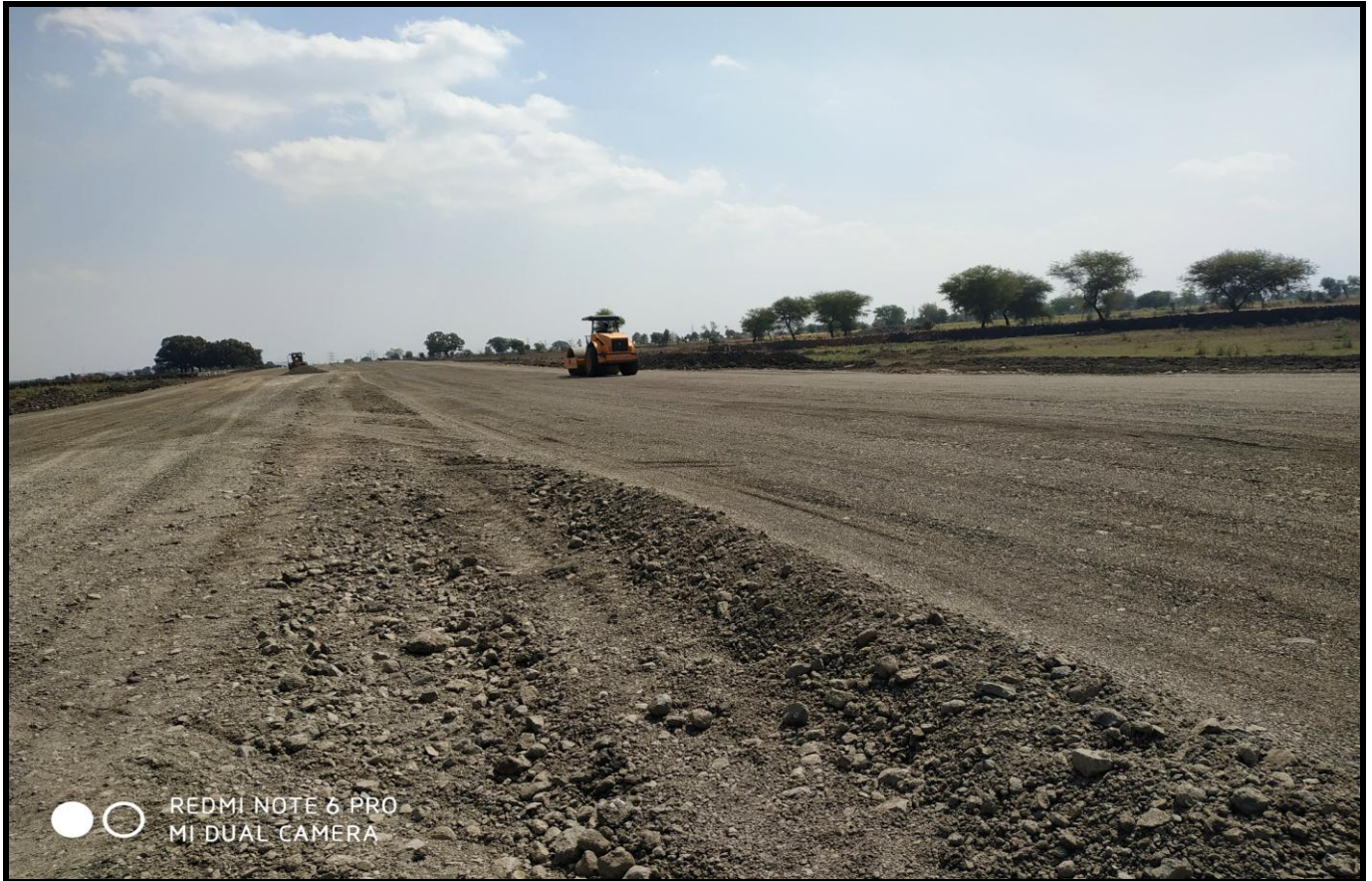
Subgrade Top at Ch.31+000
