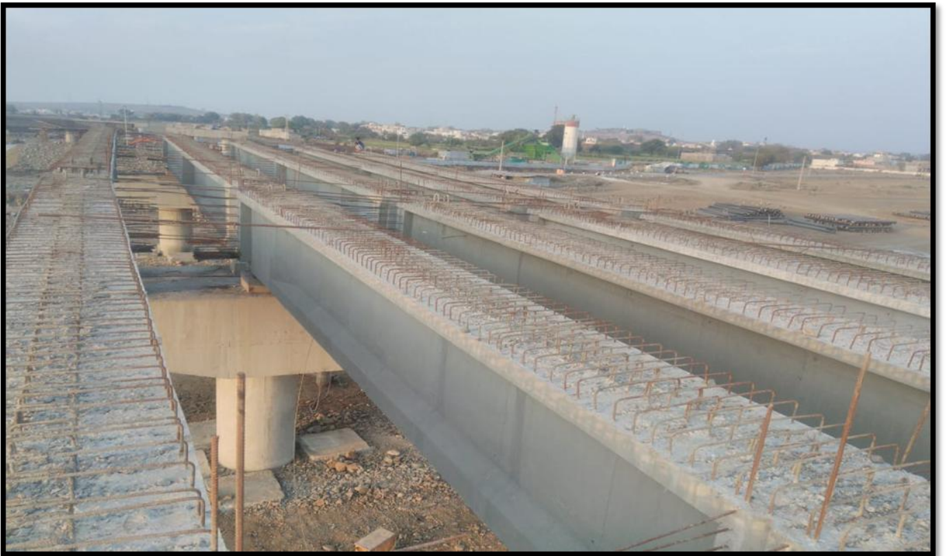
Elevated Highway@ Ch. 47+830
