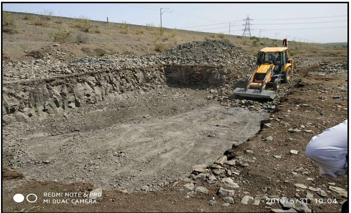
R.O.B Excavation @ Ch.44+158
