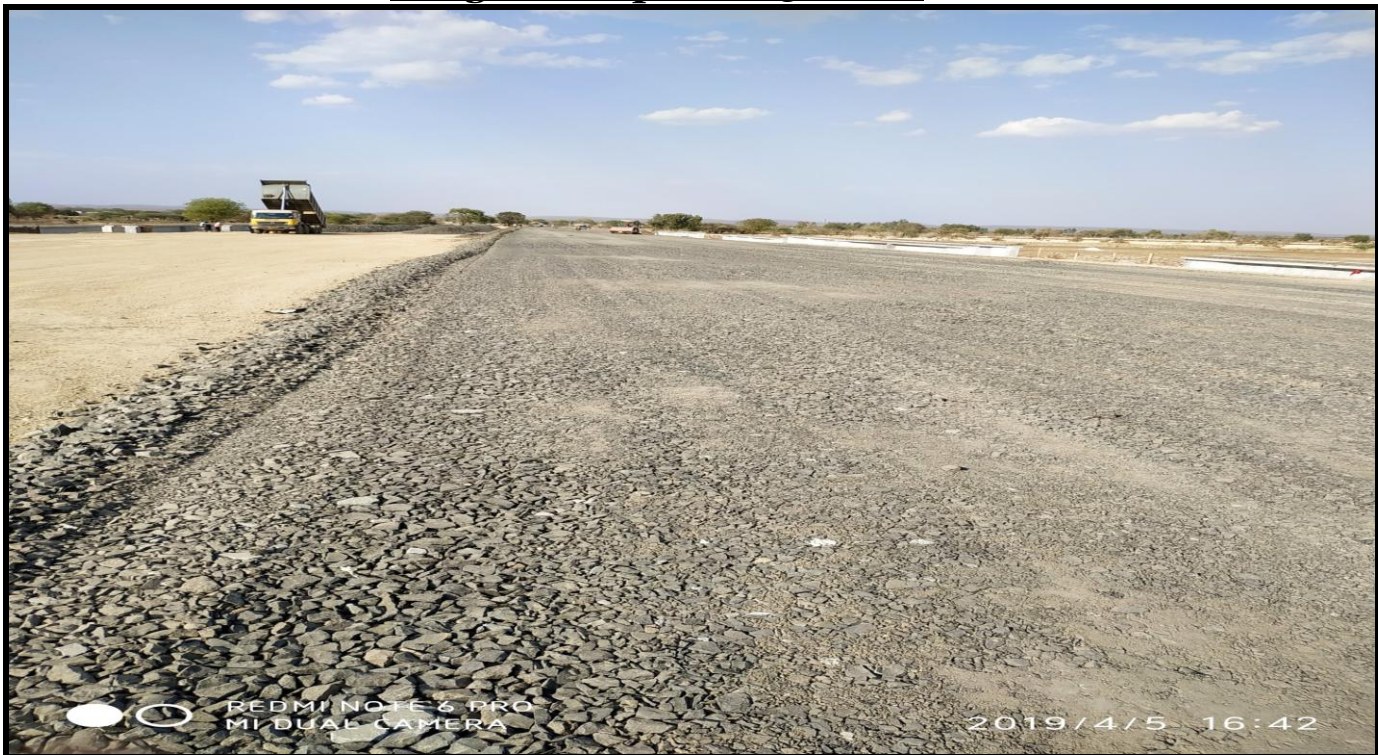
GSB @ Ch. 46+500 (RHS)
