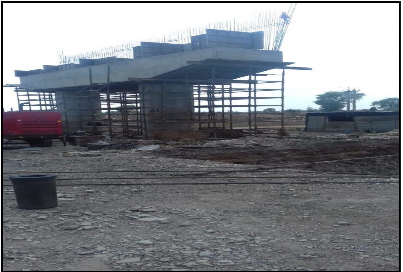
Abutment Cap A-1 & A-2 VUP @ Ch.25+100 (R/S)
