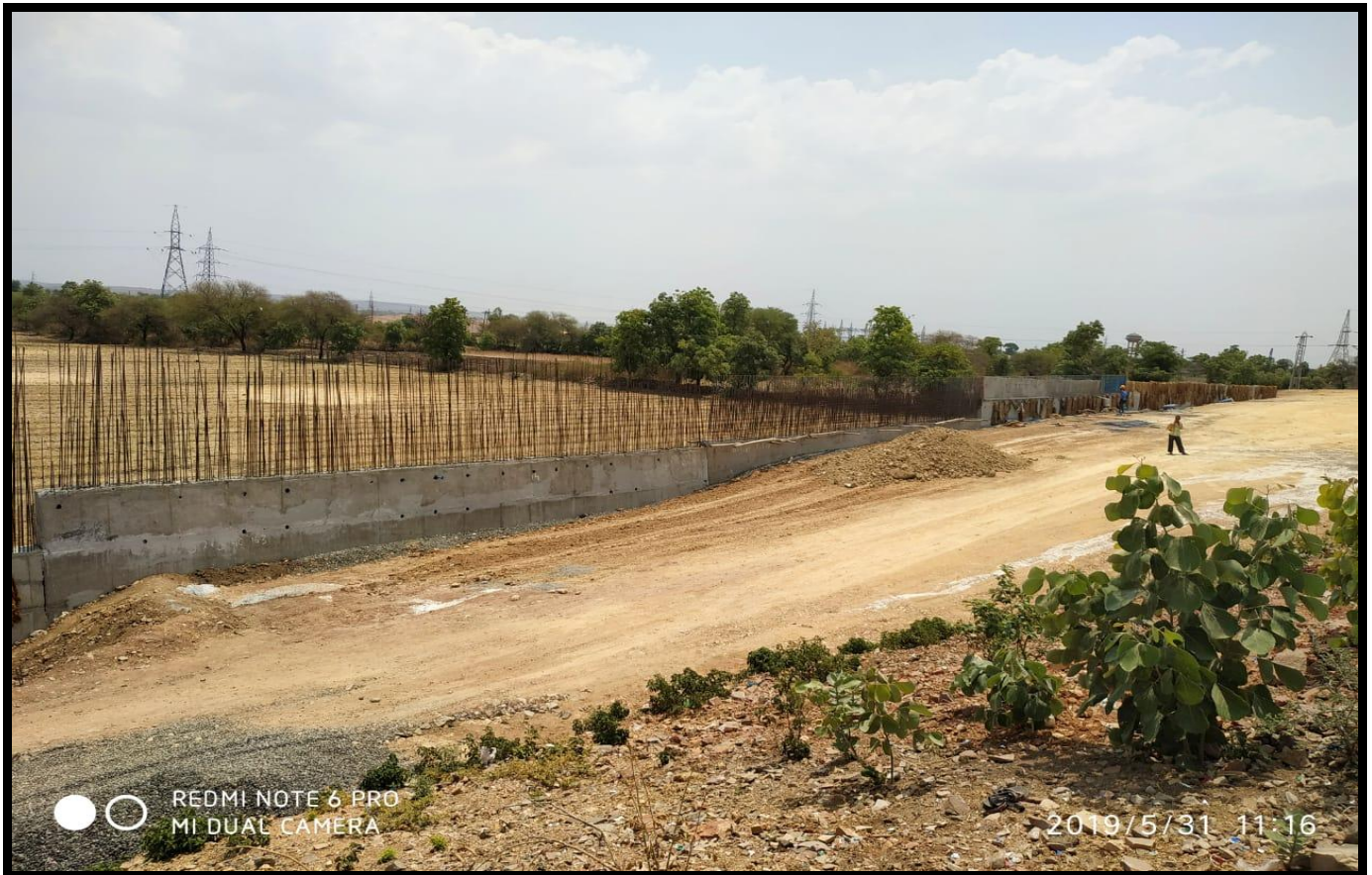
Retaining Wall @Ch. 57+200
