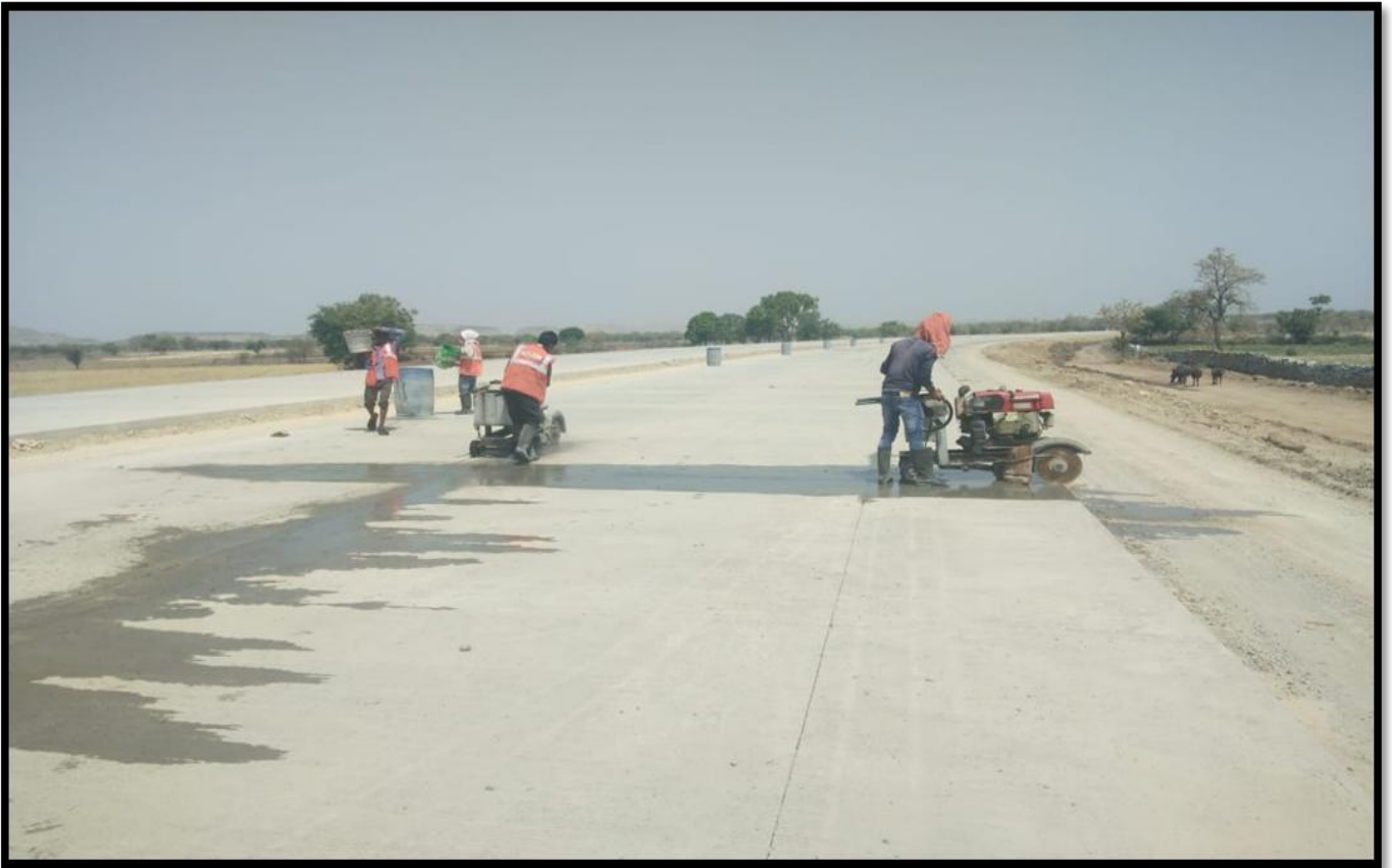
PQC Laying & Final Cutting
