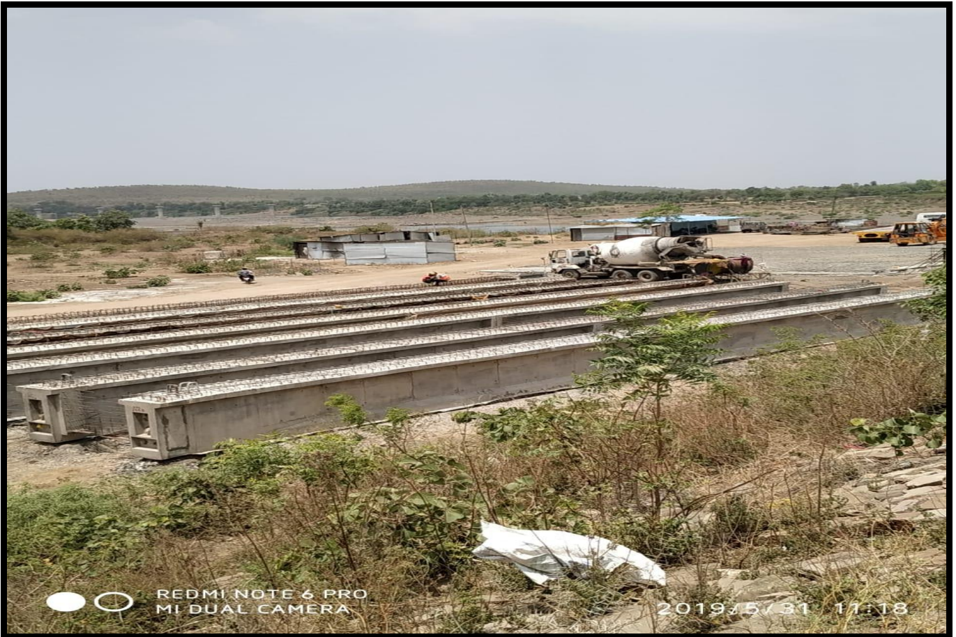
MJB Girder Casting at Ch.57+127
