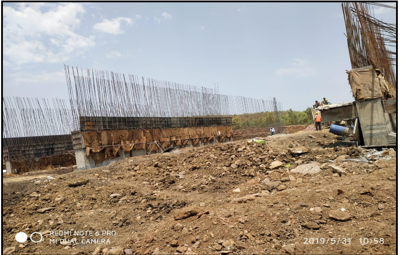
Minor Bridge Work @ Ch. 54+040
