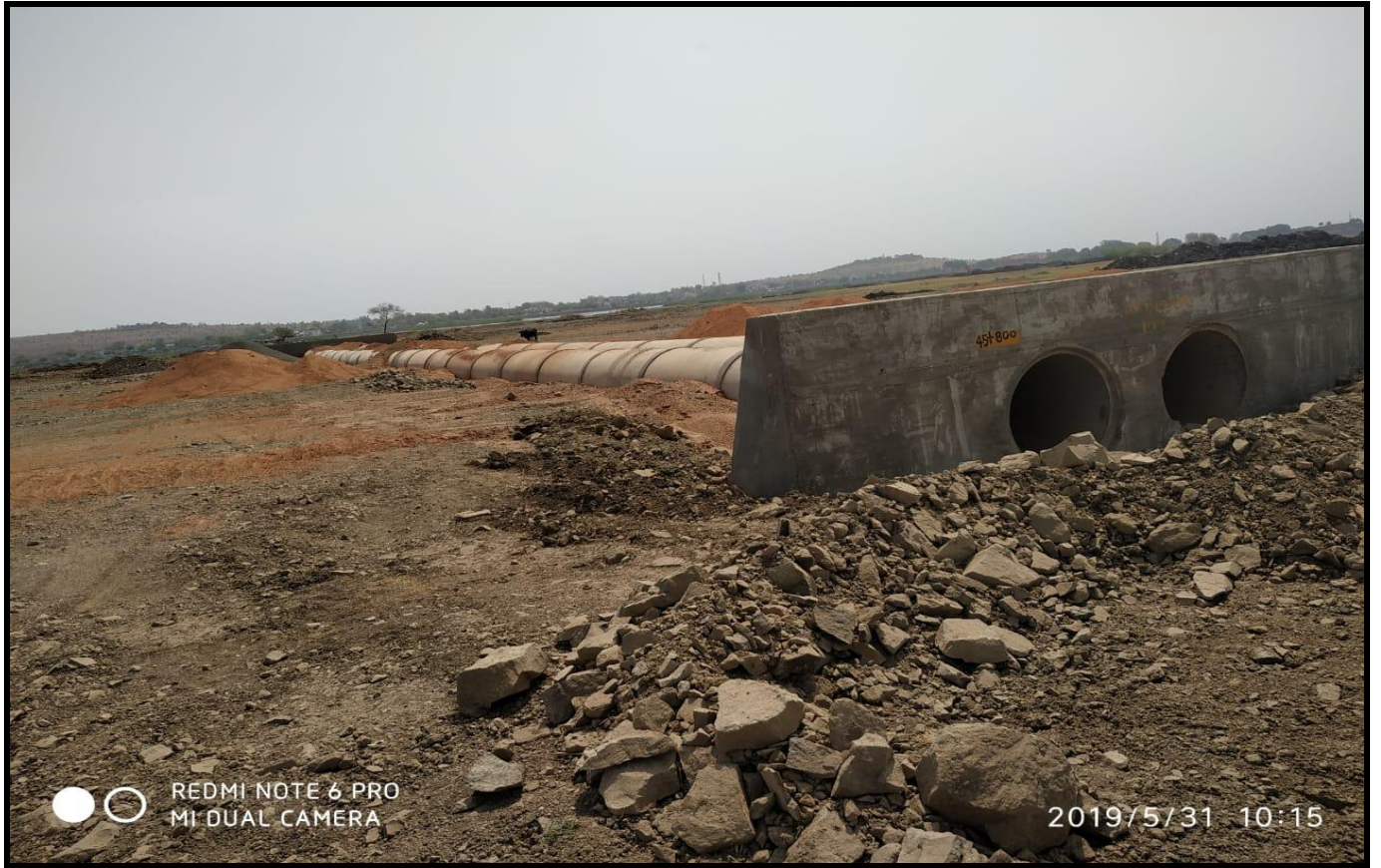
Hume Pipe Culvert @ Ch.45+800
