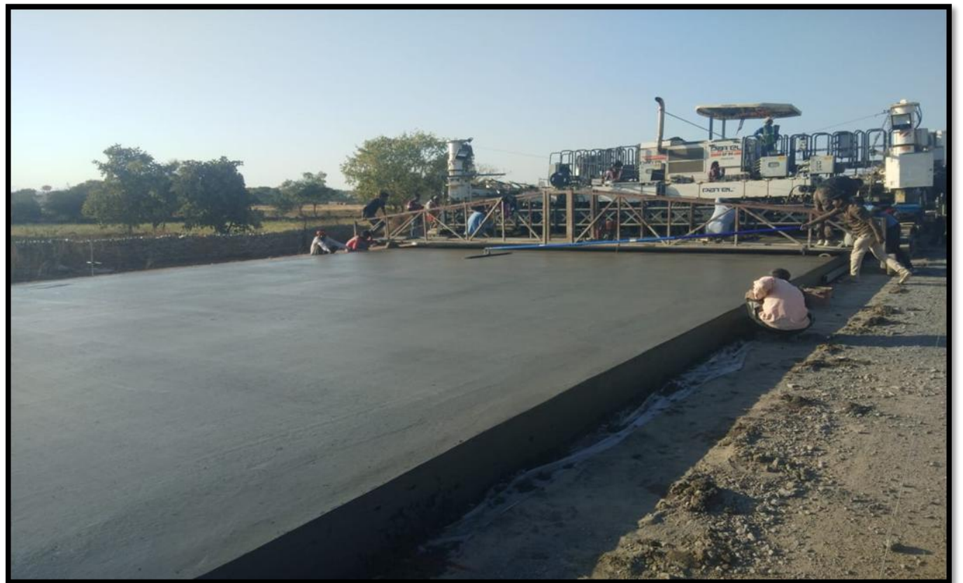
PQC Laying at Ch.25+800 to 26+480
