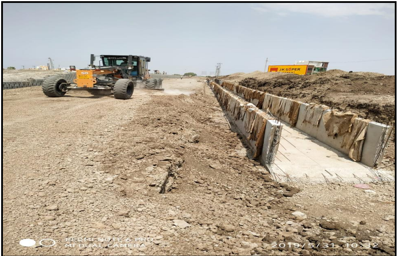
Drain Work @ Ch.49+300
