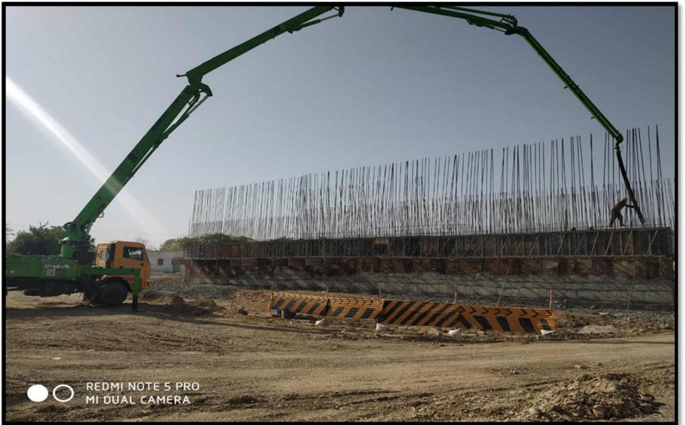
LVUP Concrete Work @ Ch. 12+450
