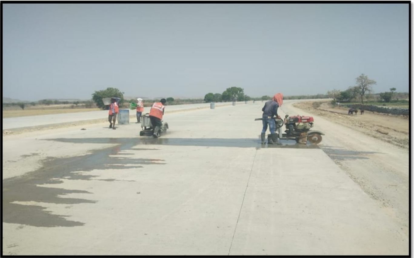
PQC Laying & Final Cutting
