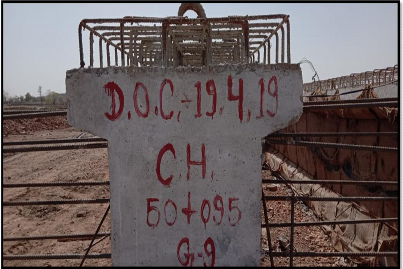
Girder Casting @ Ch. 50+095
