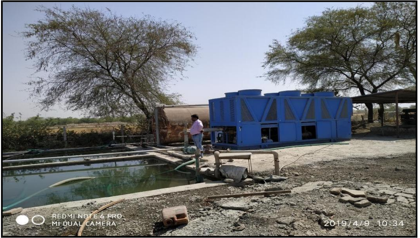
Chilling Plant Erected at Camp-1
