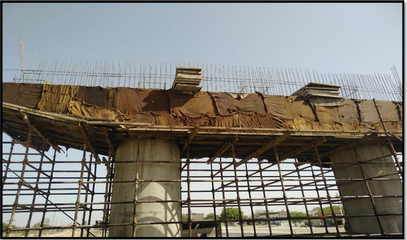
Abutment Cap A-1 VUP @ Ch.25+100
