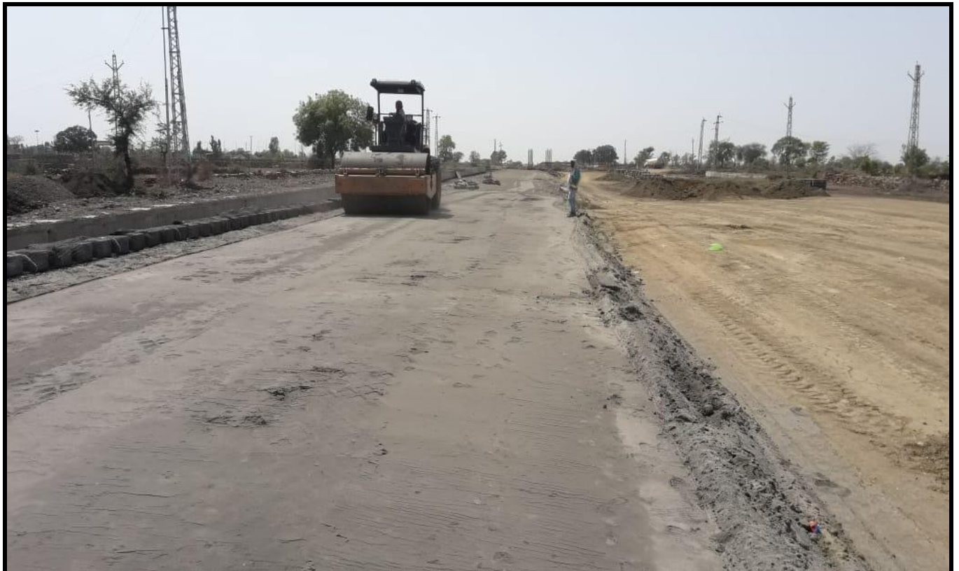
Pond ash Rolling at Ch.41+307 to 41+440
