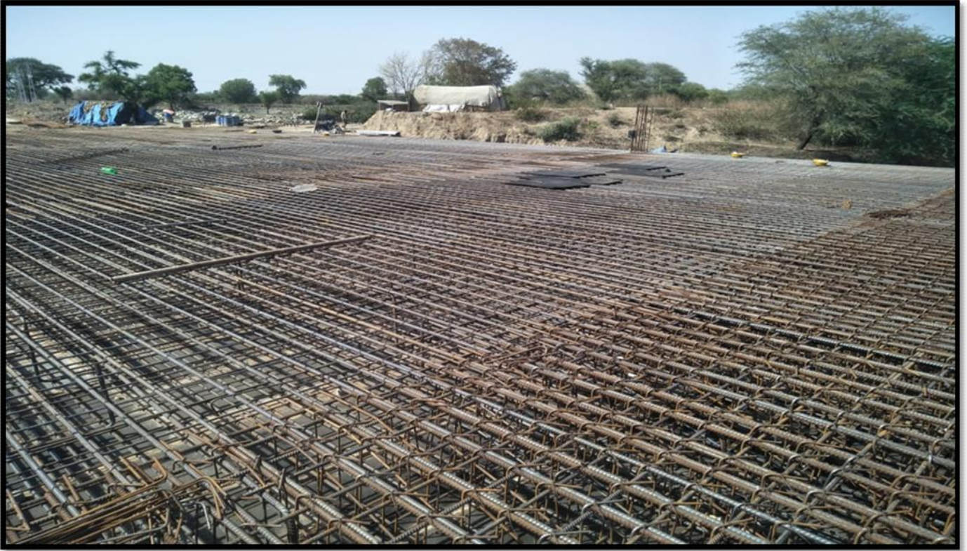
MNB Slab Reinforcement @Ch. 17+890
