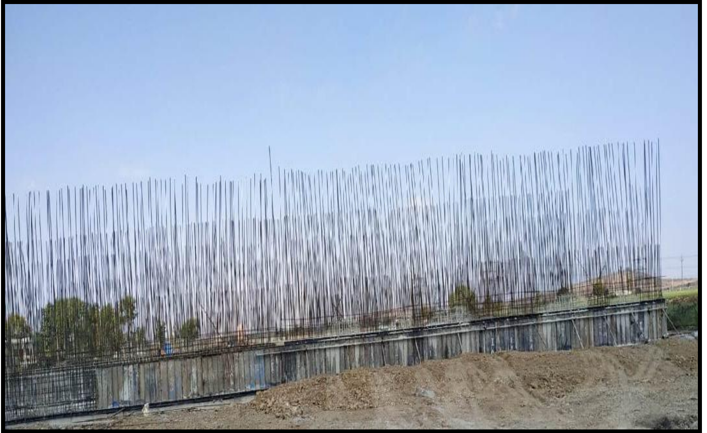
Minor Bridge @ Ch. 44+800
