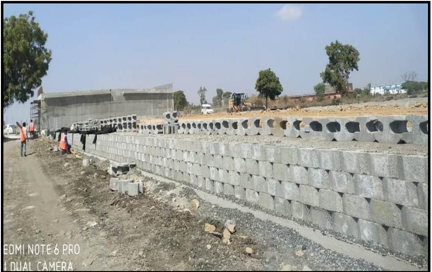
RE Wall Block Erection @ Ch 41+465
