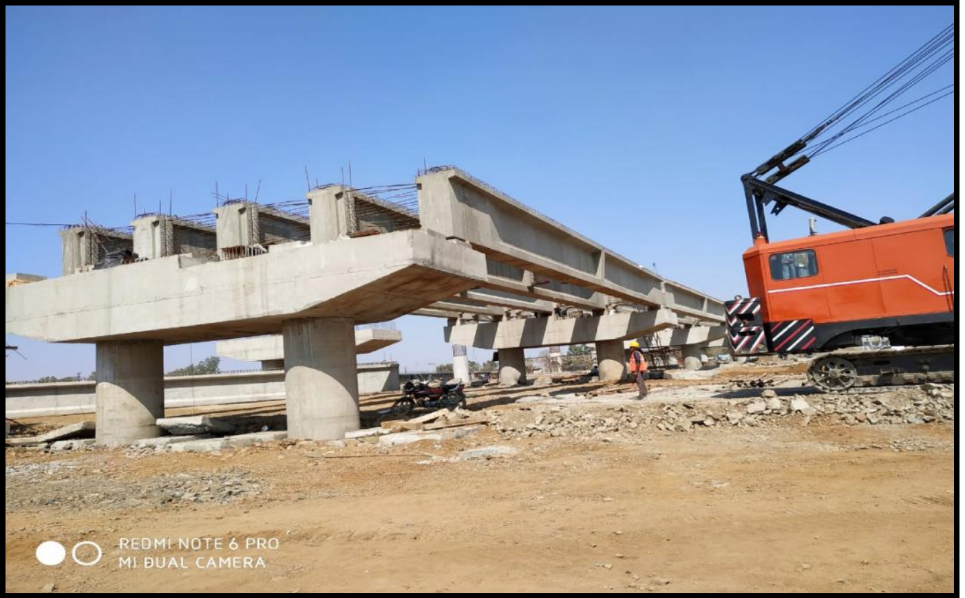
Girder Launching at Elevated Highway @ Ch 47+830
