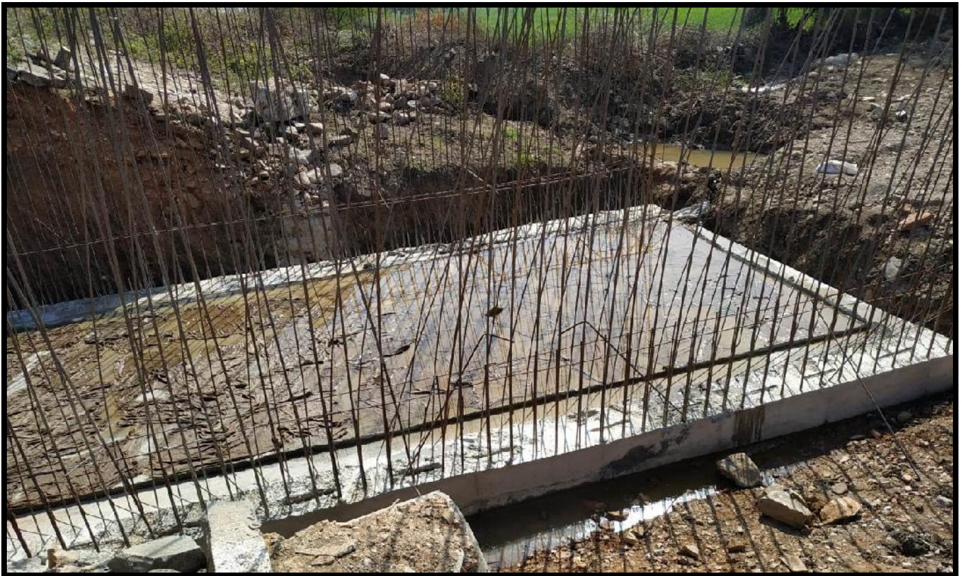
Raft of Box Culvert @ Ch. 55+820
