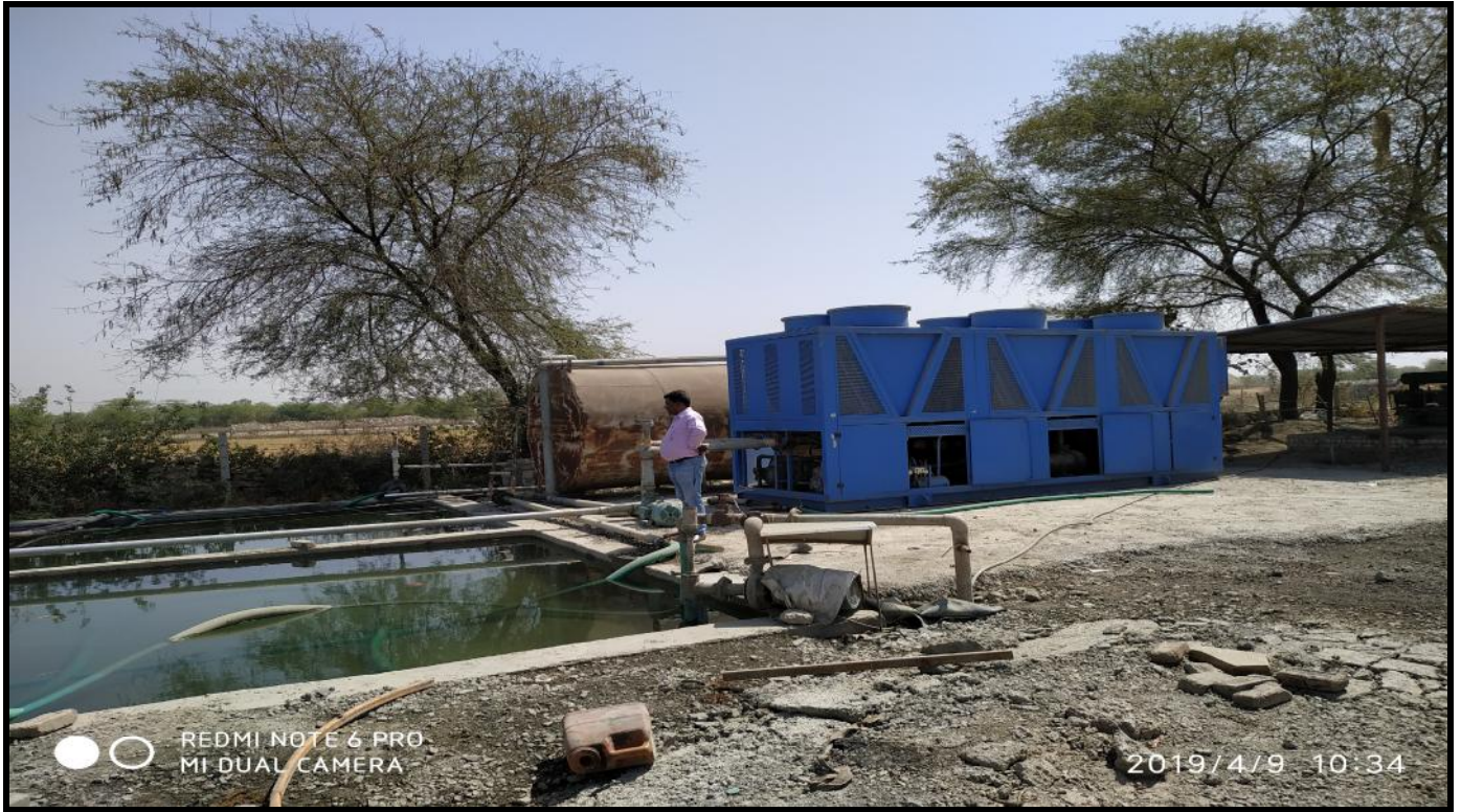
Chilling Plant Erected at Camp-1
