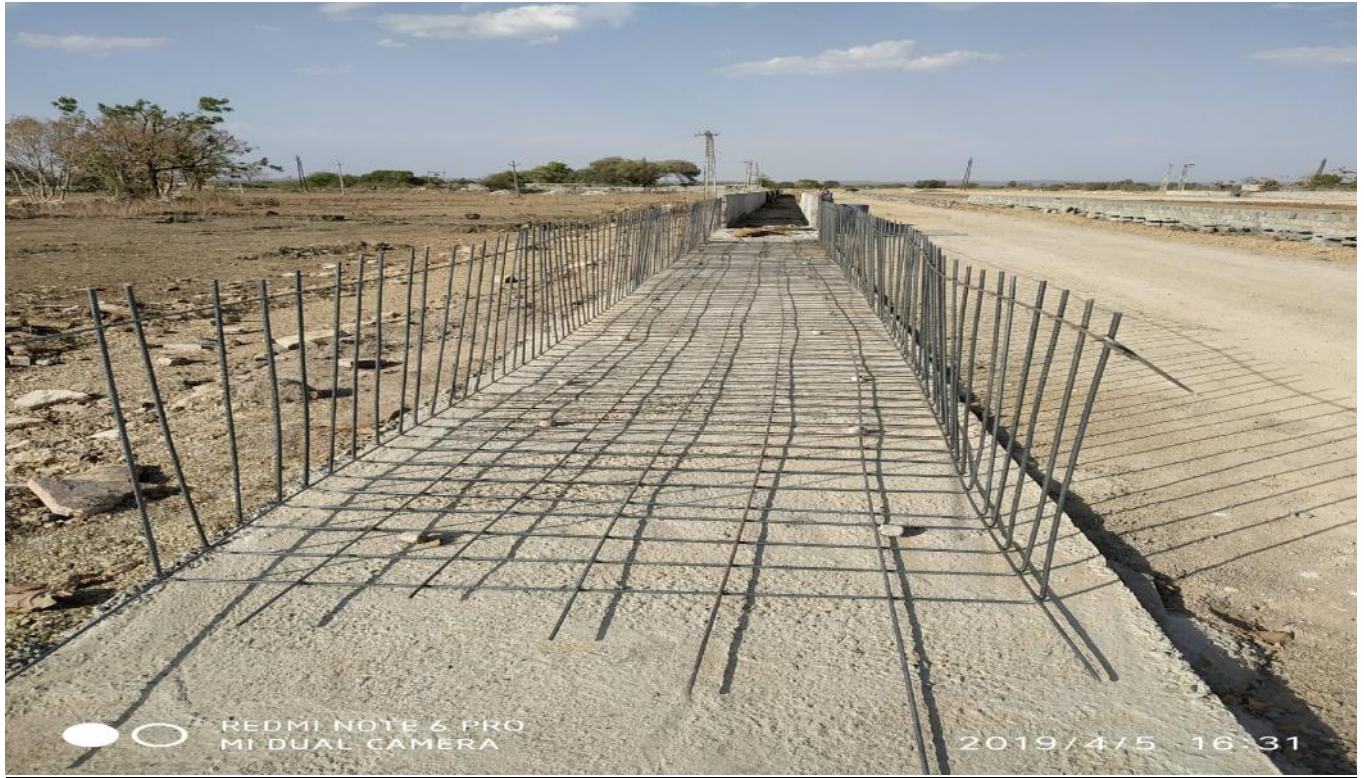
Drain Wall at Ch.26+600
