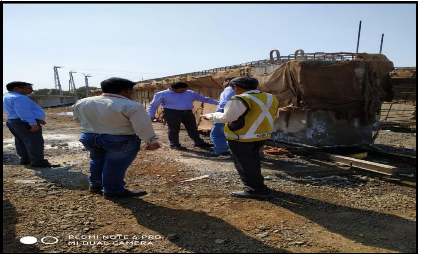
Checking of Casted Girders by Landers Engineers @ Ch 47+830
